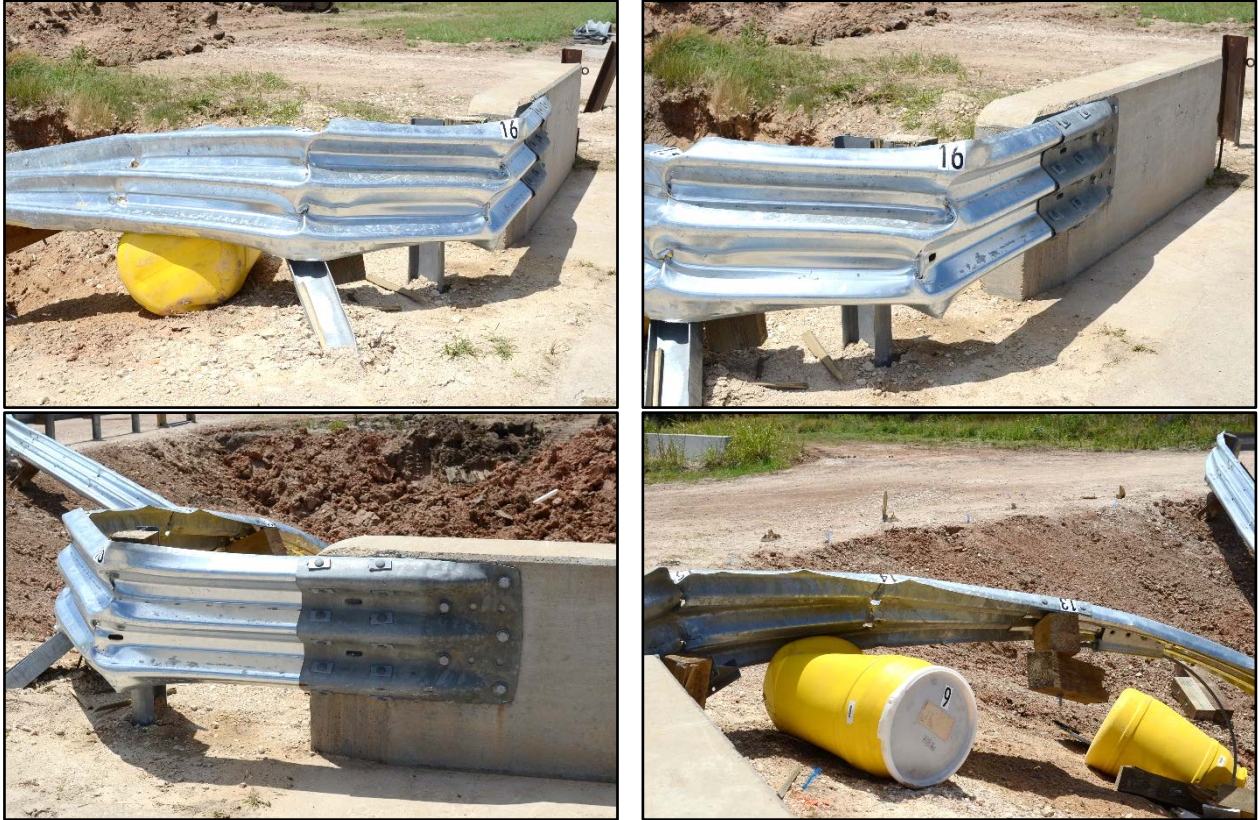
Figure 7.6. Damage to Rail Section Parallel to Roadway after Test No. 469137-3-1.
