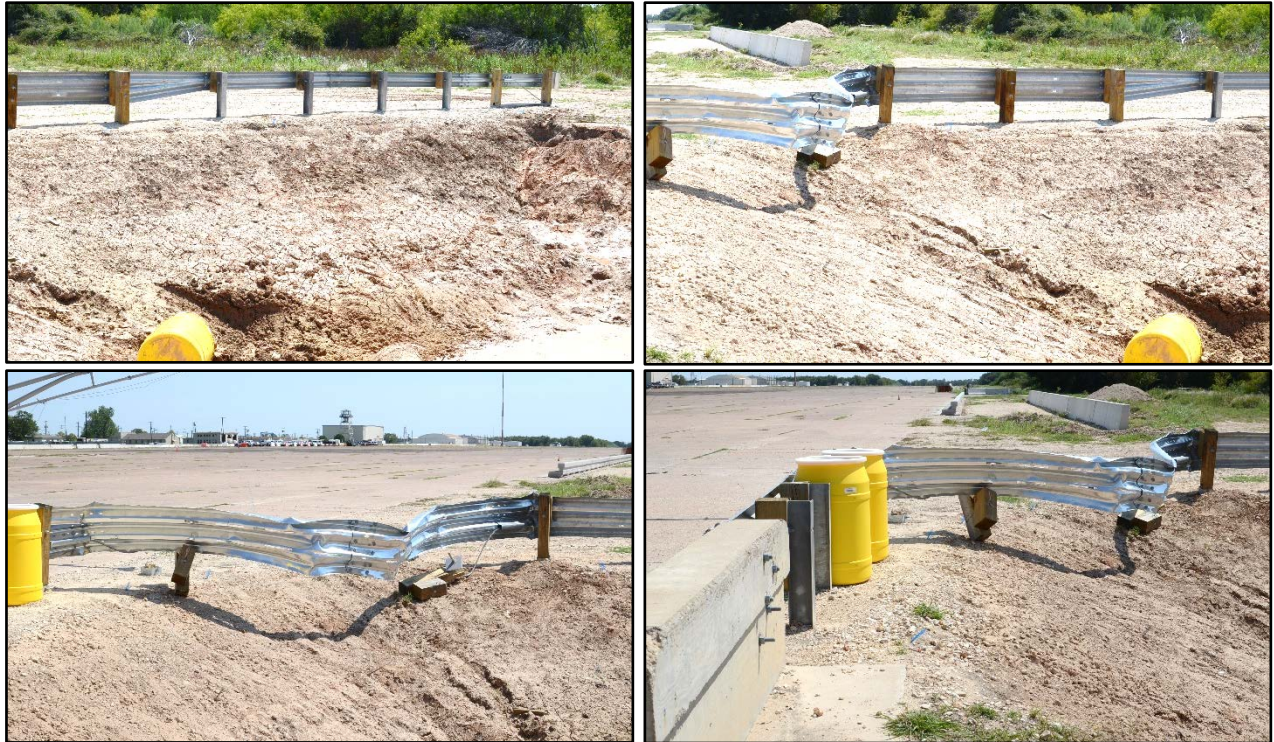
Figure 8.5. Field Side of Test Article after Test No. 469137-3-2.
