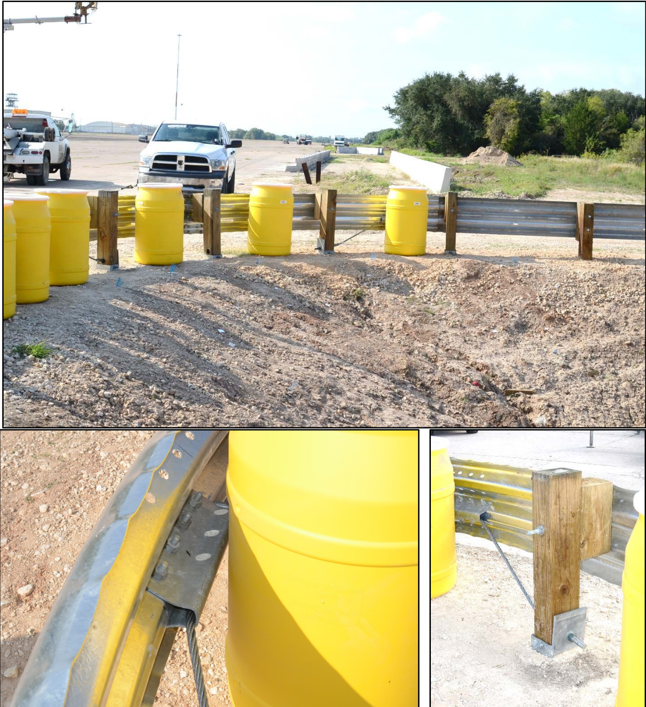
Figure 4.4. Cable prior to Test Nos. 469138-3-3 and 469138-3-4.
