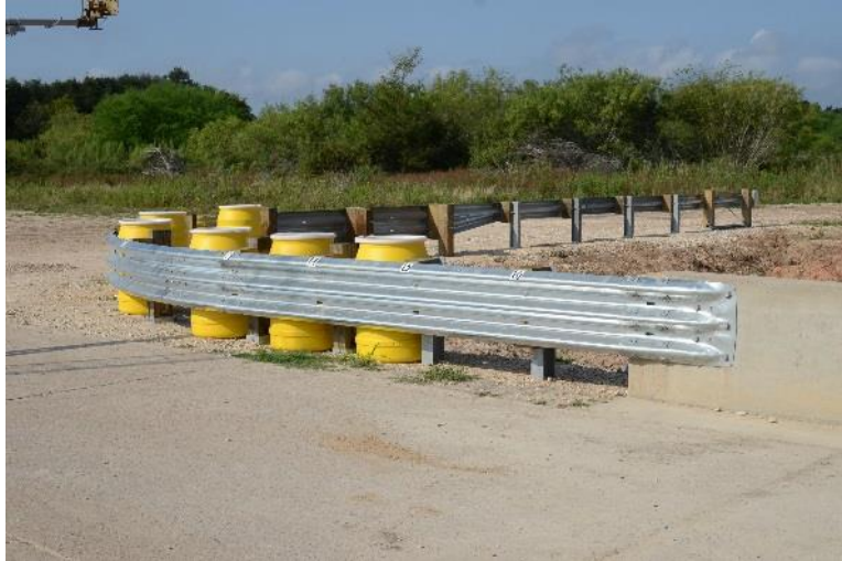
Figure 1. Test Installation of the New TL-2 Short Radius Design.
