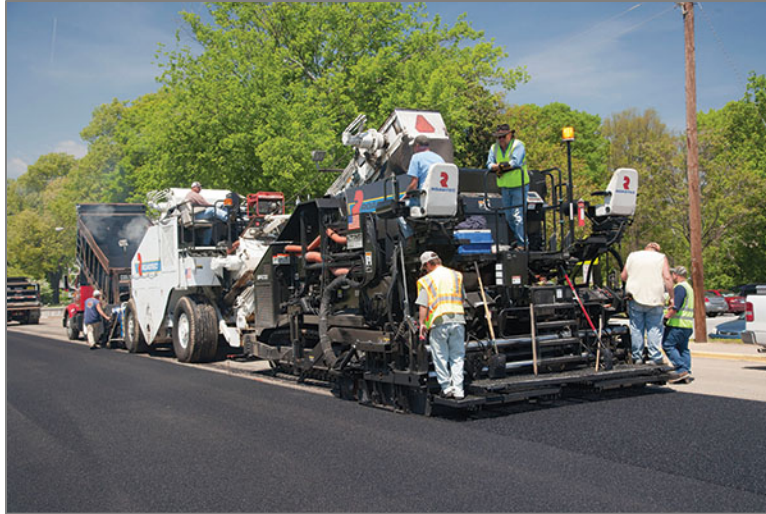
Figure 2-4. Underseal Membrane Applied with a Spray Paver.
