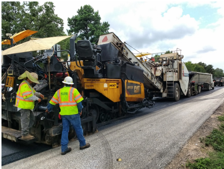
Figure 5-4. US 79 Paving Train.
