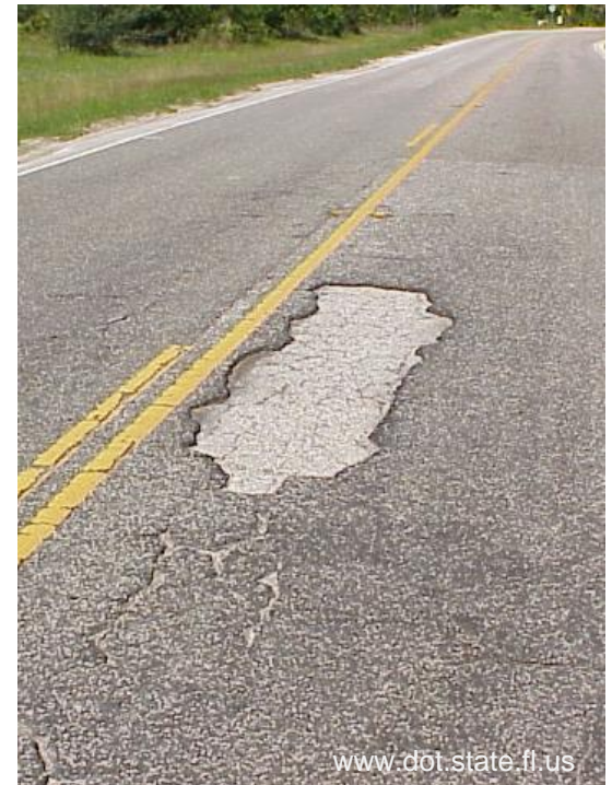
Delamination
