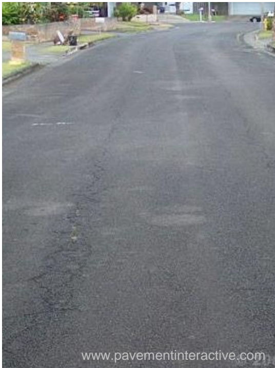
Fatigue cracking
