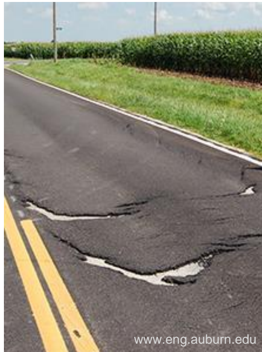
Slippage cracking
