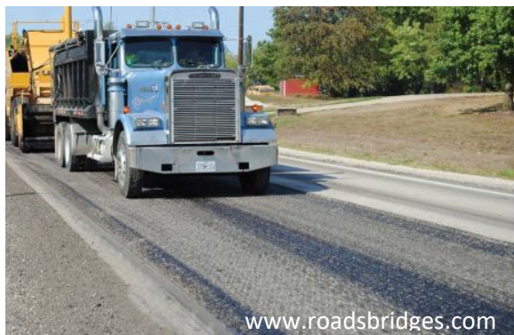
FIGURE 8 – Tack Tracking.
