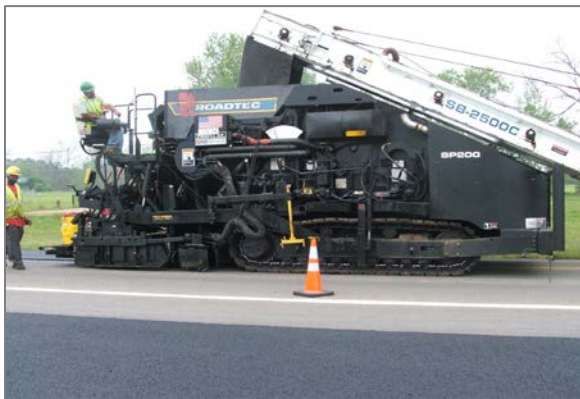
FIGURE 4 – Spray Paver Membrane Underseal.
