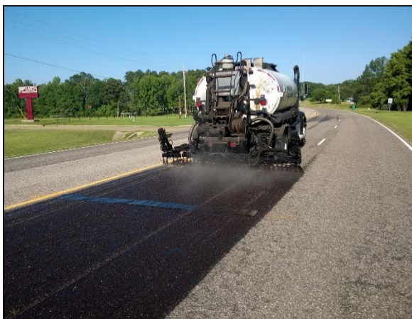
FIGURE 1 – Traditional Tack Coat.
