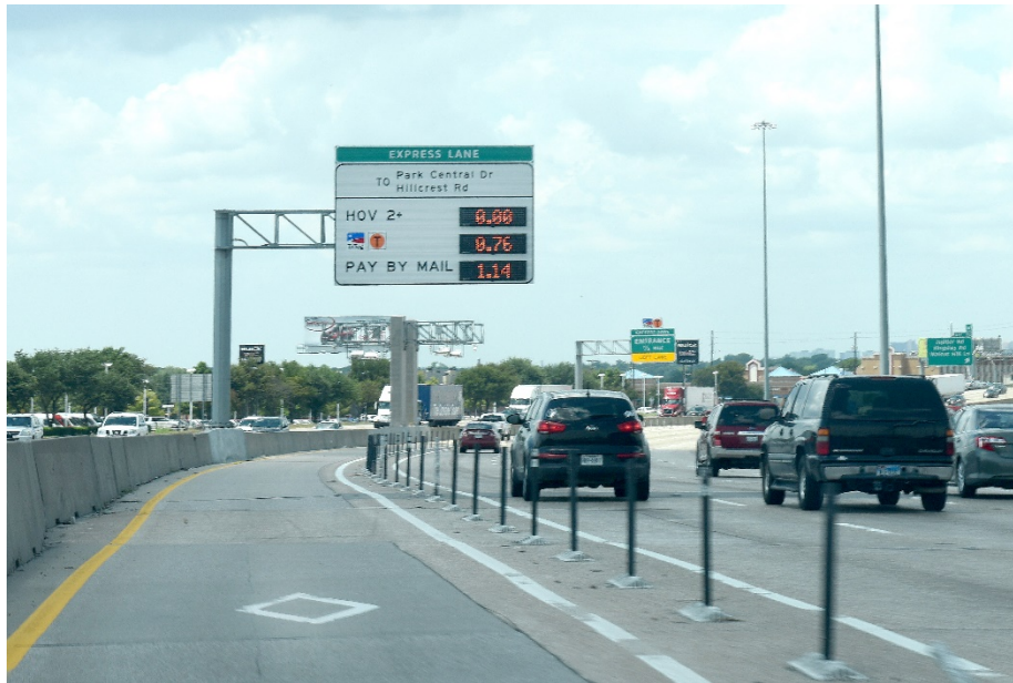
Figure 1. Westbound I-635 East TEXpress Lane® in Dallas, Texas.
