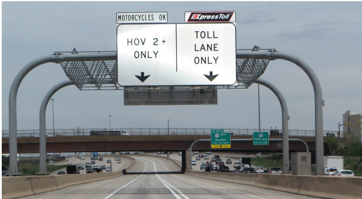
Figure 3. HOT Declaration Lane at Toll Gantry on I-25 Managed Lanes in Denver, Colorado.
