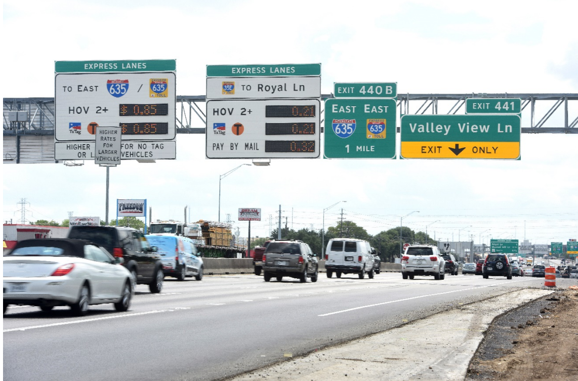
Figure 9. Southbound I-35 Sign Bridge for I-635 LBJ and 35E TEXpress Lanes® in Dallas.
