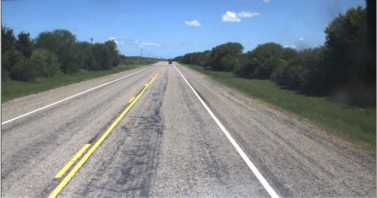
Figure 60. Section 33 along FM 2678 in the Corpus Christi District.
