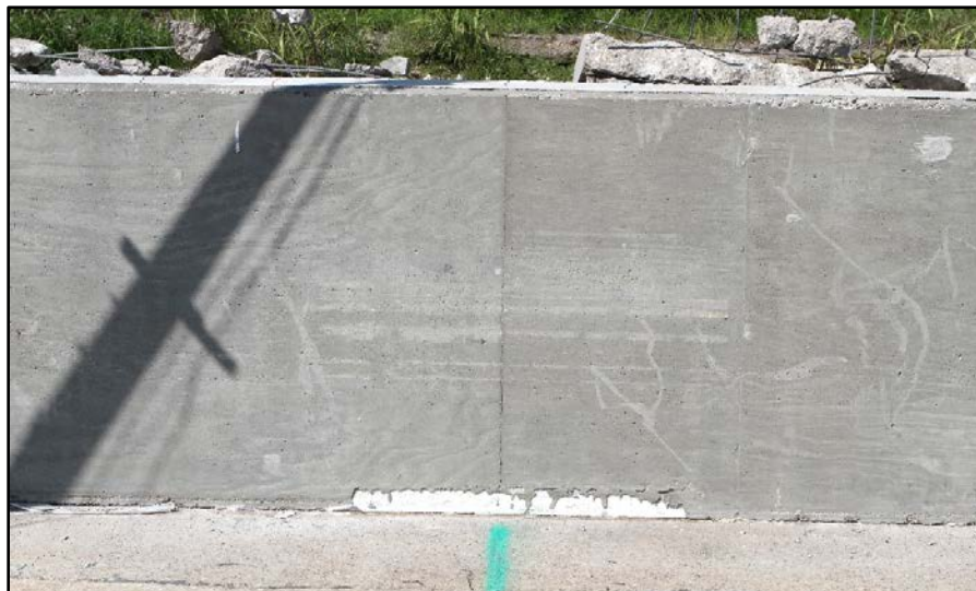
Figure 5.11. Impact Side of Barrier after Test No. 468957-B5.
