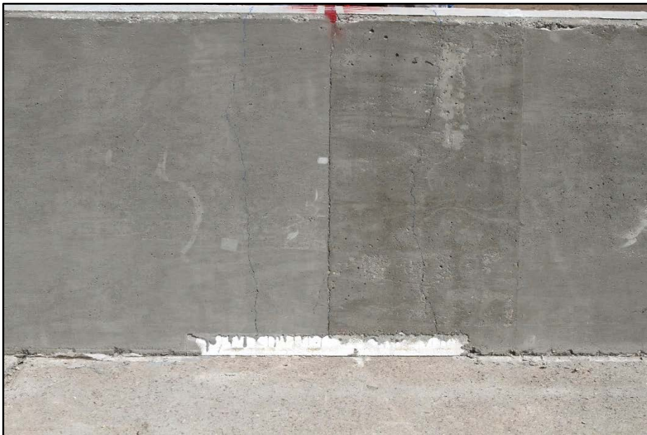
Figure 5.17. Field Side of Barrier after Test No. 468957-B6.
