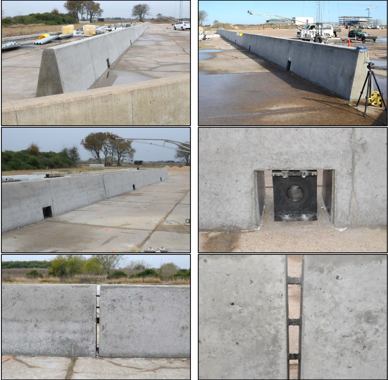
Figure 6.2. TxDOT Rubber Mounted Single Slope Barrier prior to MASH Tests 4-10 and 4-11.
