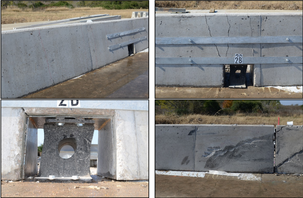
Figure 11.4. Damage to Barrier #2 after Test No. 468958-3.
