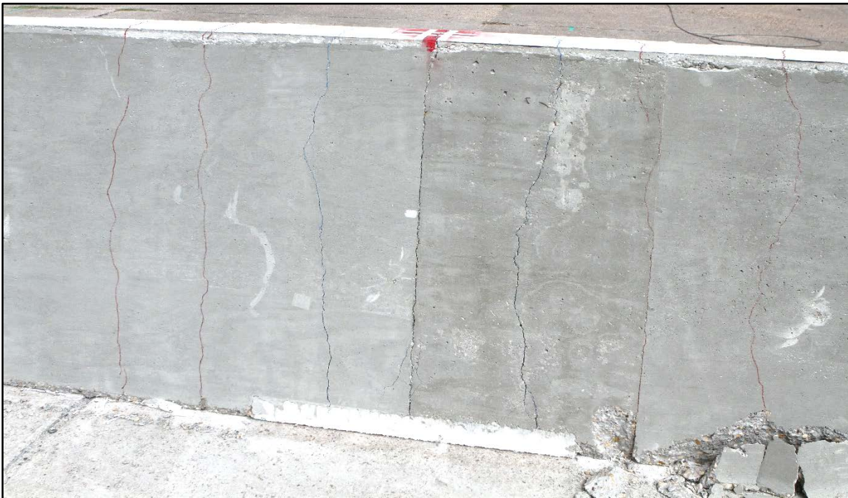
Figure 5.22. Field Side of Barrier after Test No. 468957-B7.
