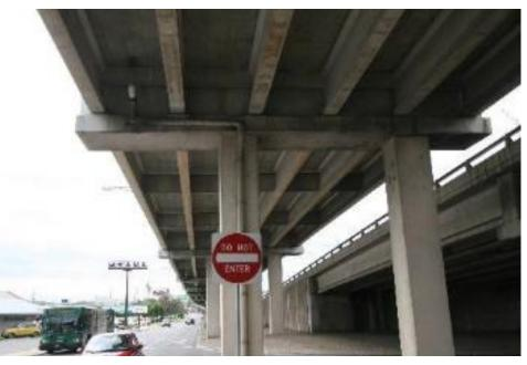
Figure 3.11. Drainage Pipes Attached to Ledge of Multi-Column Bent.
