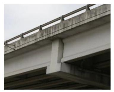
Figure 3.9. Edge of Deck Extends Past End of Inverted-T Bent Caps.
