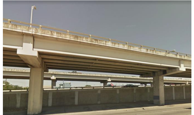
Figure 1. Inverted-T Bent Cap on I-35 in Austin, Texas.
