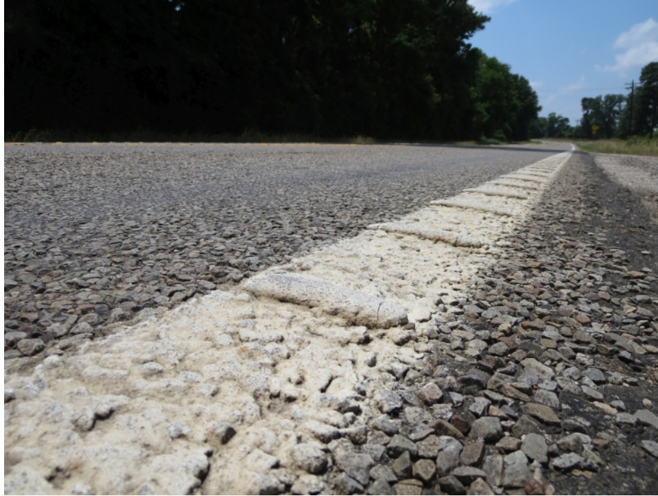
Figure 7. FM 1971 Edge Line Profile Audible Marking.
