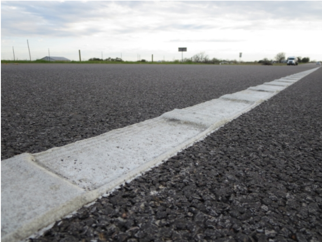
Figure 16. New Profile Pavement Marking near Lincoln.
