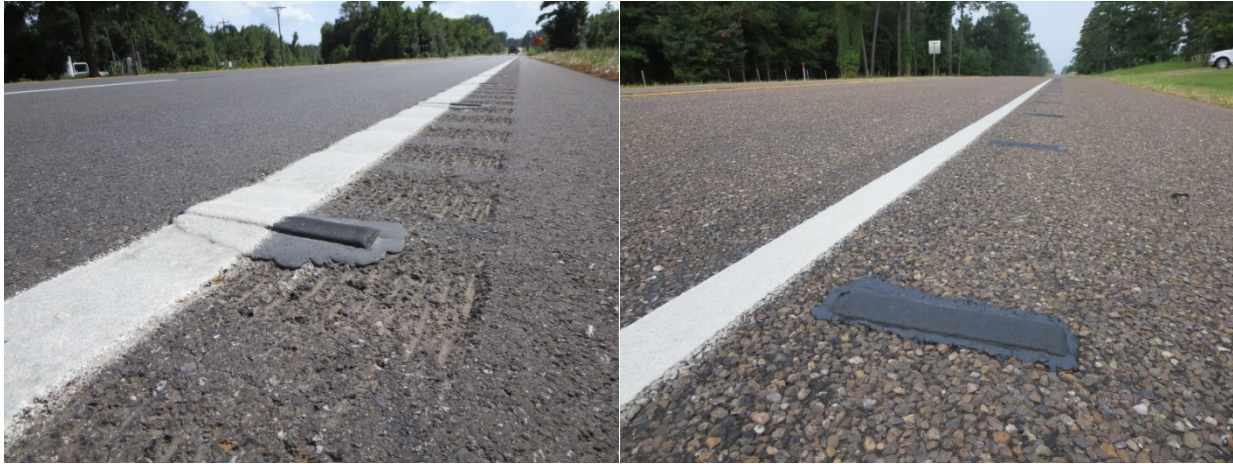
Figure 2. Rumble Bars on Edge Line and Shoulder.
