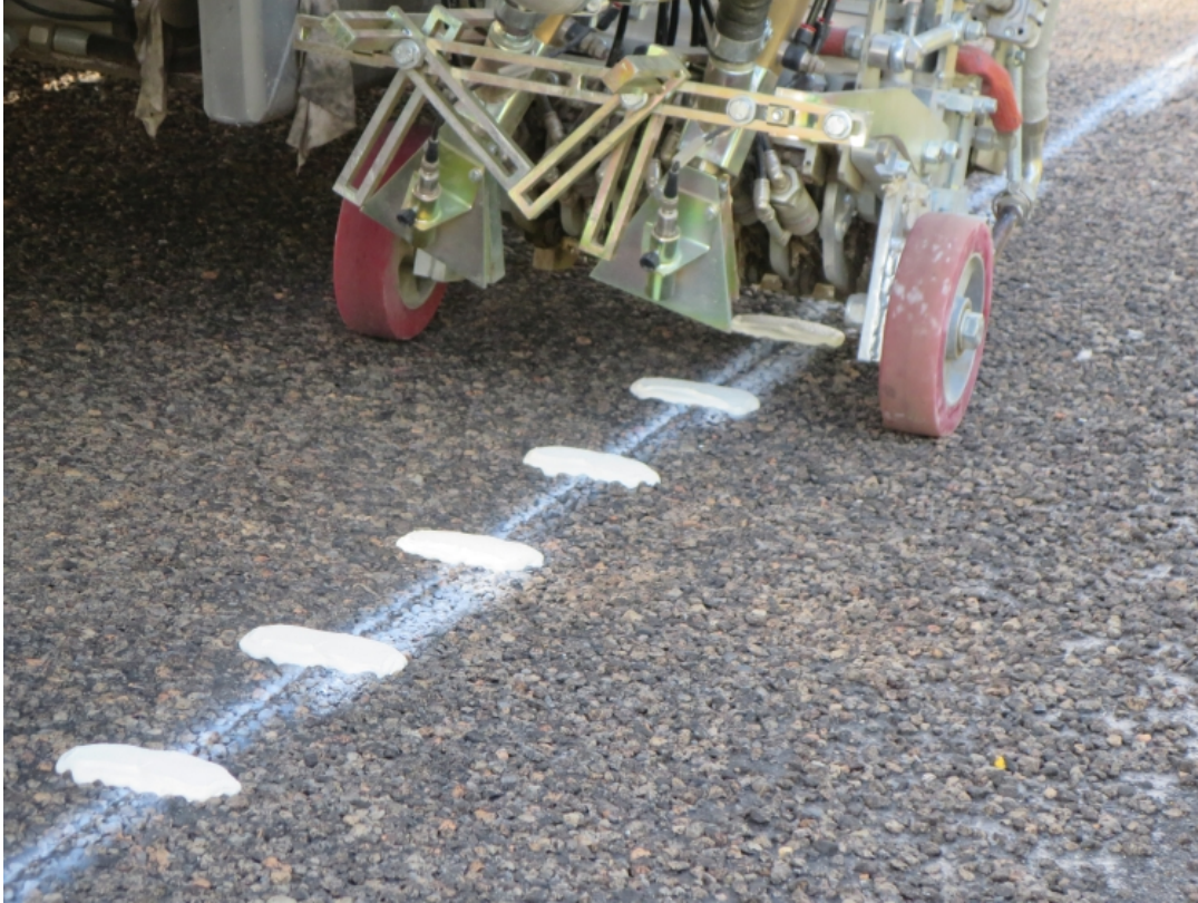
Figure 18. Profile Bump Installation.
