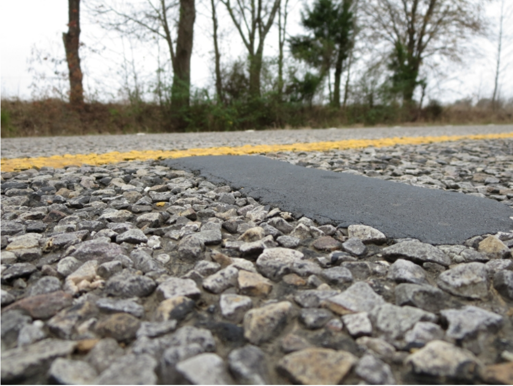
Figure 13. FM 2088 Center Line Rumble Bars (Bars Are Somewhat Flattened Out).
