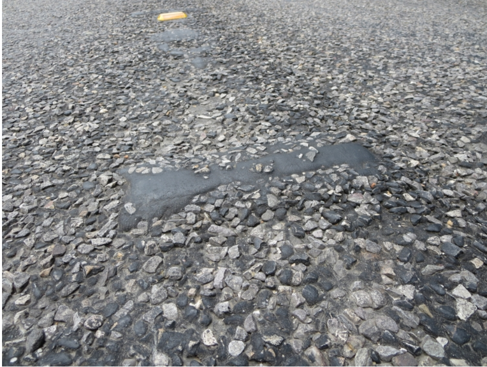
Figure 9. SH 155a Center Line Rumble Bars with One Seal Coat.
