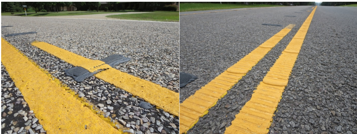
Figure 3. Rumble Bars and Audible Markings on Centerlines.
