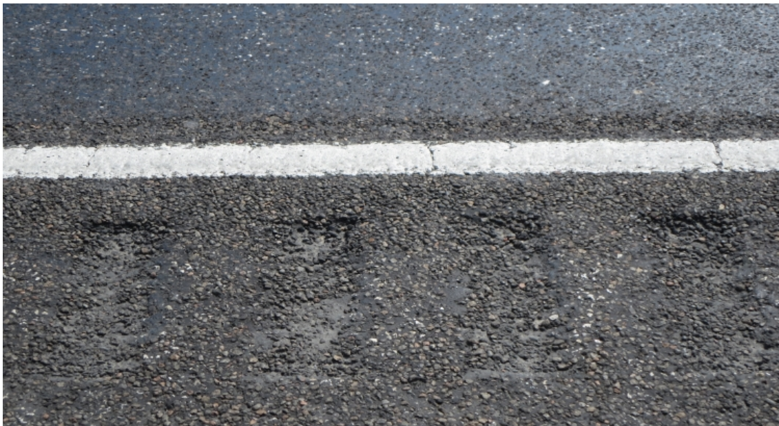
Figure 17. Seal Coat over Milled Rumble Strip near Bryan.
