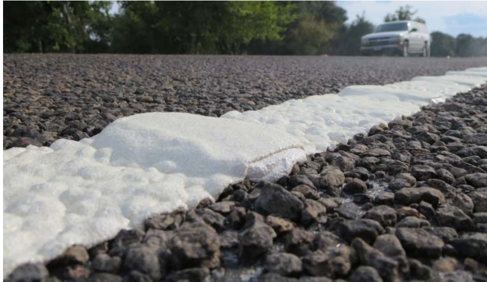
Figure 21. New Profiled Marking with Solid Line over Bump (WB1).
