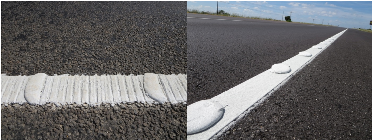
Figure 1. Inverted Profile Marking (Audible) and Profile Edge Line Markings.
