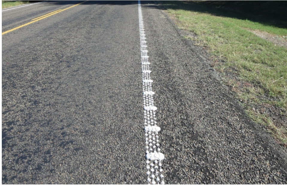
Figure 23. Profiled Bumps with Dot Marking (Standard Spacing, EB1).
