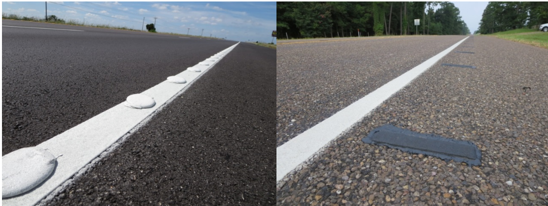
Profile pavement markings (left), rumble bars (right).
