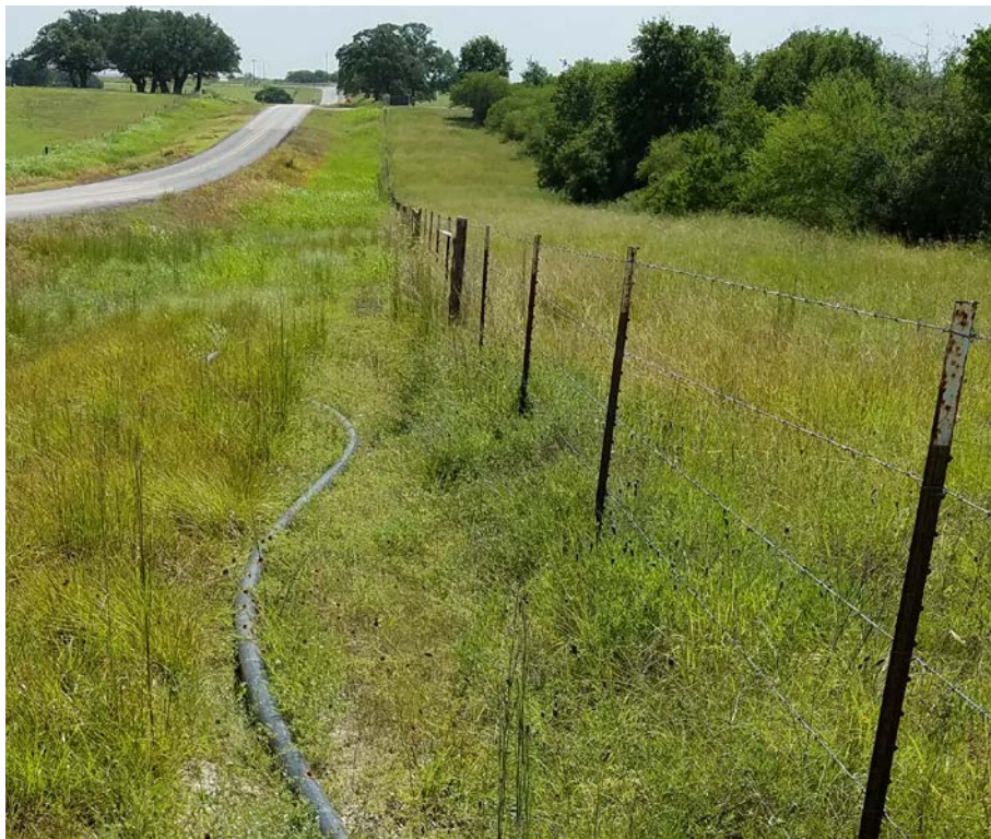
Figure 32. Temporary Pipeline Installation on FM 2816 in De Witt County.
