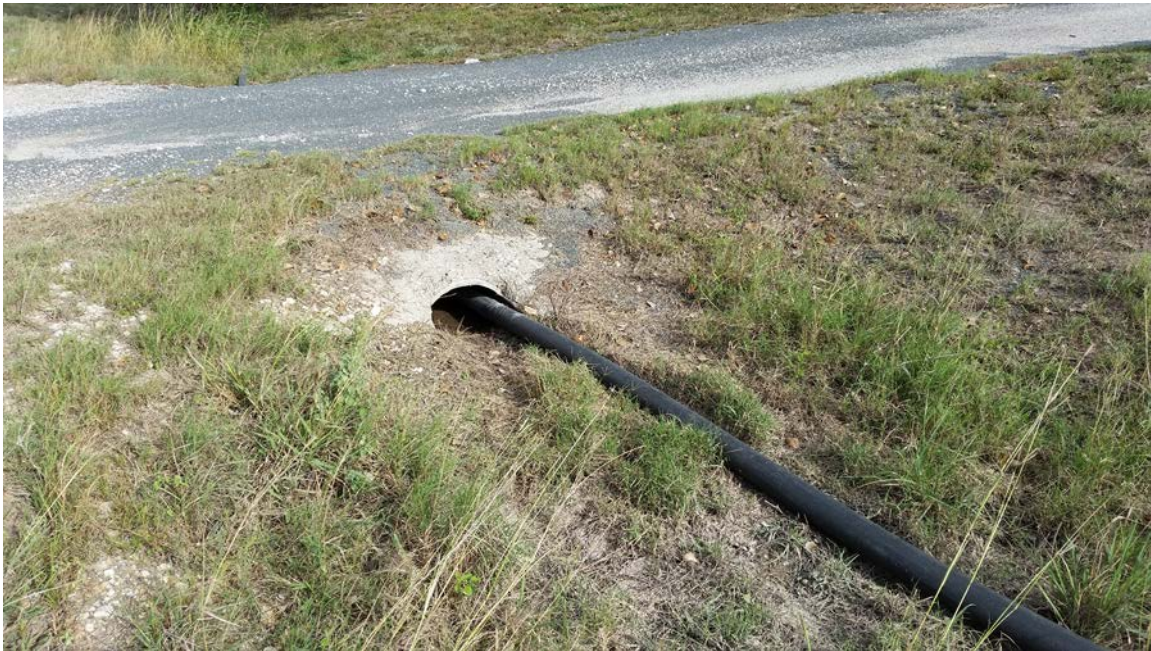
Figure 17. Temporary Pipeline Installed in Driveway Culvert.
