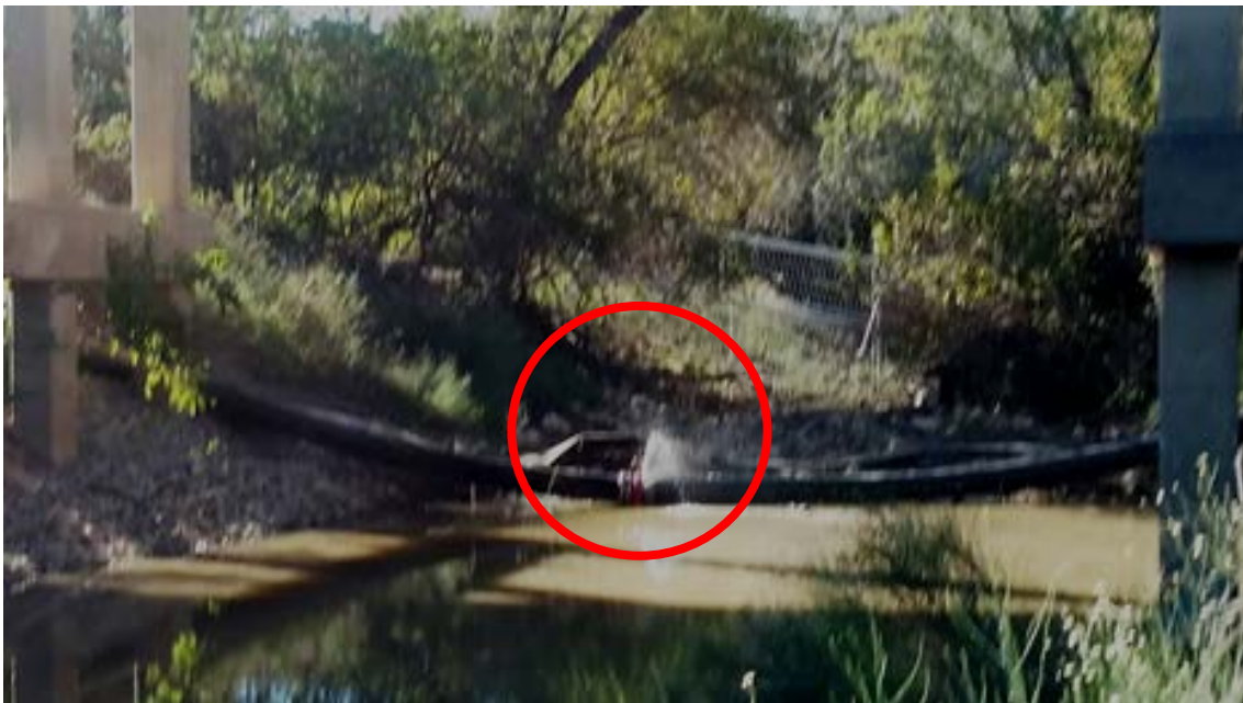
Figure 20. Temporary Pipeline Water Leak on a Water Stream in the Eagle Ford Shale Region.
