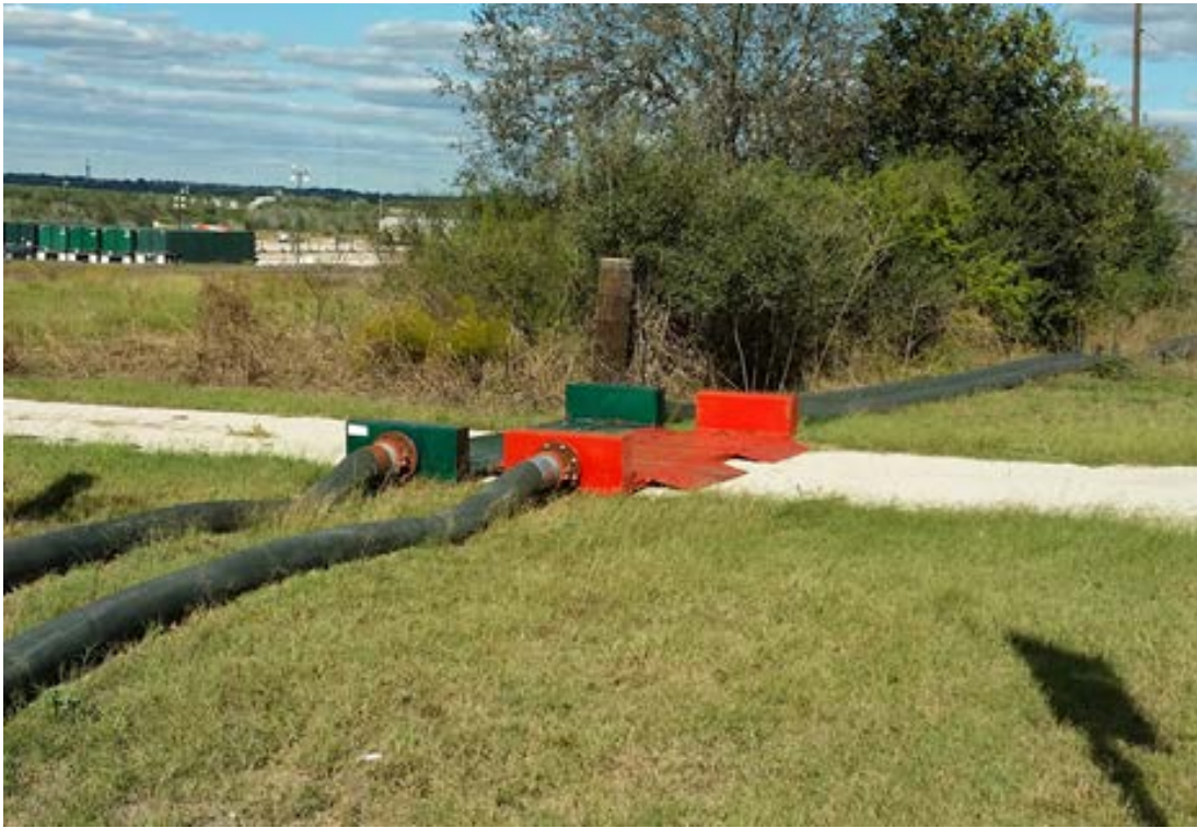
Figure 15. Temporary Pipeline Driveway Crossing Ramp and Manifold.
