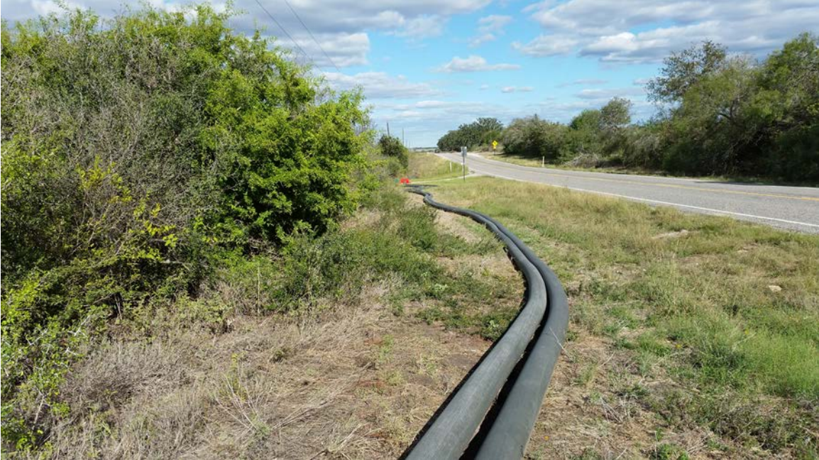
Figure 22. Temporary Pipeline Installation around Vegetation.
