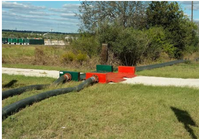
Figure 13. Temporary Pipeline Driveway Crossing Ramp and Manifold.
