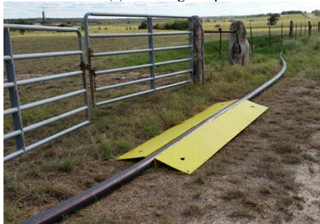
(a) Crossing ramp
