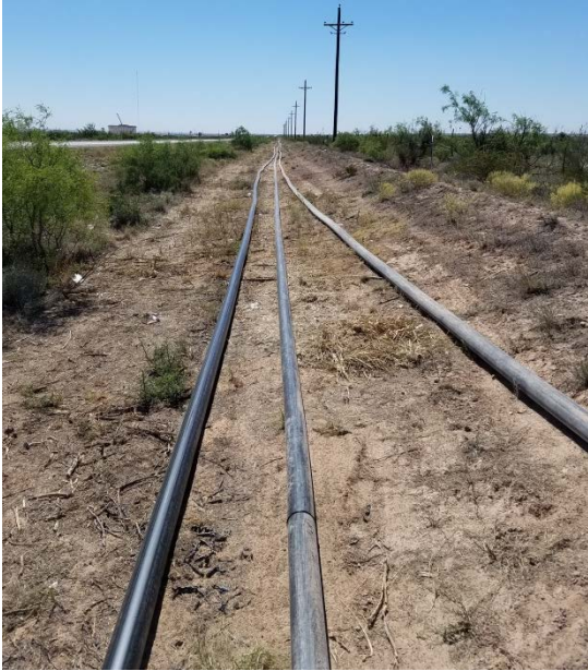
Figure 7. Polyethylene and Lay-Flat Temporary Pipelines.
