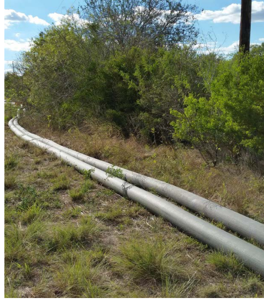
Figure 7. Polyethylene and Lay-Flat Temporary Pipelines.
