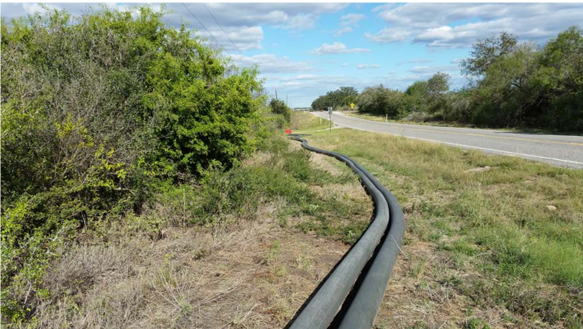
Figure 2. Temporary Pipeline Installation around Vegetation.
