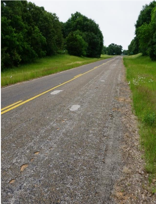
Before FDR (photo courtesy TxDOT-BRY)
