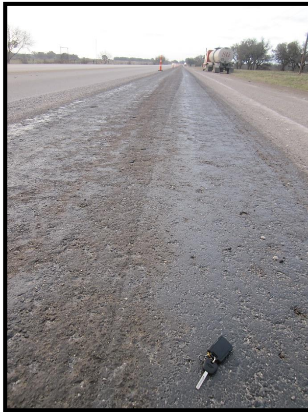
Figure 8. Treated, Finished Section after Fog Seal.
