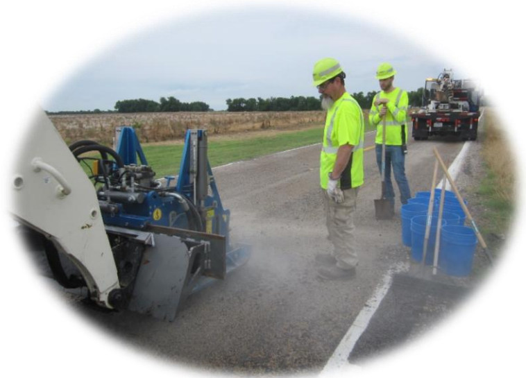
Generating sample for mix design
