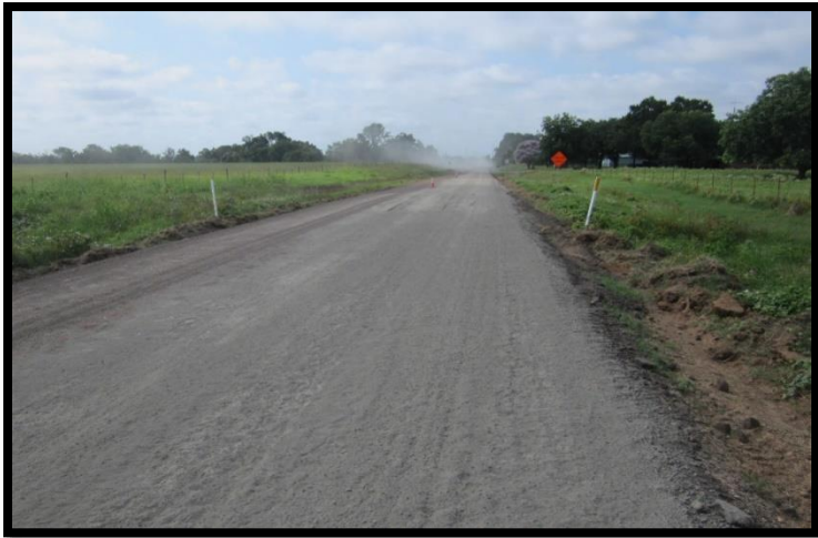
Spreading additive
