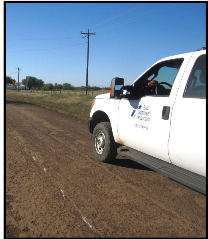
Painted cut line for reclaimer to follow
