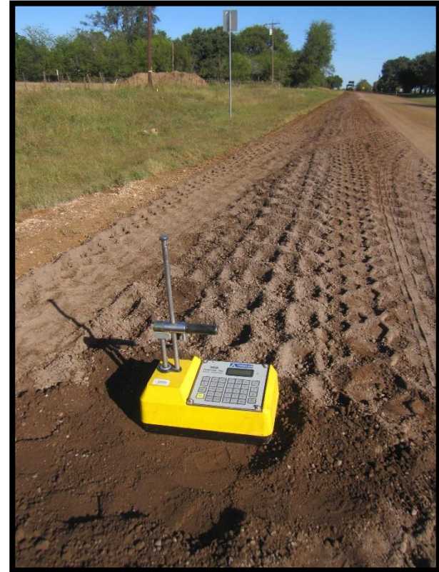
Existing moisture also checked during pulverization check
