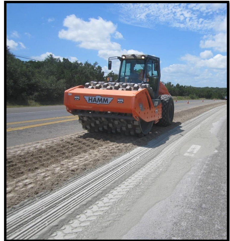
Compacting FDR mix
