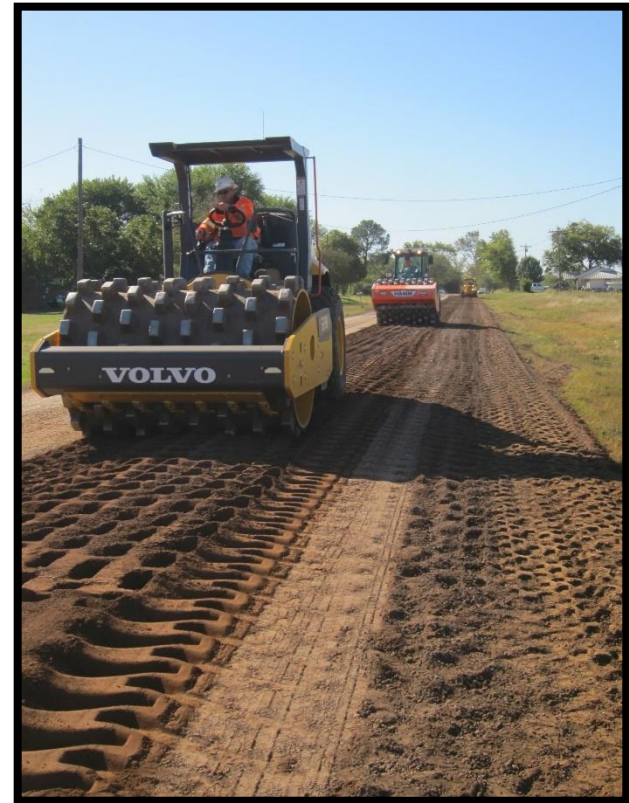
Using 2 padfoot rollers for compaction
