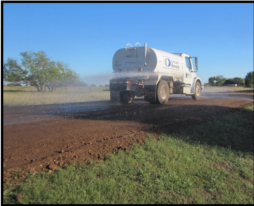
Sprinkling to preserve surface moisture during finishing
