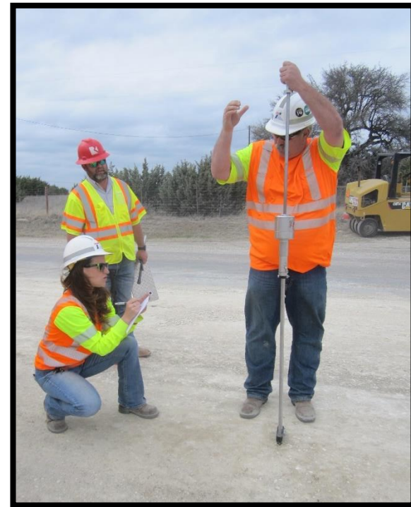
Checking 10" layer thickness with DCP for compaction uniformity
