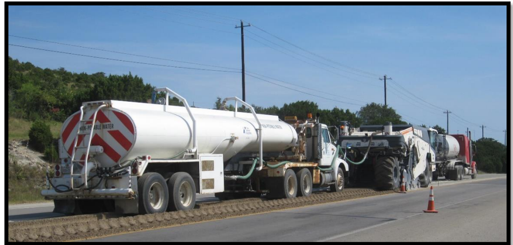
Pulverization, application of oil and moisture in one pass
