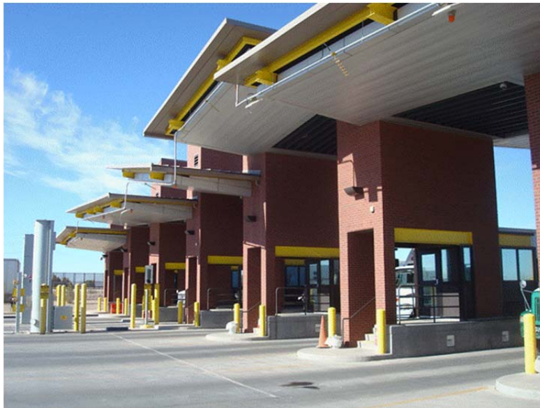
Figure 30. RFID Readers Installed at CBP’s Primary Inspection Facility at the Ysleta-Zaragoza POE.
