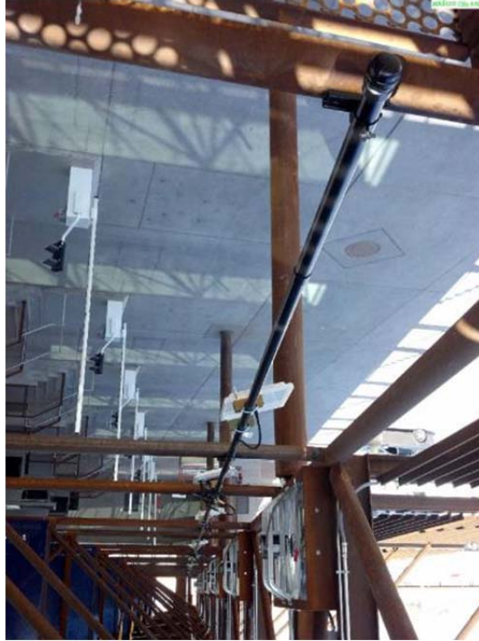
Figure 31. RFID Readers Installed at CBP’s Primary Inspection Facility at the Mariposa POE.
