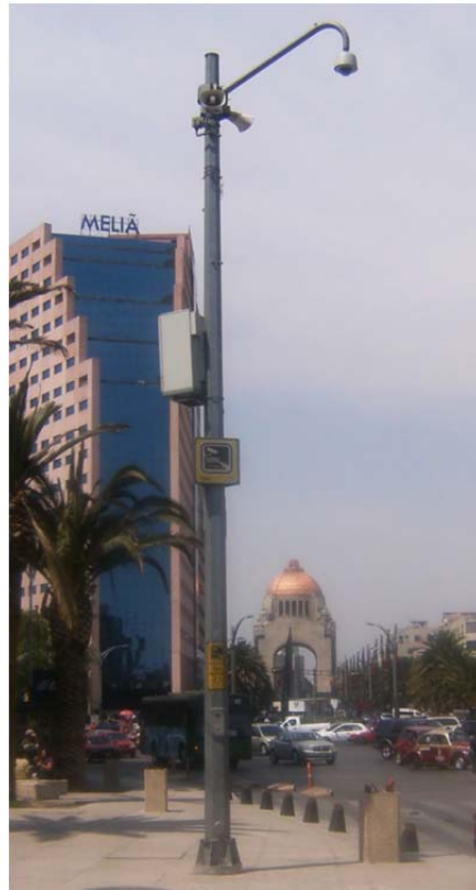
Figure 22. PTZ IP Cameras Installed in Mexico City.
