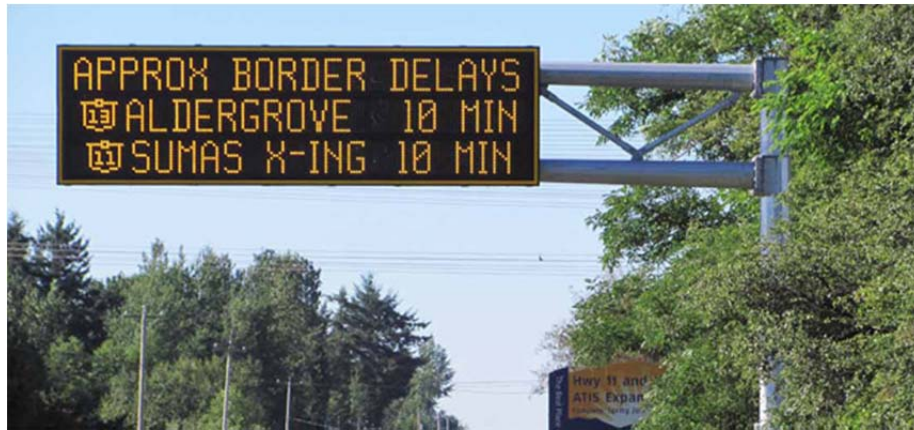
Figure 45. Different Kind of DMS Installed on the Same Roadway Leading to the United States from Canada.
