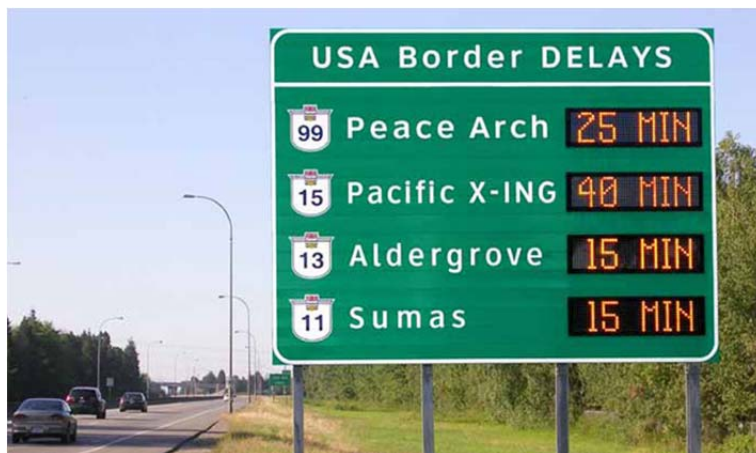
Figure 44. DMS Installed on the Canadian Side of the Border with Washington State.
