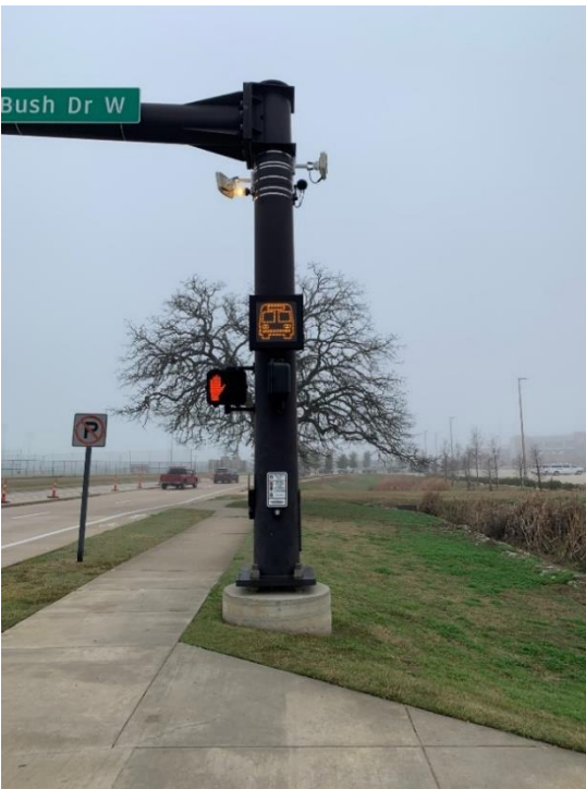
Figure 7. Location of FLIR Sensors on Traffic Pole.
