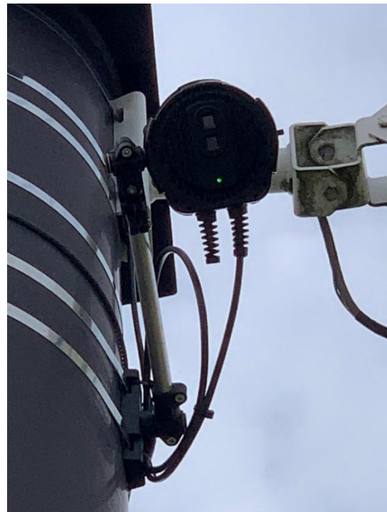
Figure 7. Location of FLIR Sensors on Traffic Pole.
