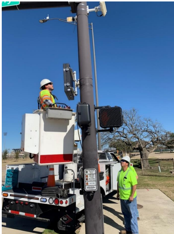
Figure 11. City of College Station Personnel Installing Equipment.
