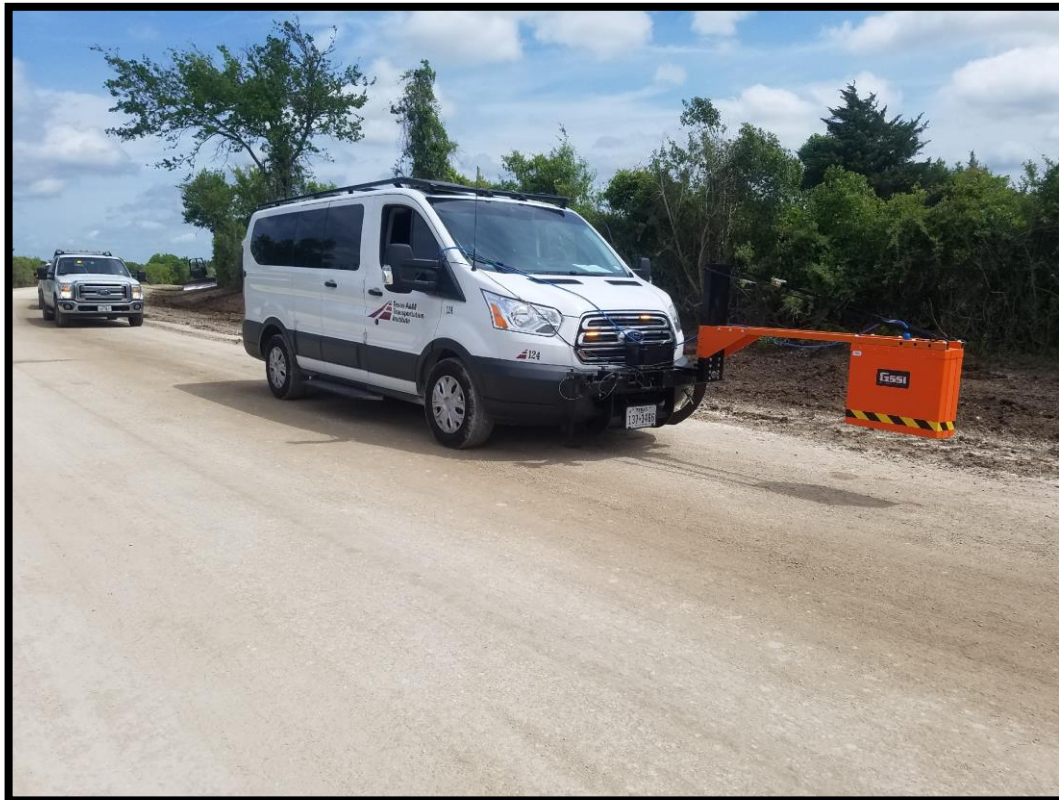
GPR testing on Completed Base Course
