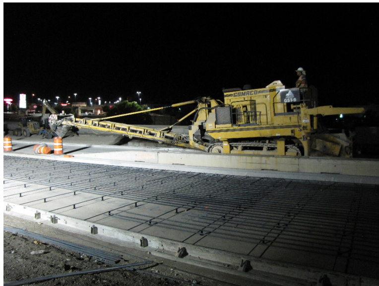
Figure 17. Concrete Slip Paver in Temple.
