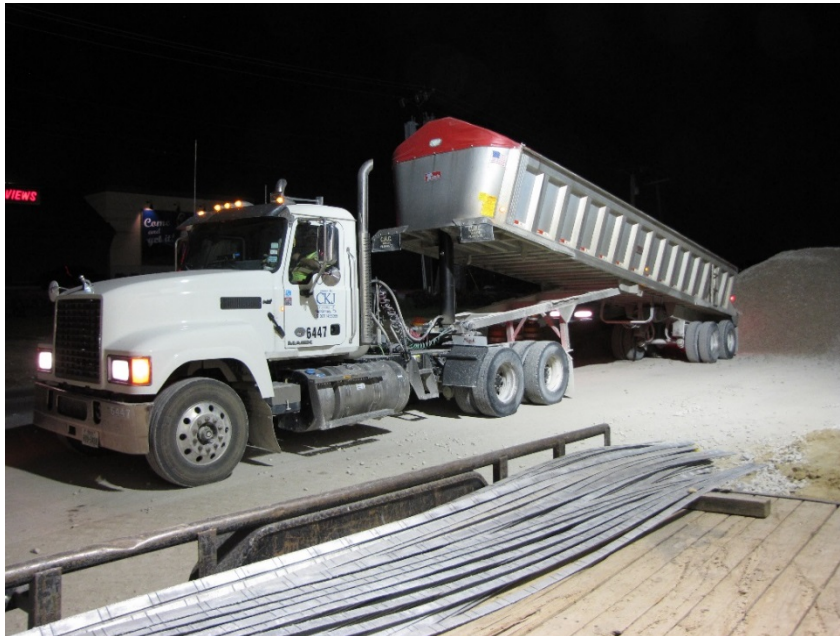
Figure 19. Dump Truck Unloading Crushed Stones during the Nighttime.
