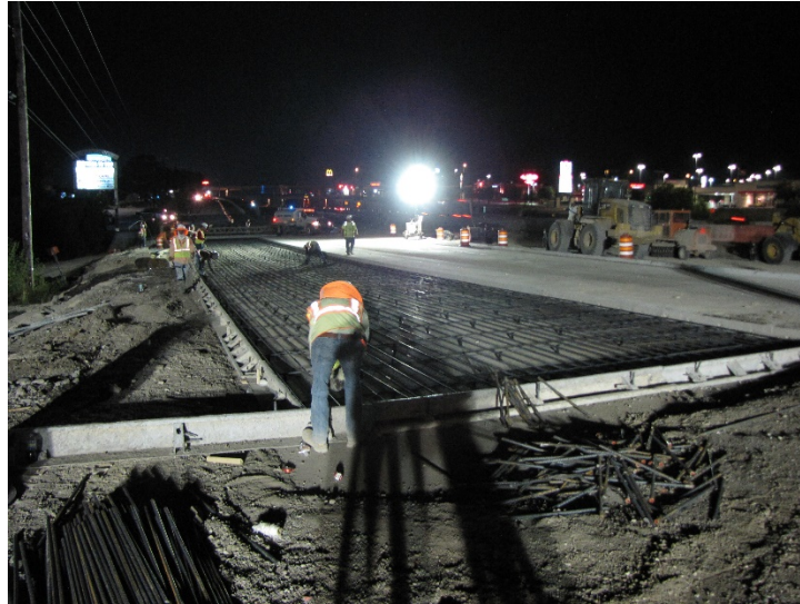
Figure 16. Workers on Setting Forms for Concrete Pour in Temple.
