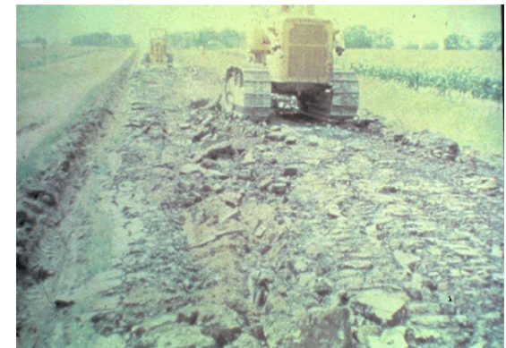
Ripping and crushing
