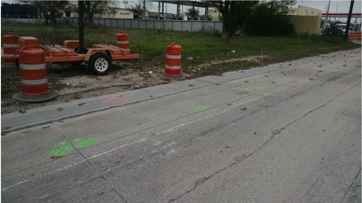
Figure 168. Solms Rd. Patching of Longitudinal Cracking.
