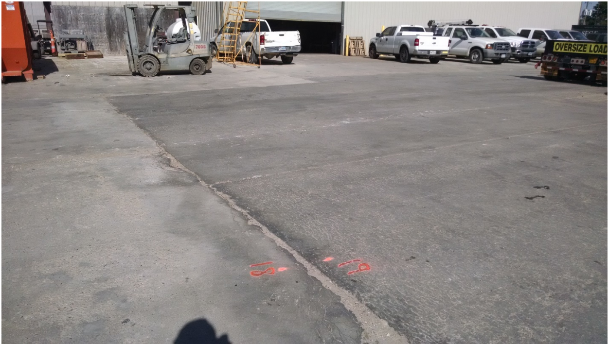
Figure 152. Construction Joint from Transverse to Longitudinal (December 2015).
