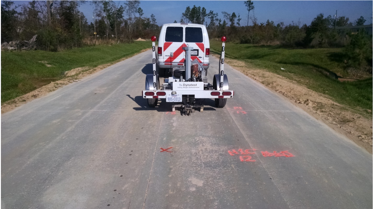
Figure 164. Bella Vista Natural Subgrade.
