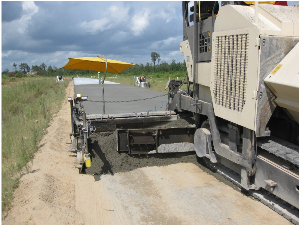
Figure 155. Bella Vista Paving Operation (July 2015).
