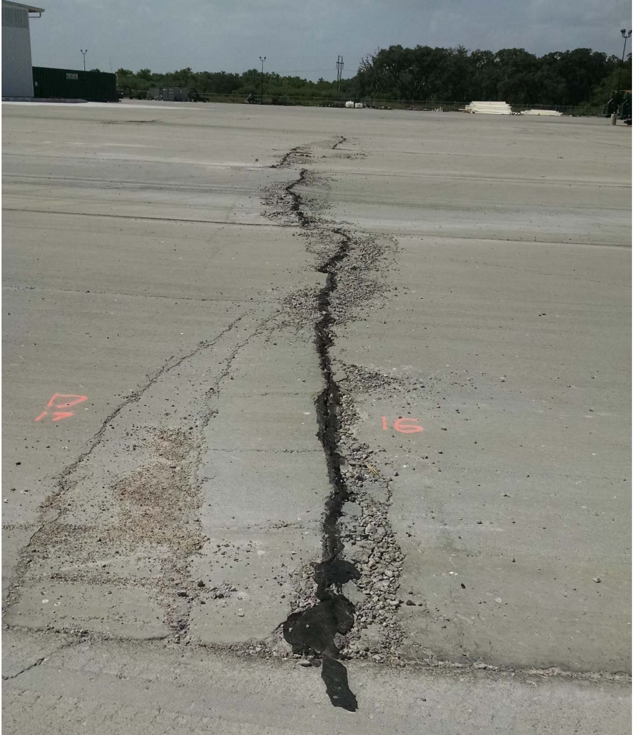
Figure 148. Pioneer Locations 16 and 17 (Major Blow-Up).
