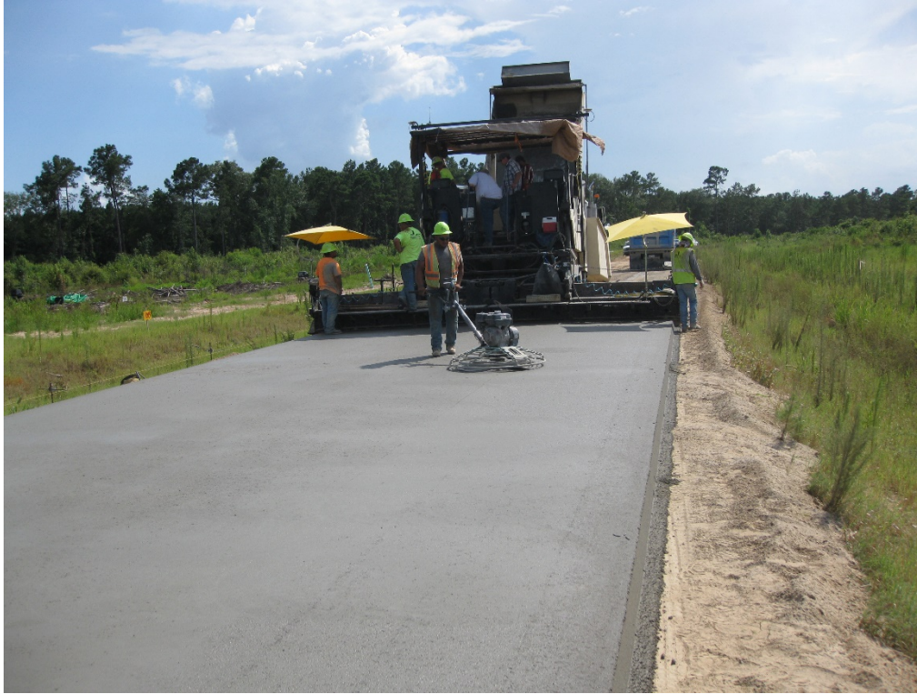
Figure 156. Bella Vista Finishing Operation.
