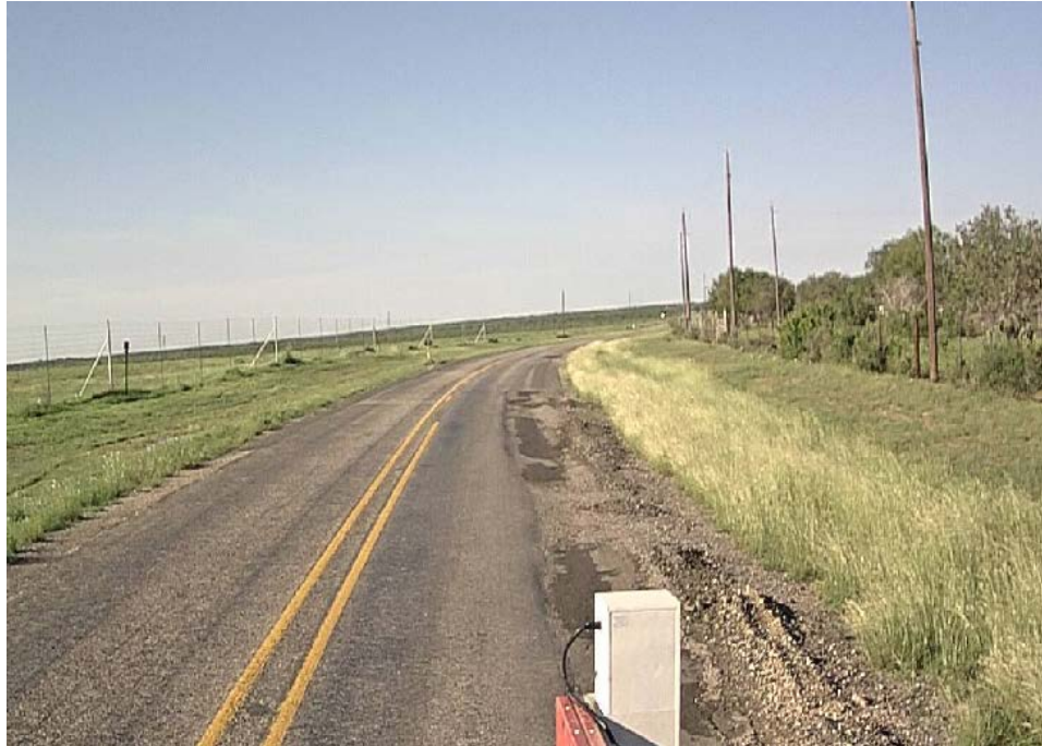
Figure 25. Pavement Condition prior to Construction.
