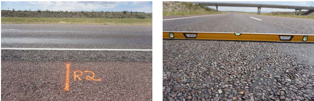
Figure 48. Pictures of Pavement Surface and Rutting: (a) No Cracking and (b) Rutting.
