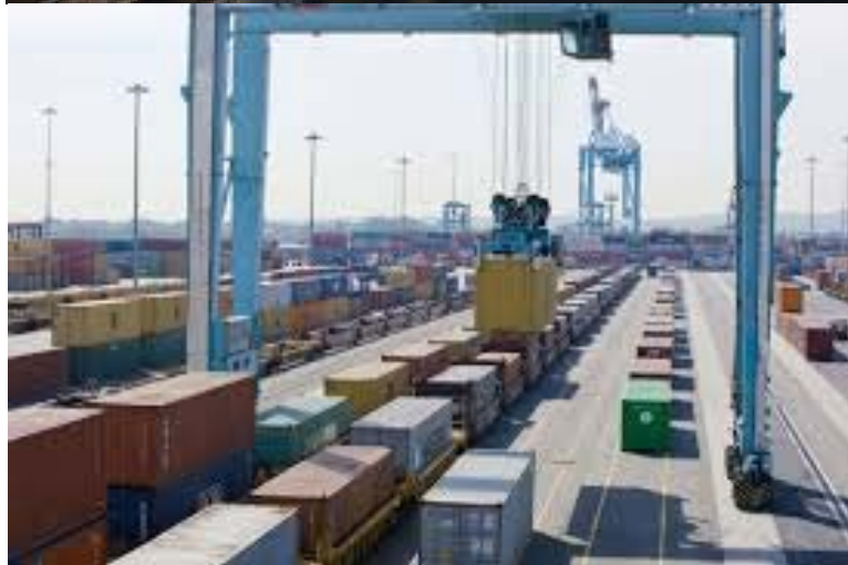
Figure A-37. Images of On-Dock Rail.
