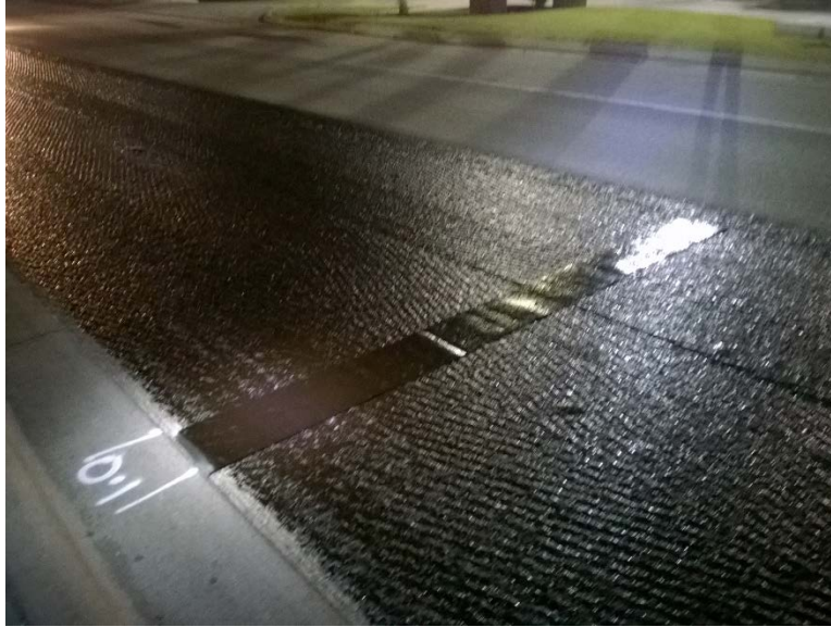
Figure 6-4. Measurement of Tack Application Rate (ASTM D2995).
