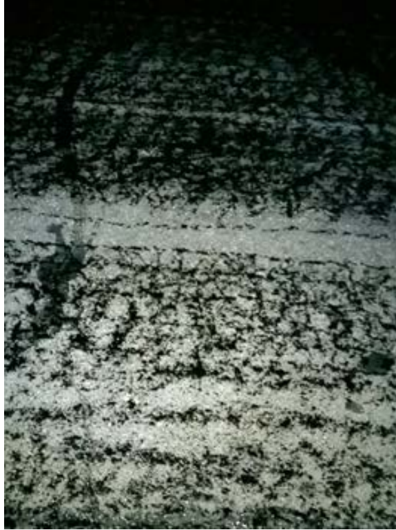
Figure 6-5. Non-Uniformity of Tack C Application.
