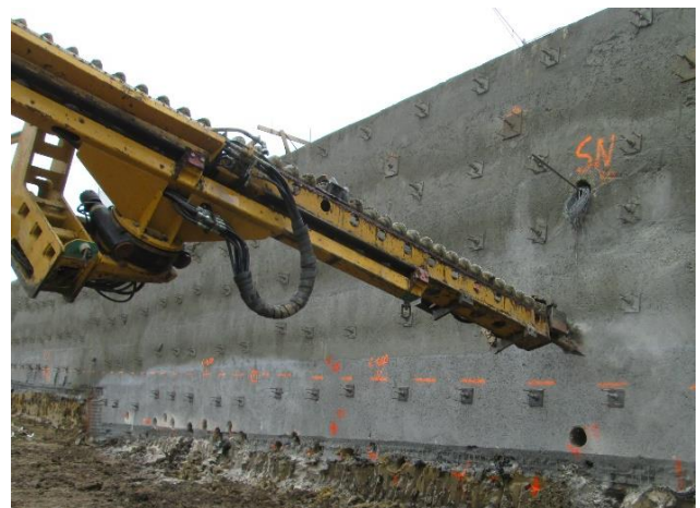
Figure 1. Soil Nail Wall.
