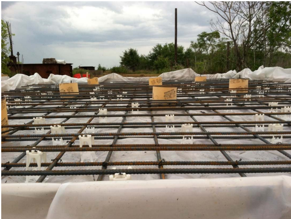
Figure 99. Placing the Top Layer Reinforcement.
