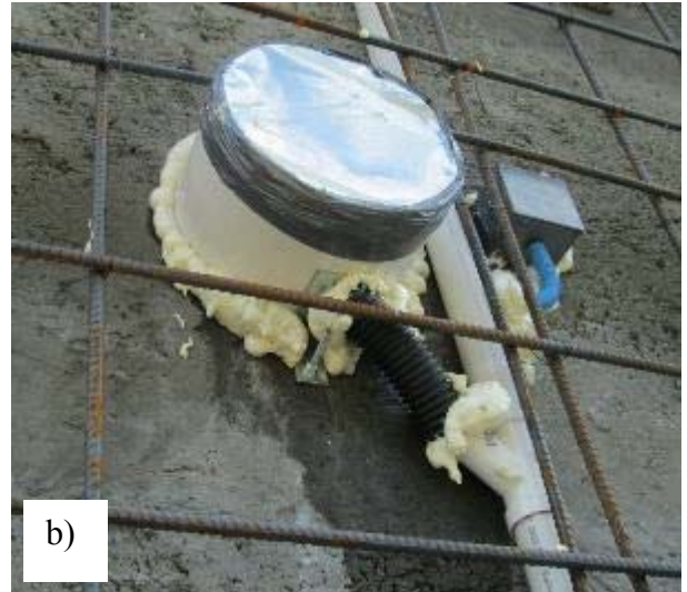
Figure 240. a) Cover Plate at Top of the PVC Tube; and b) Seal the PVC Pipe to the Shotcrete Facing.
