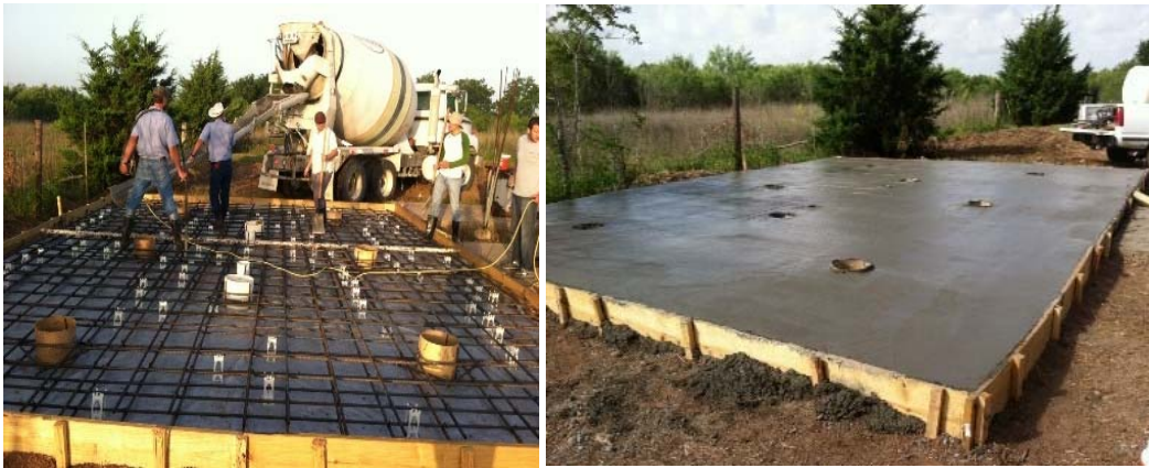
Figure 101. Pouring the Concrete.
