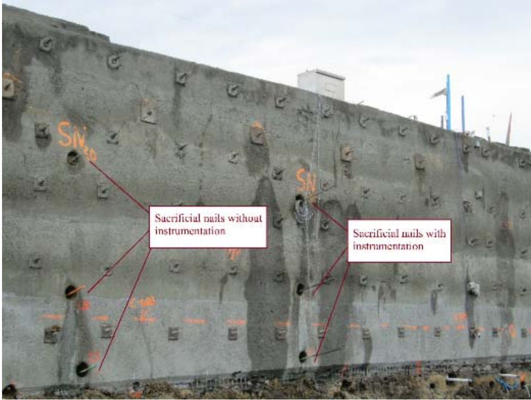
Figure 157. Installation of the Sacrificial Nails at Different Heights of the Wall.
