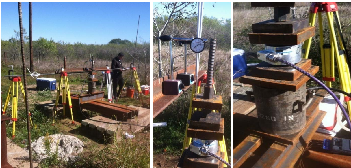
Figure 109. Details of Load Test Setup for Nails outside the Concrete Slab (i.e., Nails NS1, NS2, and NW1 to NW8).
