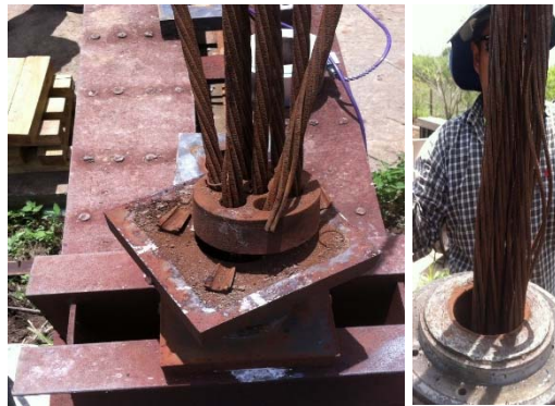
Figure 64. Failure of Anchor 3 and 4 Tendons during the Test at 238 Kips.
