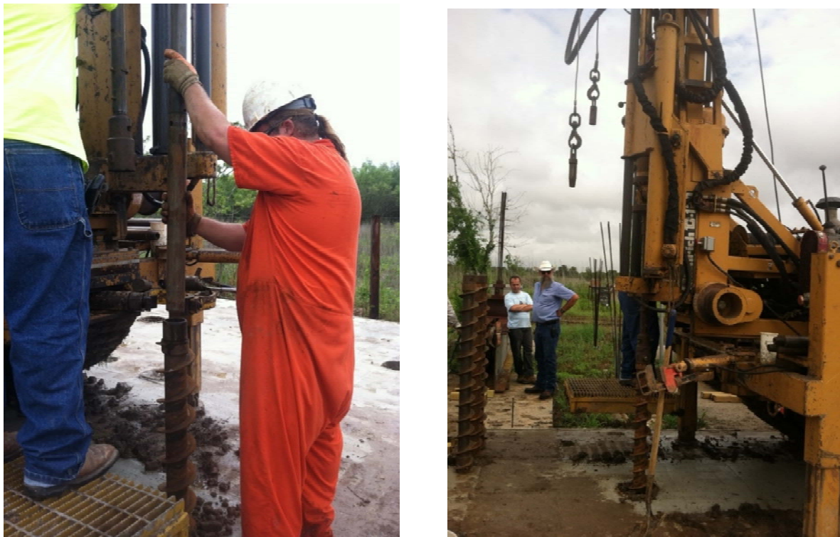
Figure 103. Drilling the Holes.
