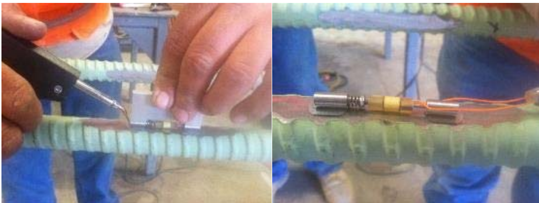
Figure 214. Welding the Gauges to the Nail Bars with Spot Welder.
