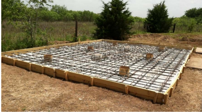
Figure 100. Placing the Wood Frame.
