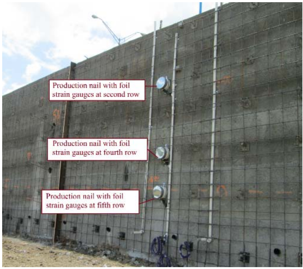
Figure 205. Instrumented Production Nails with Foil Strain Gauges at Station 2+06.
