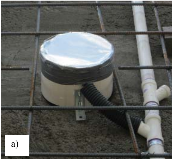
Figure 240. a) Cover Plate at Top of the PVC Tube; and b) Seal the PVC Pipe to the Shotcrete Facing.
