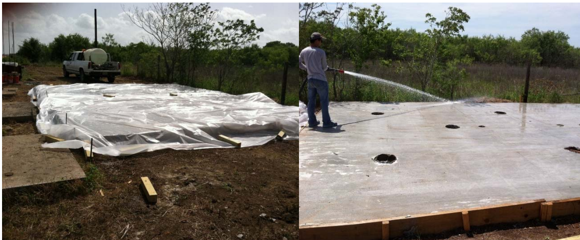
Figure 102. Curing the Concrete.
