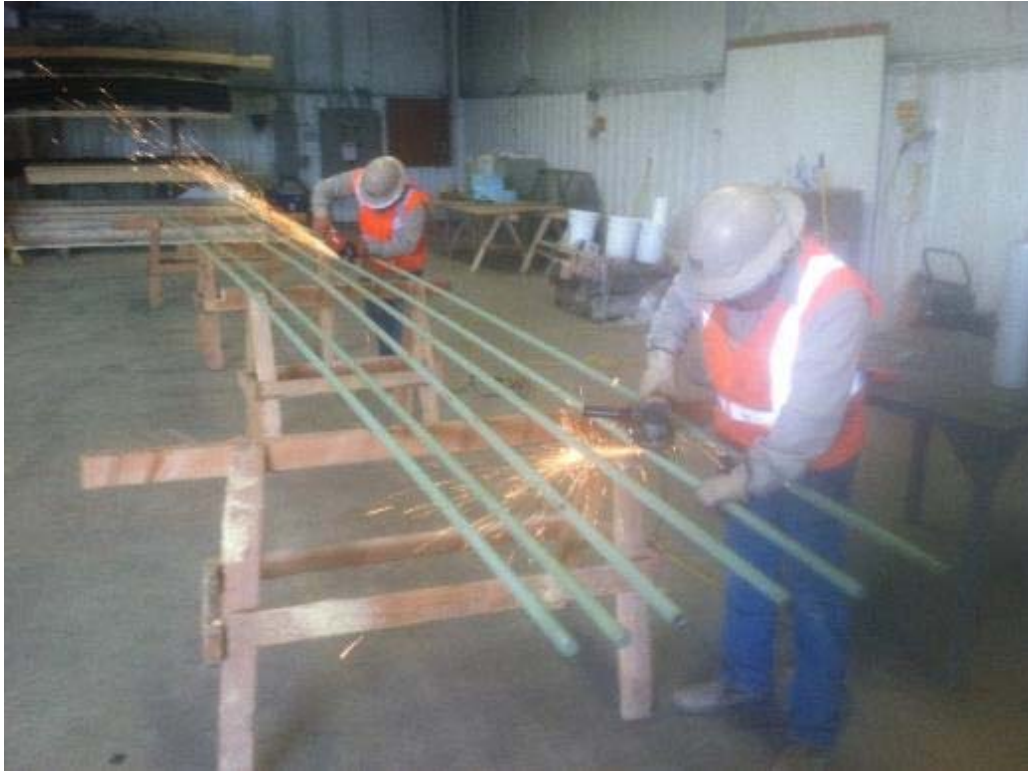
Figure 213. Grinding Nail Bars at Designated Position with Electric Grinder.
