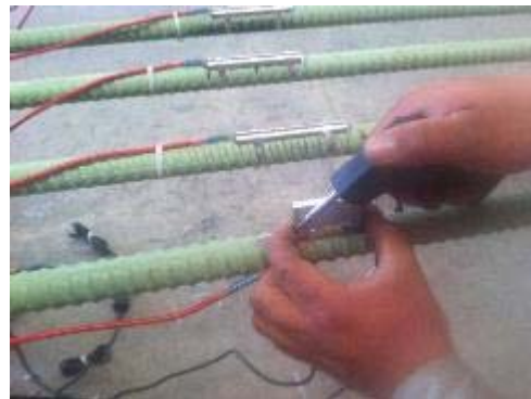
Figure 216. Installing the Aluminum Cover.
