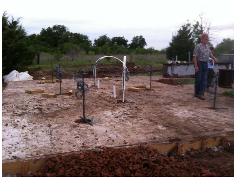
Figure 107. Final View of the Installed Soil Nails on Concrete Slab.
