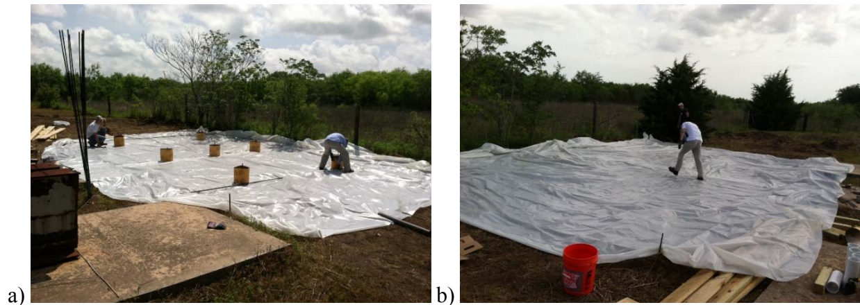
Figure 97. a) Laying Plastic Membrane; b) Marking Nail Locations.
