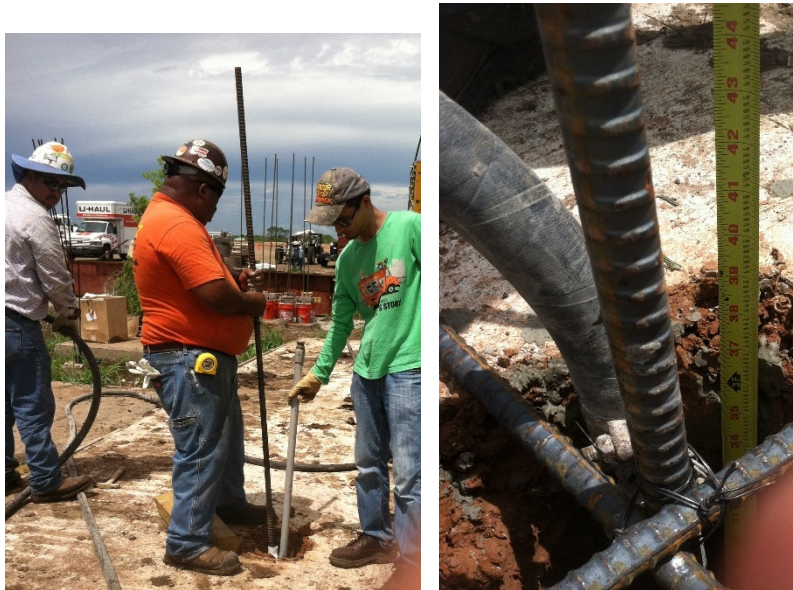
Figure 106. Grouting and Nail Installation.
