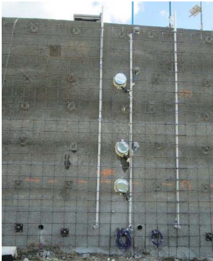
Figure 241. Pipes Used to Conduct the Load Cell Cables to the Ground.
