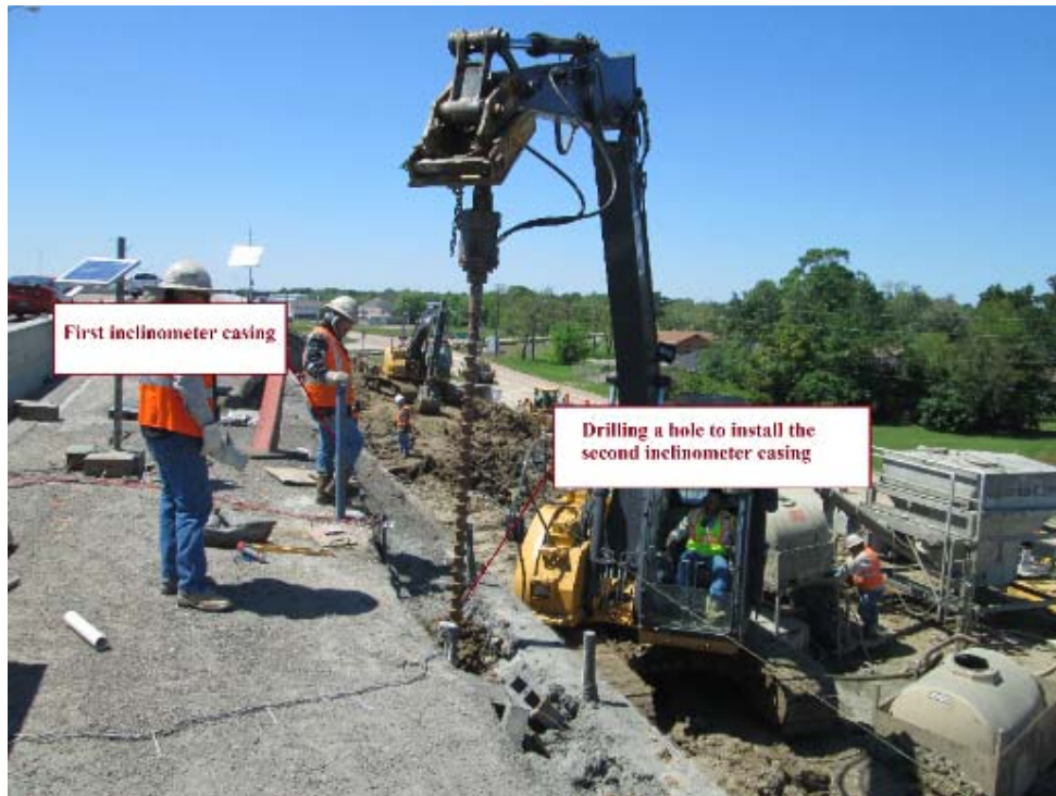
Figure 187. Installation of the Second Inclinometer Casing at Station 2+00 on April 14.
