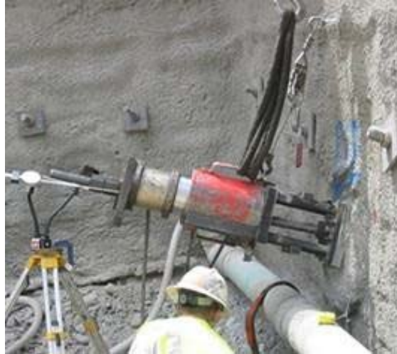
Figure 39. A Nail Load Test Performed in Inclined Soil Nails.
