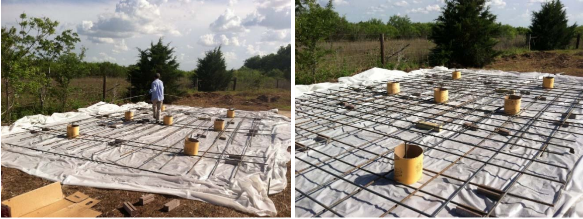
Figure 98. Placing the Bottom Layer Reinforcement.
