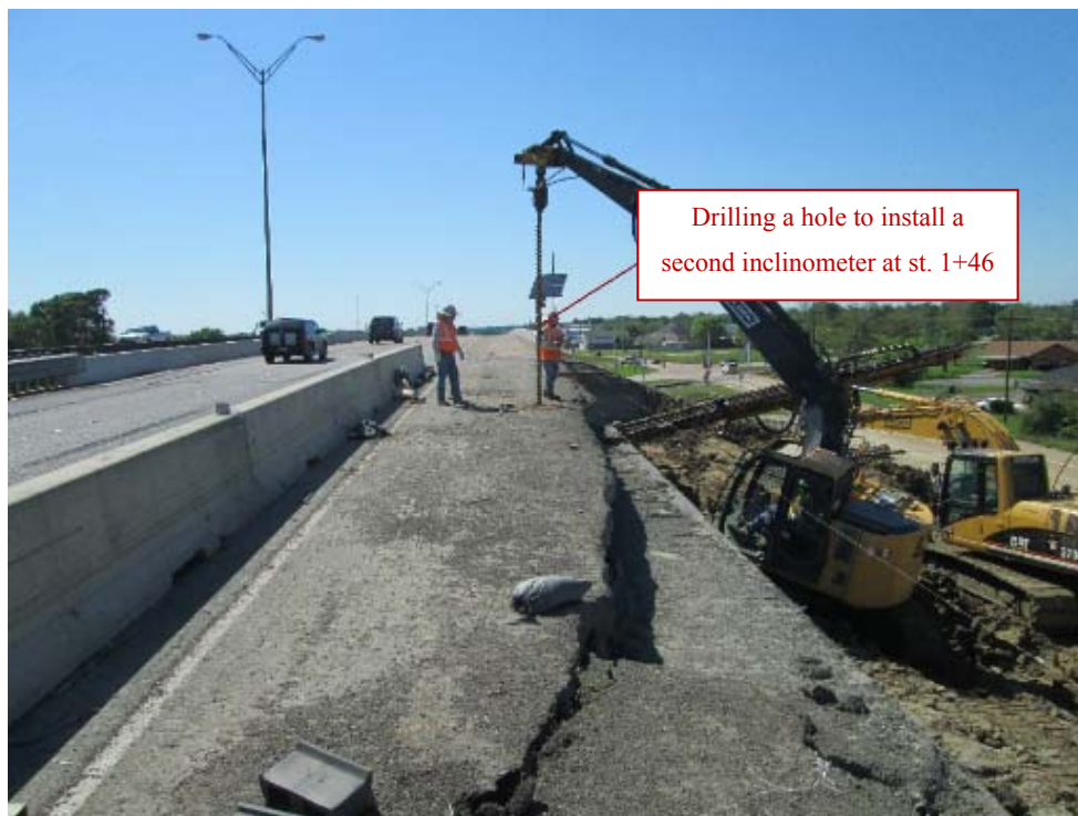
Figure 188. Installation of Second Inclinometer Casing at Station 1+46 on April 14.
