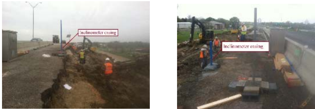
Figure 185. First Inclinometer Casing at Station 2+00.
