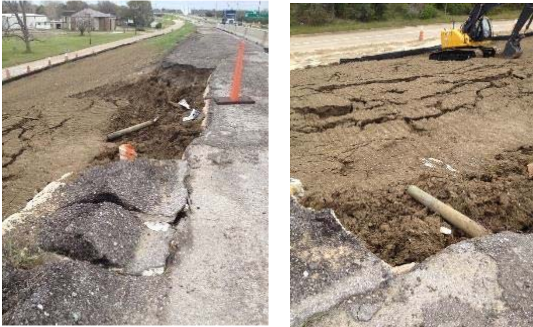
Figure 148. Condition of the Embankment Soil before the Project Was Started.
