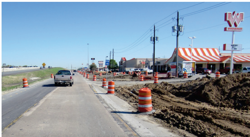
Figure 17. Typical Work Zone Setup at McKinney Driveways.
