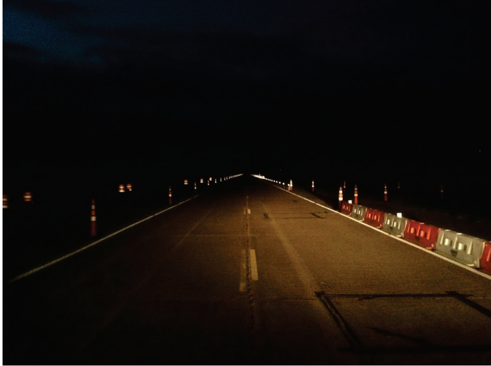
Figure A-37. Treatment 6: 18-Inch LCDs on Main Lane with 42-Inch Cones on Driveway.
