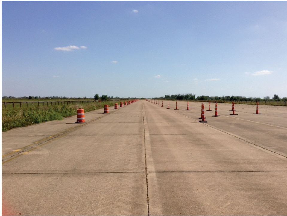
Figure A-23. Treatment 1: 42-Inch Cones on Main Lane with 42-Inch Cones on Driveway.
