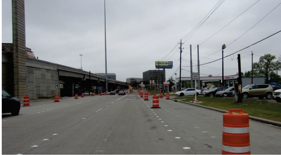
Figure 18. Typical Work Zone Setup at Houston Driveways.
