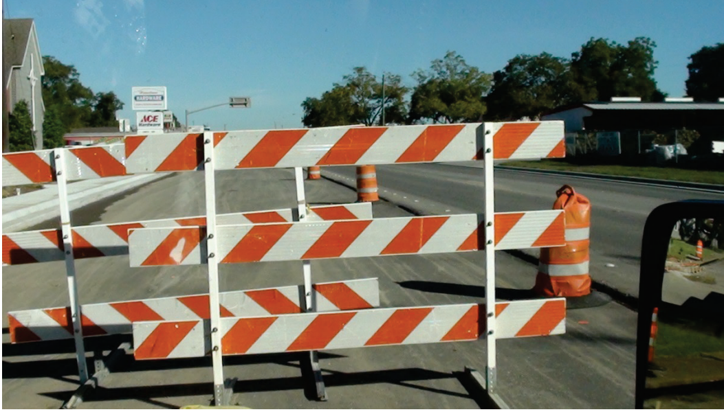
Figure 5. Type 3 Barricades in a Texas Work Zone.
