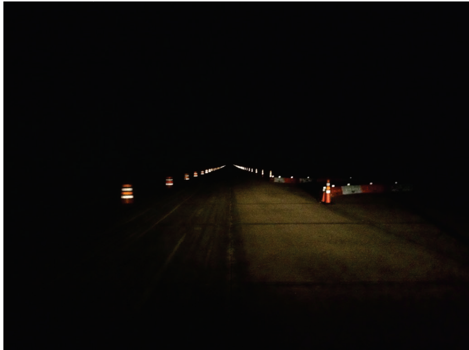
Figure A-34. Treatment 3: 42-Inch Cones on Main Lane with 18-Inch LCDs on Driveway.
