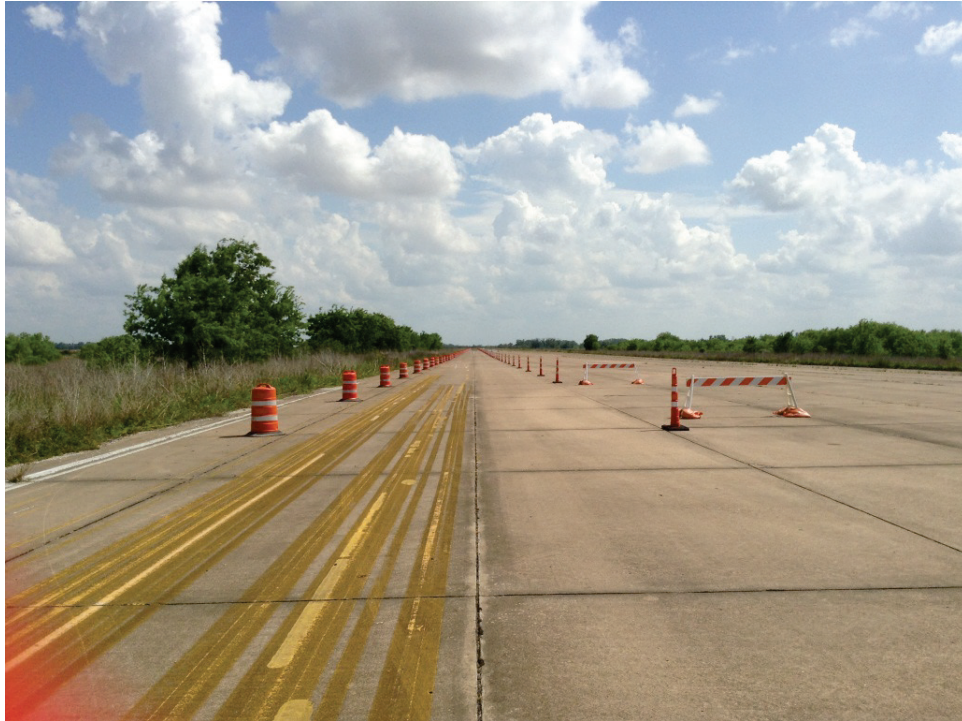
Figure A-26. Treatment 4: 42-Inch Cones on Main Lane with 36-Inch Type I Barricades on Driveway.
