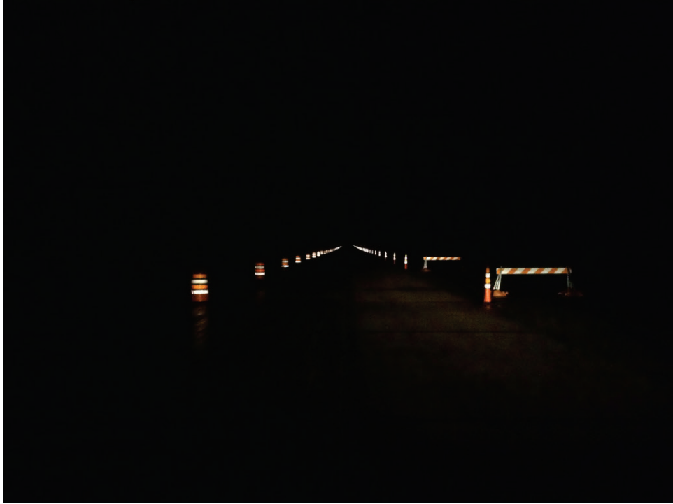
Figure A-35. Treatment 4: 42-Inch Cones on Main Lane with 36-Inch Type I Barricades on Driveway.
