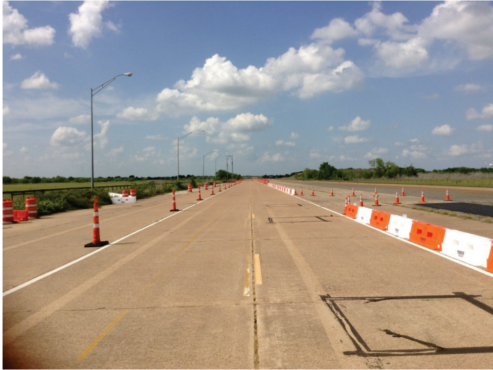
Figure A-29. Treatment 7: 18-Inch LCDs on Main Lane with 28-Inch Cones on Driveway.
