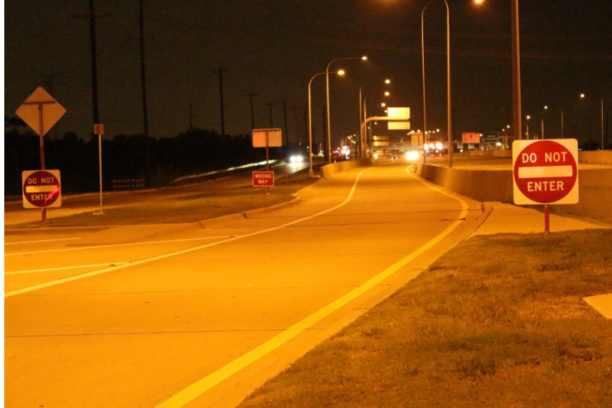
Figure 4. Example of NTTA DO NOT ENTER and WRONG WAY Lowered Signs.
