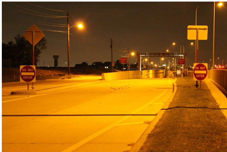
Figure 3. Example of NTTA DO NOT ENTER Lowered Signs.
