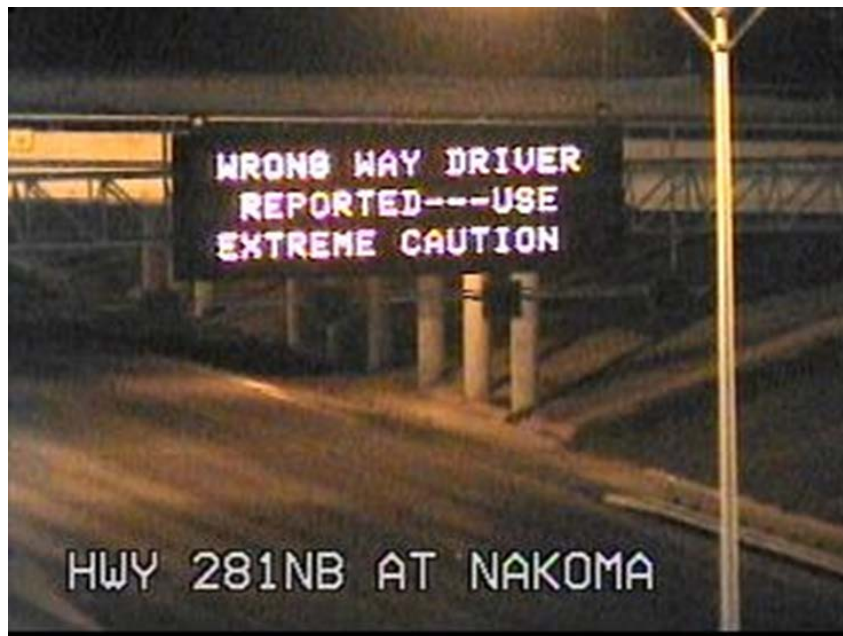
Figure 46. TxDOT's San Antonio District Wrong Way Driver Warning Message.
