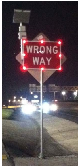
Figure 7. Example of WRONG WAY Sign with Flashing Red LEDs around Border.
