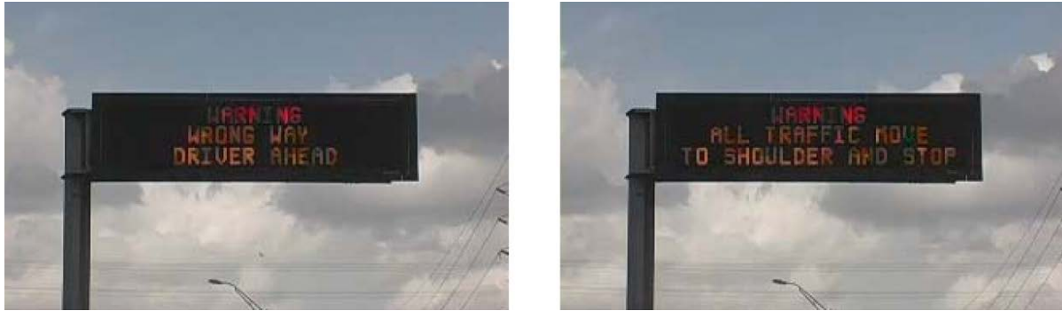
Figure 47. HCTRA's Wrong Way Driver Warning Message (34).
