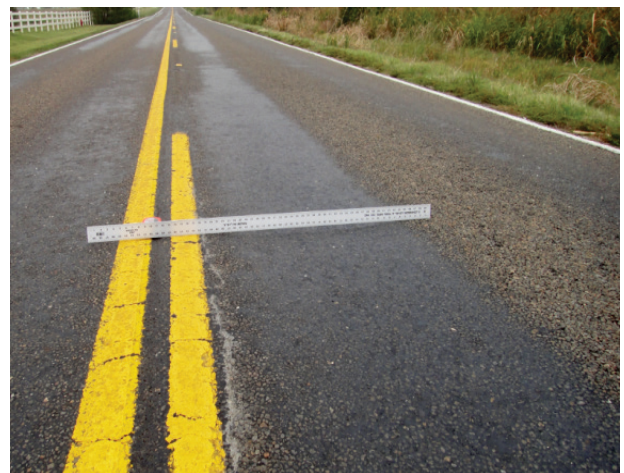
FIGURE 5 – Surfaces Exhibiting Minor Rutting Are Acceptable.
