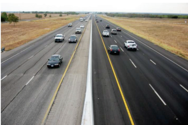
FIGURE 2 – TOM on IH 35 Under Construction – Placed in 2009 and Still Performing Excellently.
