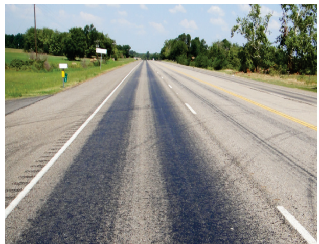
FIGURE 6 – PFC-F Can Be Placed over This Flushed Seal Coat.
