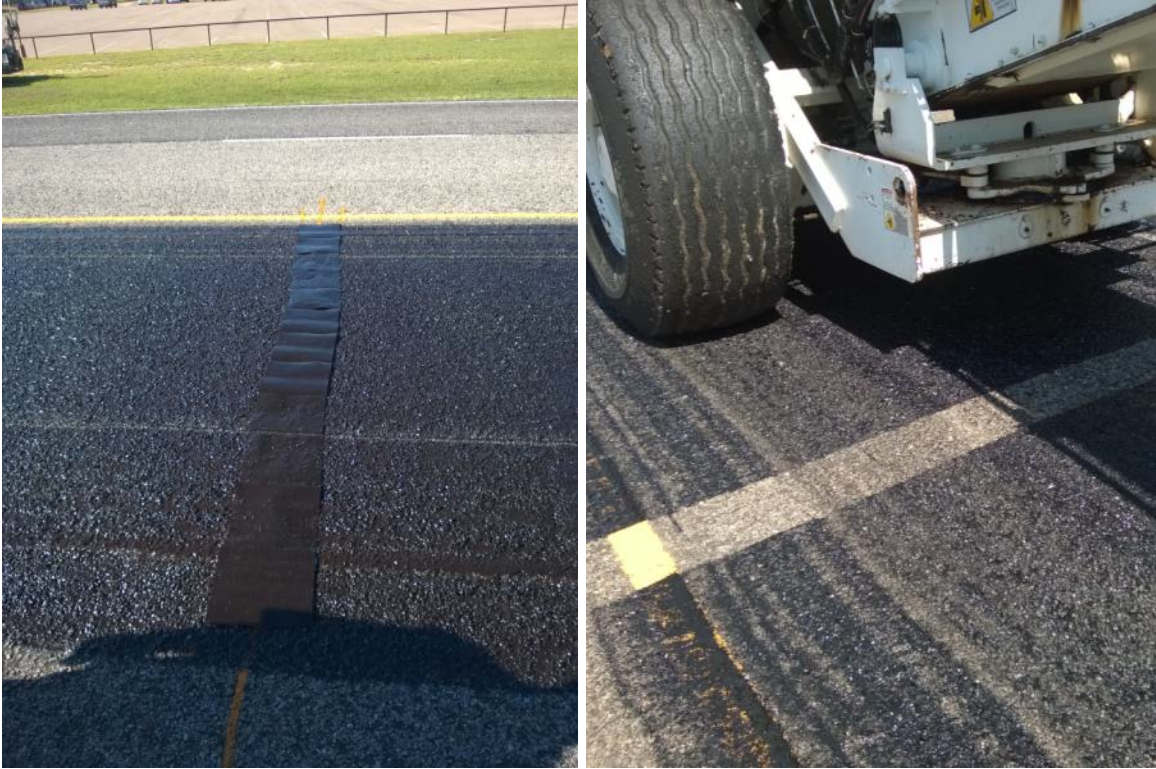
Figure G.10. Measuring Tack Application Rate.
