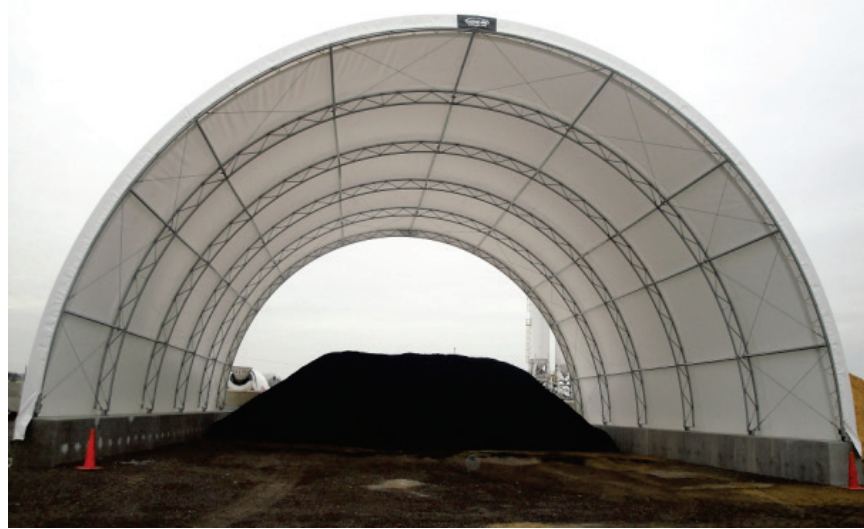
Figure 27. Covered RAS Storing Facility.
