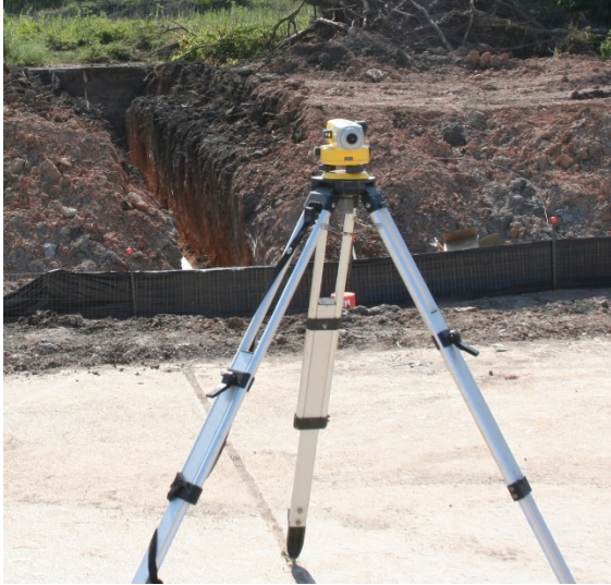
(a) Trench Excavation
