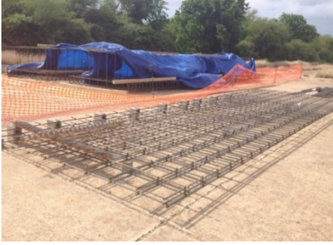
(a) Rebar Tying
