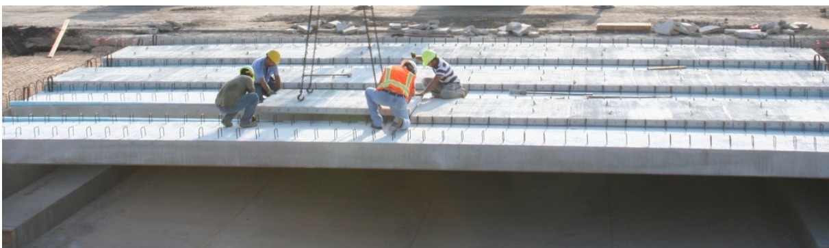
(c) Erection of Precast Concrete Panels
