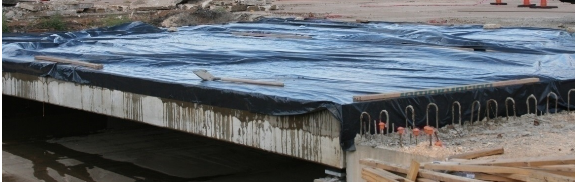
Figure B.23. Curing of Deck Concrete.
