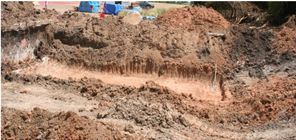
(b) Excavation for Slab on Grade below Footings
