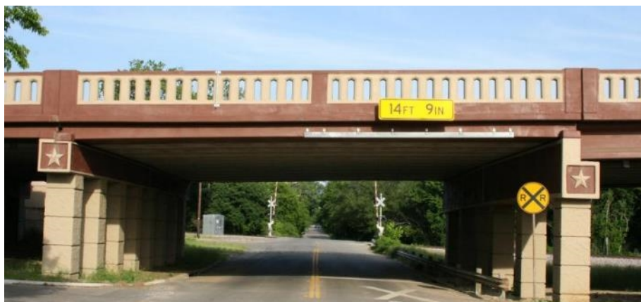
(c) Elevation View of 50 ft Northbound Bridge Span over Day Street
