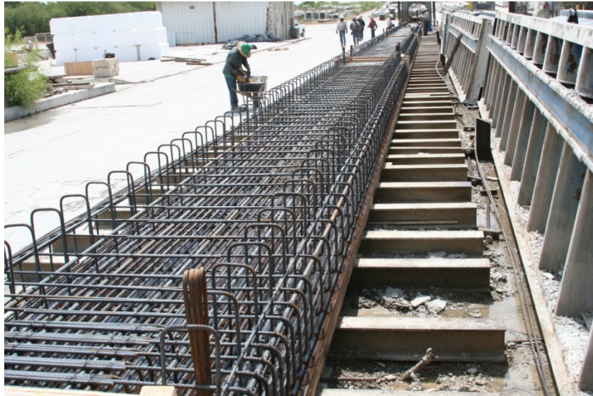
(a) Slab Beam Reinforcing Bar Placement
