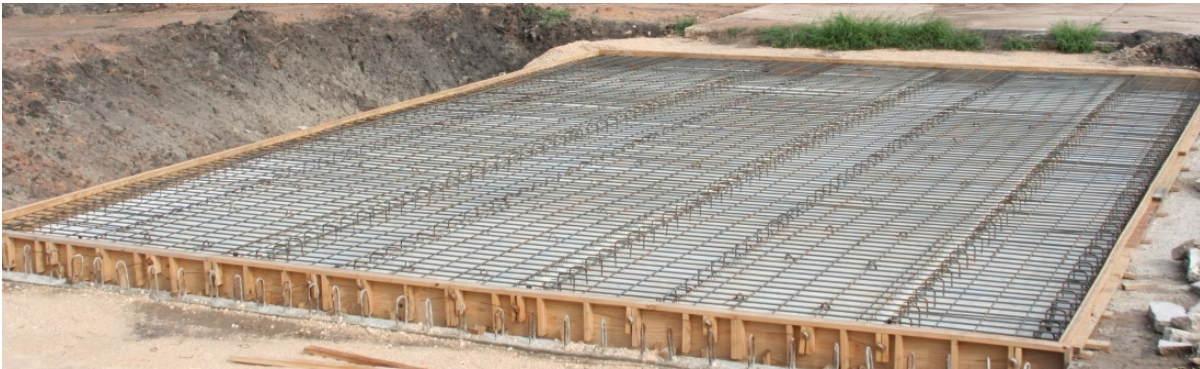
(b) Deck Reinforcing Bar Construction
