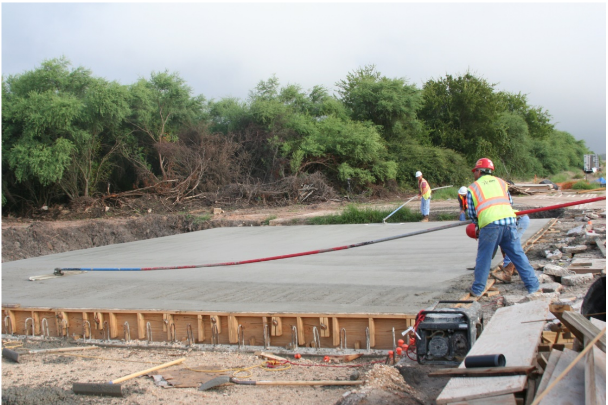
Figure B.22. Deck Concrete Finishing.
