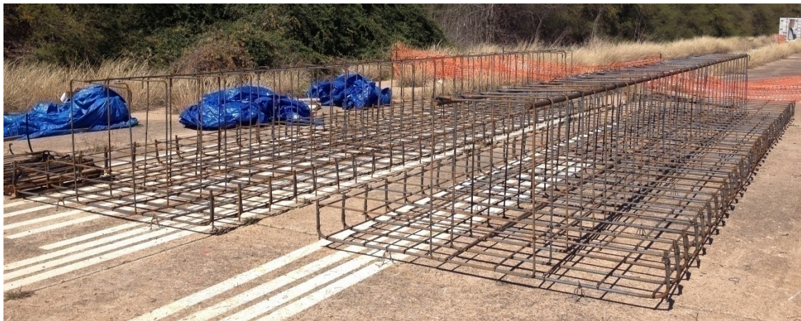
Figure B.12. Footing and Abutment Reinforcement Cage.
