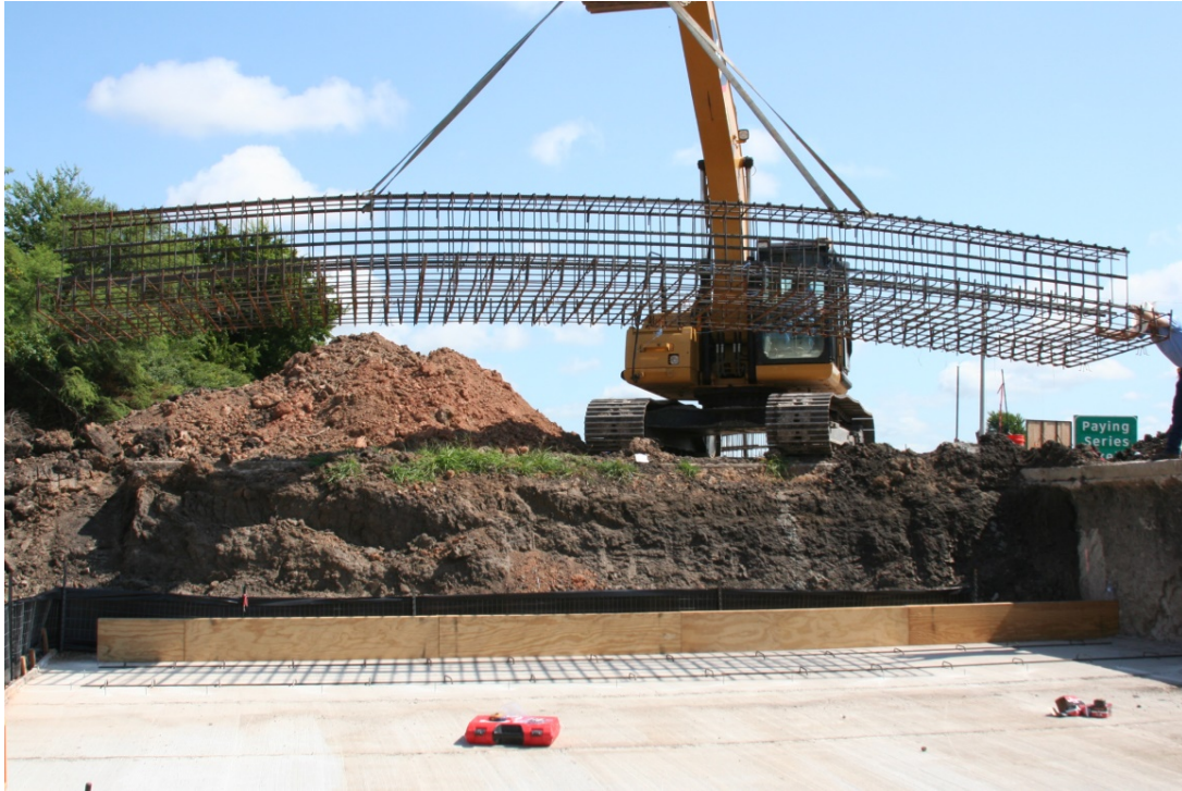
(a) Reinforcing Cage Placement
