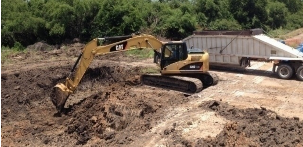
(a) Main Excavation of the Bridge Foundation
