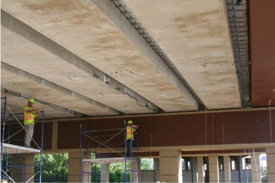
(a) Instrumentation Installation Underneath the Bridge
