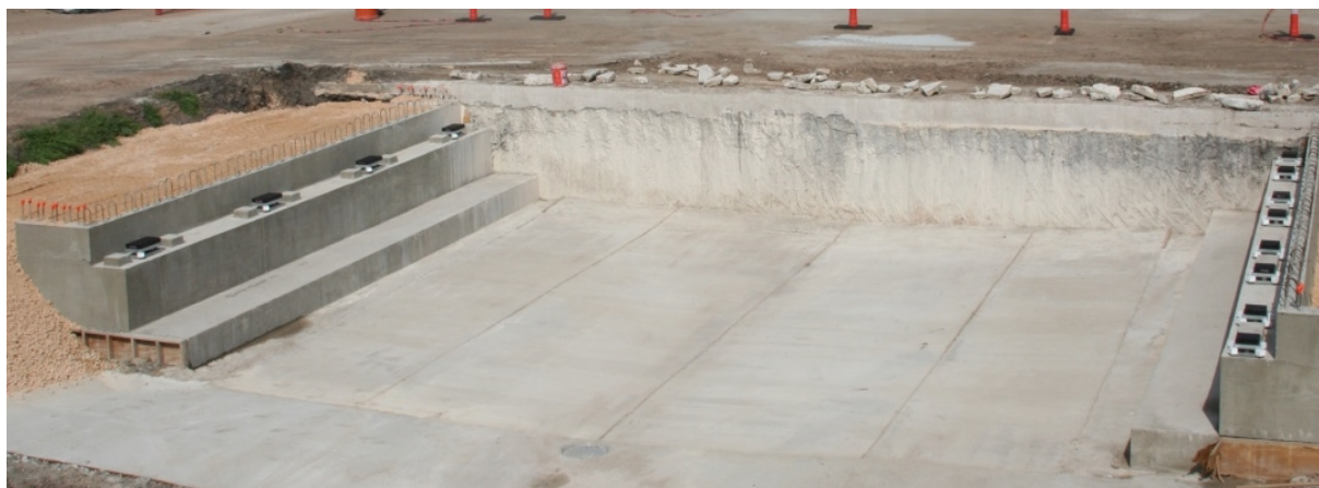
(c) Bridge Span Ready to Receive Slab Beams
