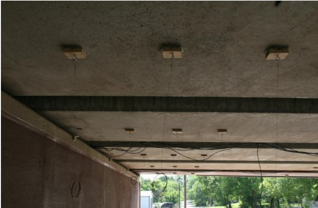
(b) LVDT and String Potentiometer Setup Installation
