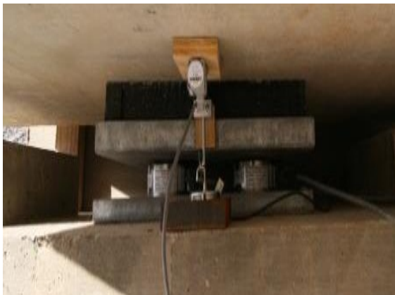
(a) Load Cells and LVDT
