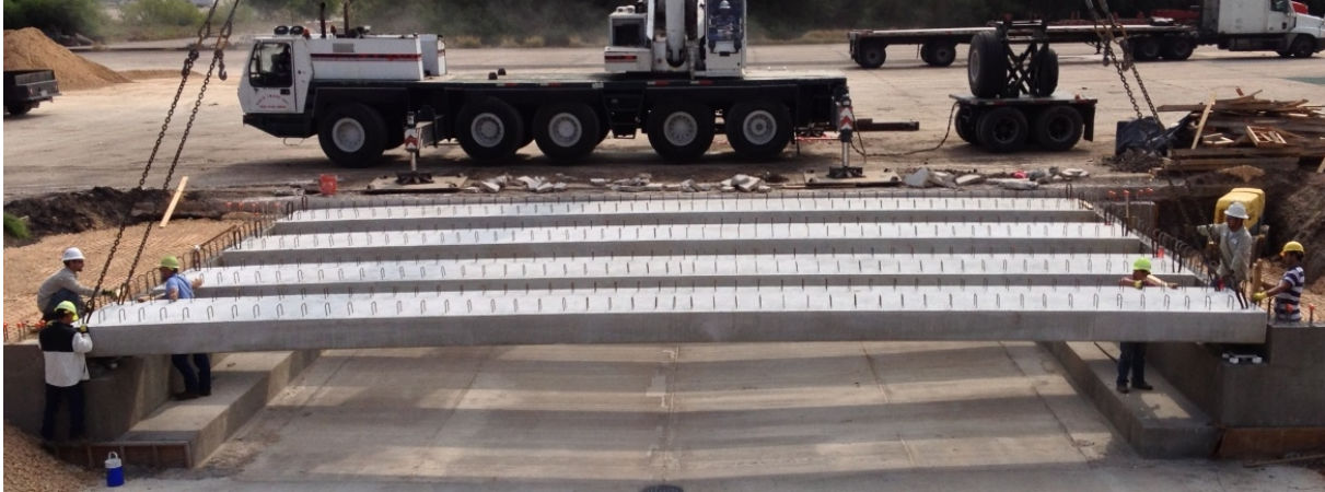
(a) Slab Beam Erection Operation
