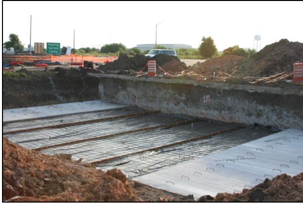
(a) Formwork and Reinforcement
