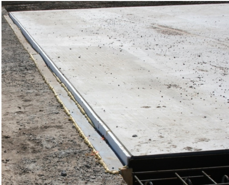
(a) Expansion Joint and Steel Sheet Form.
