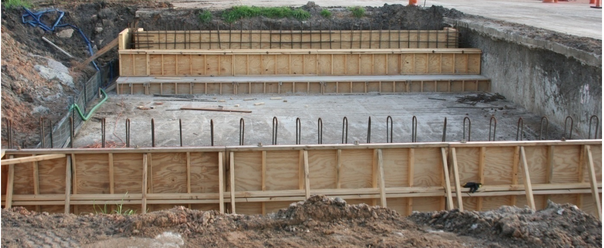
(c) Abutment and Wing-Wall Formwork Construction
