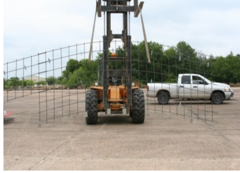
(b) Rebar Mesh Installation
