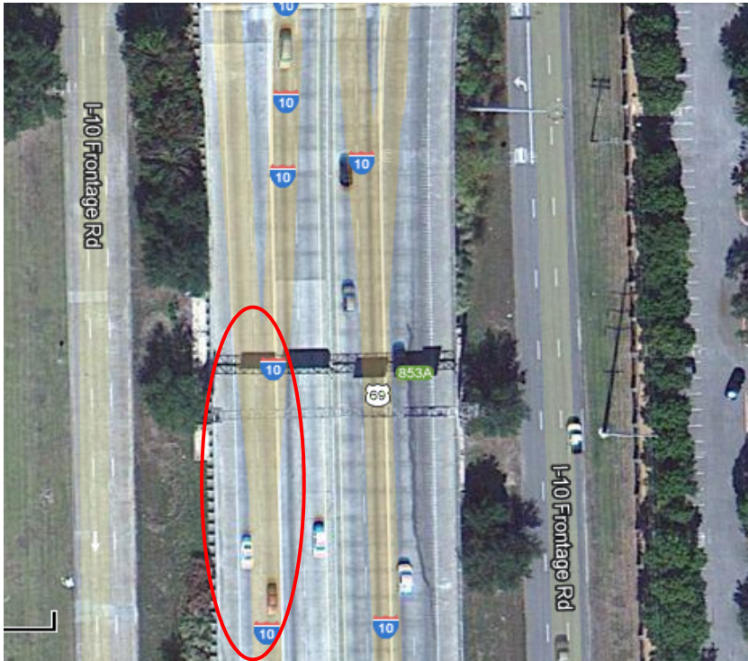
(b) Distressed Portion of the Roadway.
