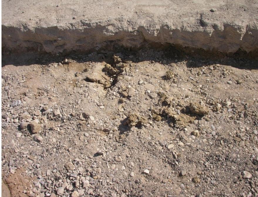
Figure 28. Clay Layer underneath BAS.
