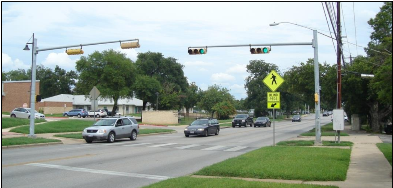
Figure 6. Example of Traffic Control Signal Installation.
