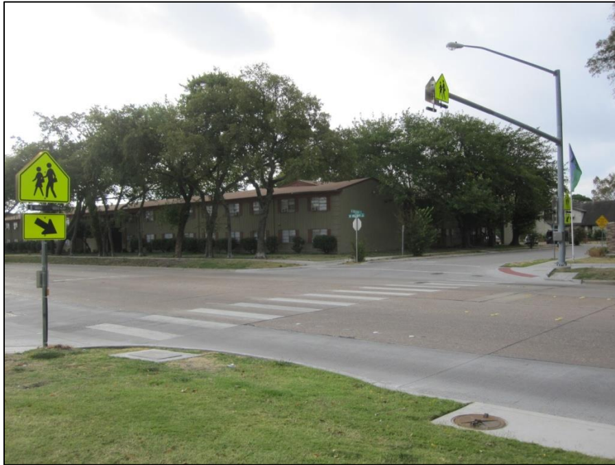
Figure 4. School Crosswalk with RRFBs in Garland, Texas (73).
