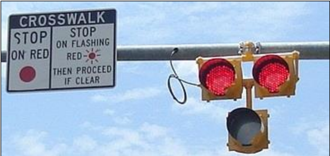
Figure 8. Example of a Sign Used with a Pedestrian Hybrid Beacon Installation.
