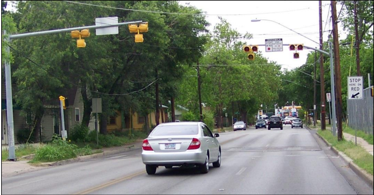
Figure 7. Example of Pedestrian Hybrid Beacon Installation.
