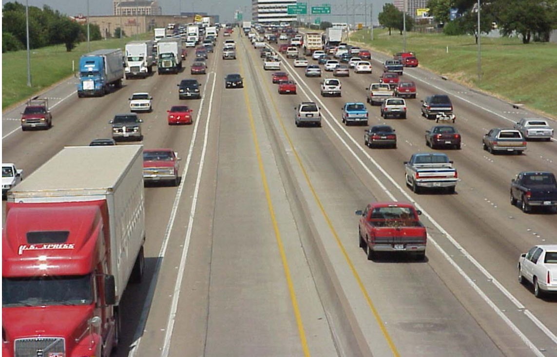
Figure 75. Example of Buffer-Separated HOV Lane Facility.
