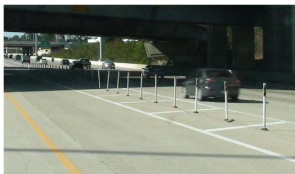
Figure 37. Pavement-Mounted Pylon.
