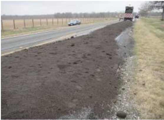
c) Placement of Material
