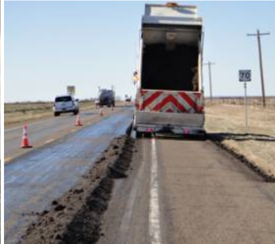
b) Placing Material
