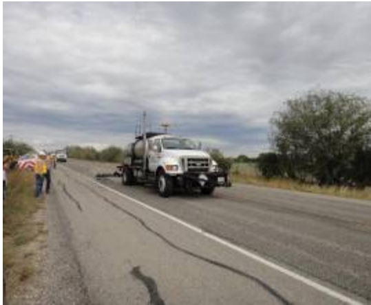
a) Application of Tack
