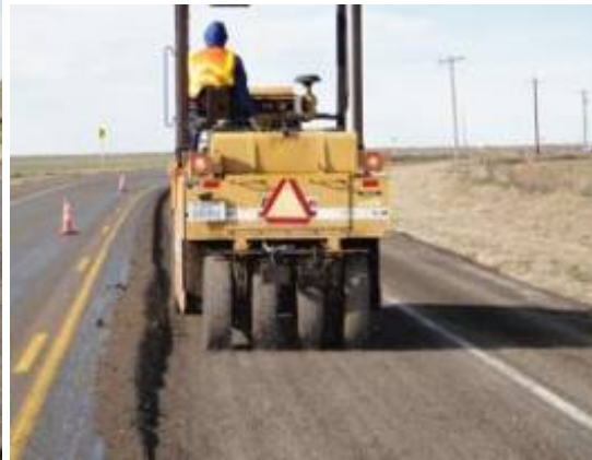
d) Compacting in Multiple Lifts
