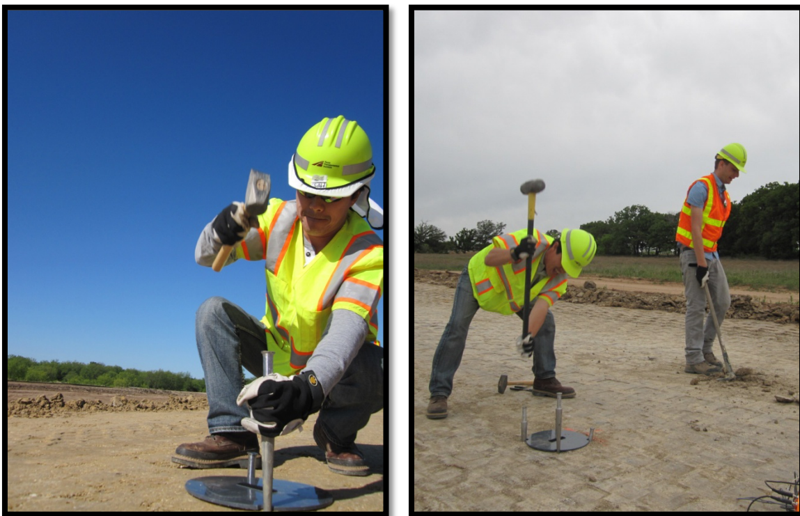
Figure 11. Preparing for EDG Tests and Collecting Soil Samples on US 67.
