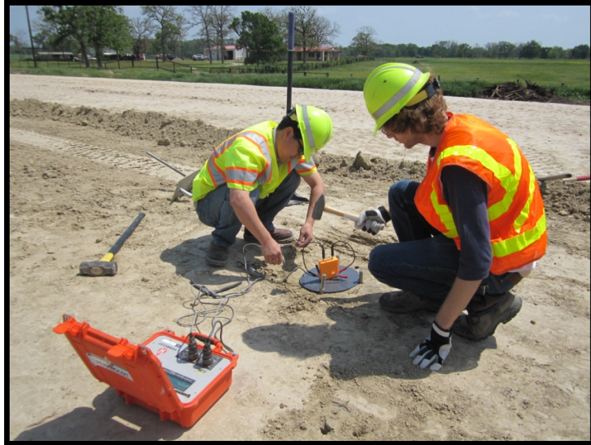
Figure 6. Preparing EDG Test on SH 21.
