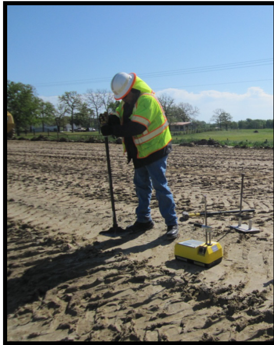
Figure 8. Preparing Test Area at High Water Content Zone on SH 21.
