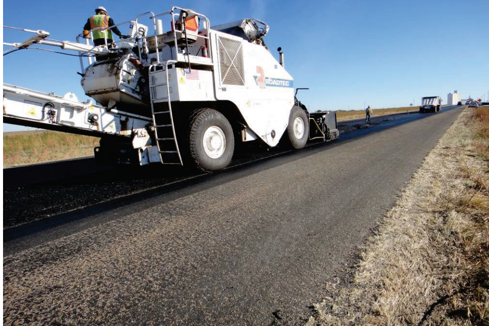
a. Roadtec Shuttle Buggy Vehicle Transferring Material.
