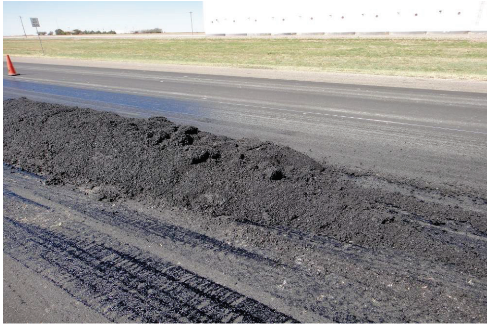
a. Big Lumps in the Asphalt Mix.
