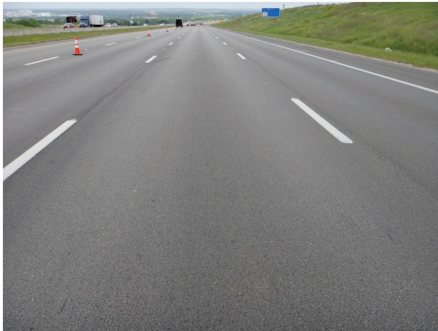
Figure 3-14. Overview of Loop 820 Test Sections Right after Construction.
