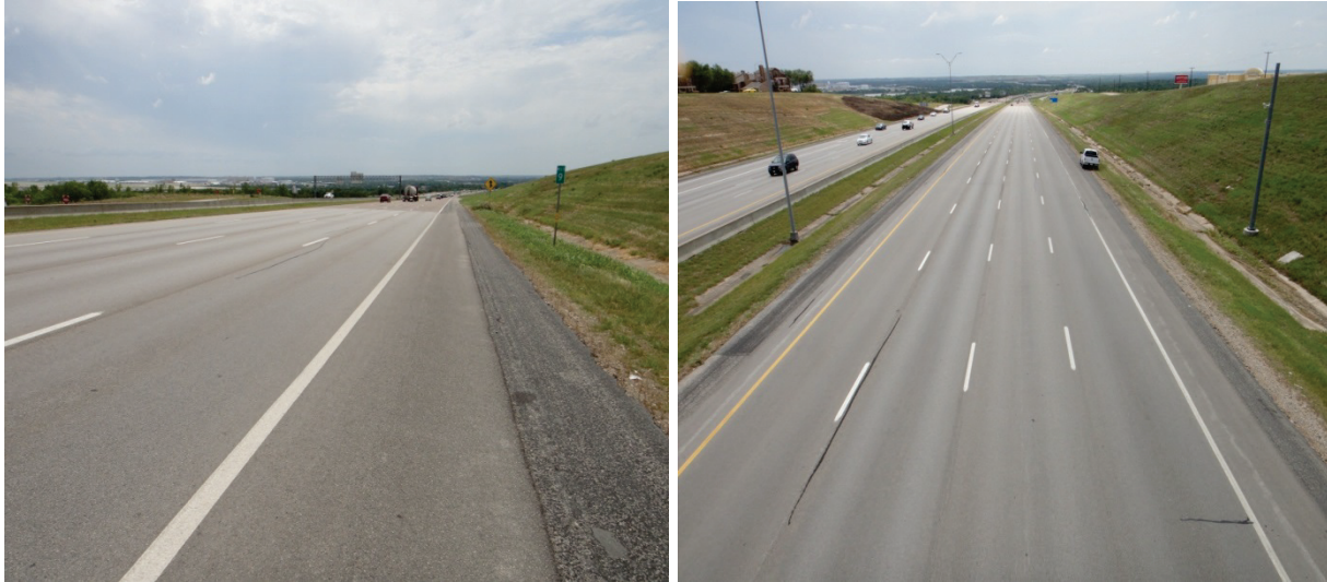
Figure 3-20. Field Survey of US 62 Test Sections.
