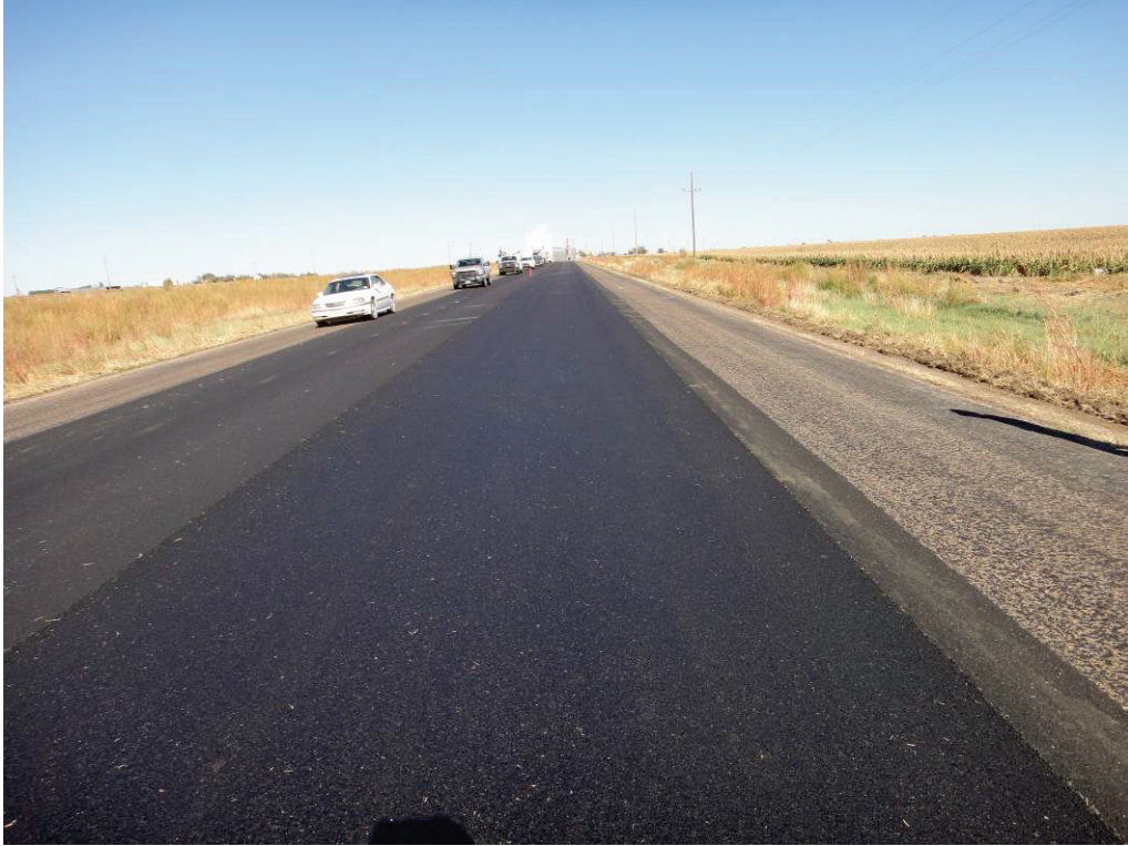
Figure 3-3. Overview of SH 15 Test Sections Right after Construction.
