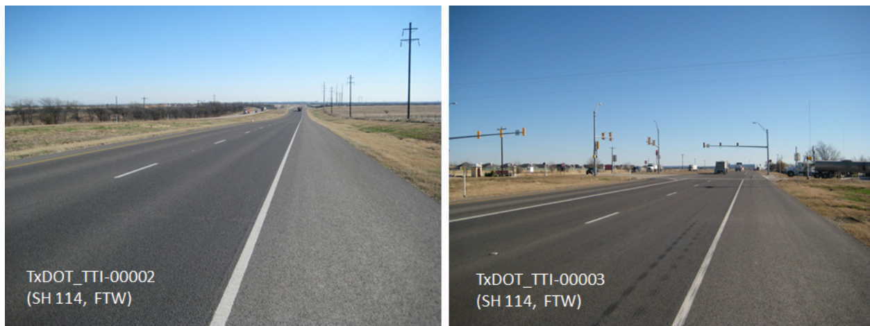
Figure 4-13. TxDOT_TTI-00002 and TxDOT_TTI-00003 after 8 Years of Service (No Visual Distresses).
