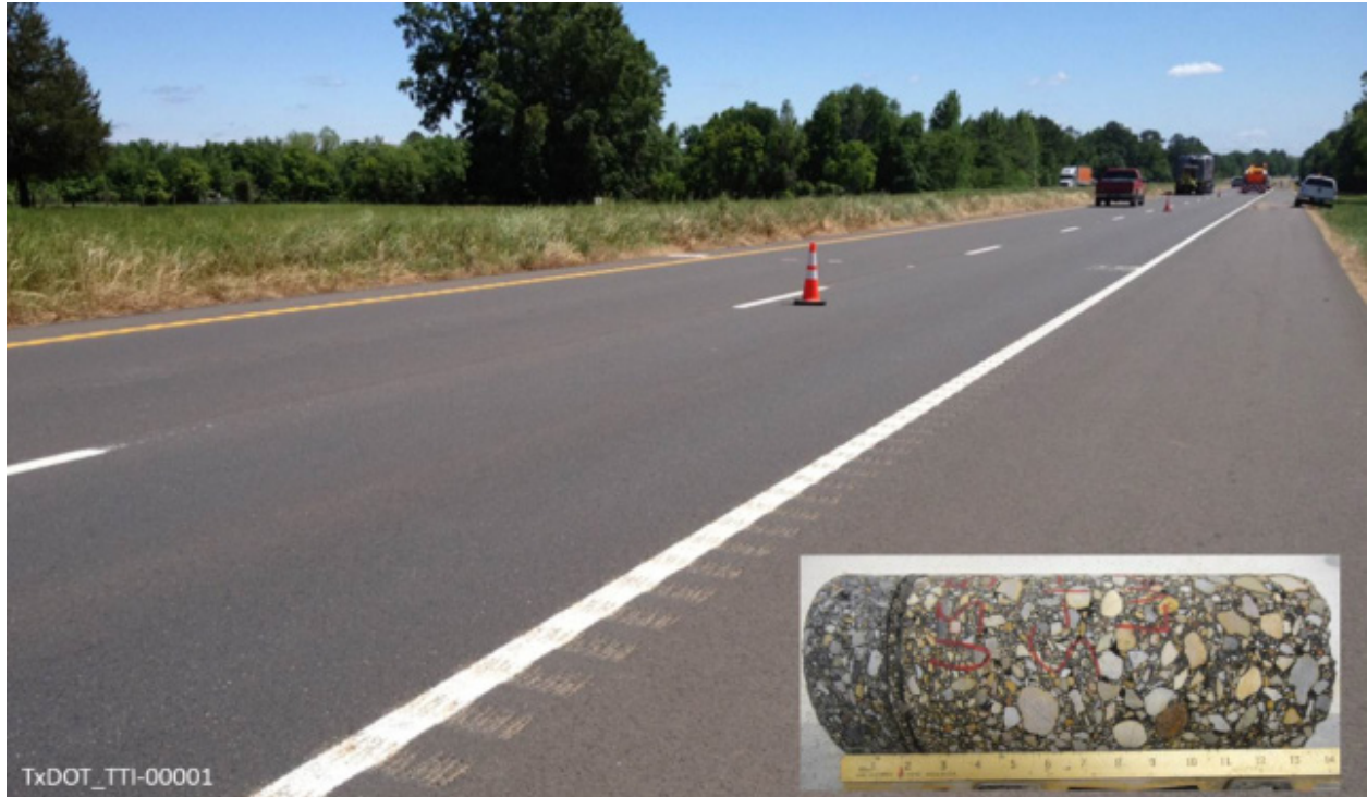
Figure 5-17. TxDOT_TTI-00001 (US 59, ATL) after 21 Months of Service (No Visual Distresses).
