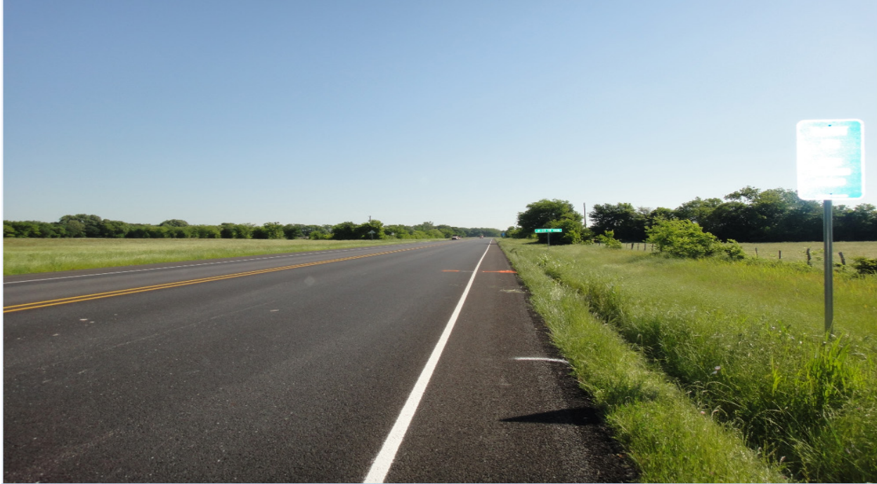
Figure 5-21. TxDOT_TTI-00006 (SH 121, PAR) after 14 Months of Service (No Visual Distresses).
