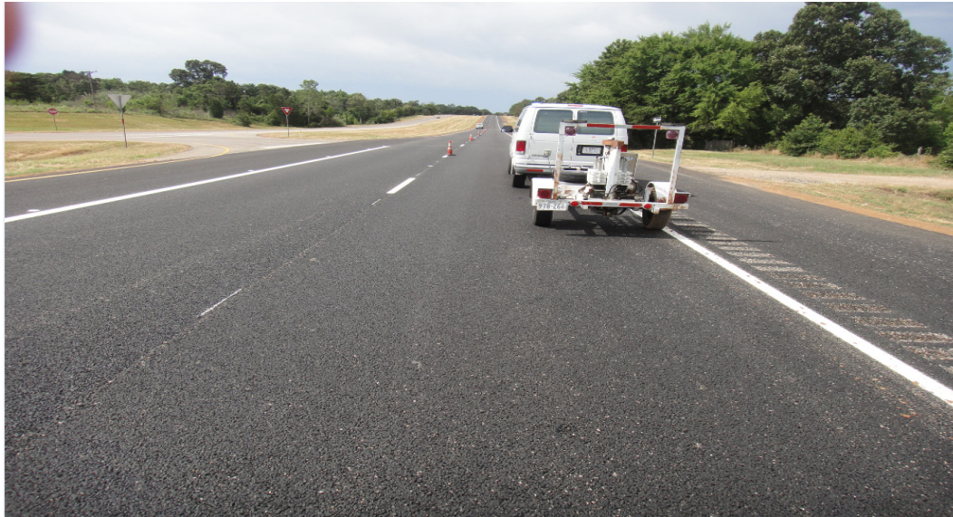
Figure 5-19. TxDOT_TTI-00007 (US 271, PAR) after 13 Months of Service (No Visual Distresses).
