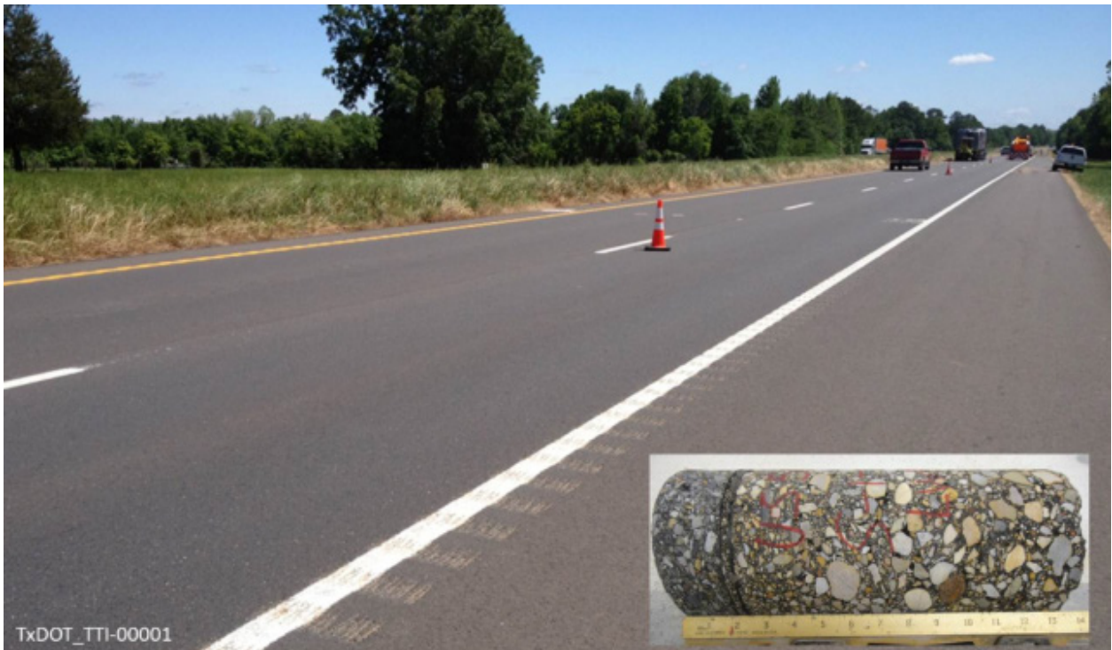
Figure 7-11. TxDOT_TTI-0001 (US 59, ATL) after 21 Months of Service (No Visual Distresses).
