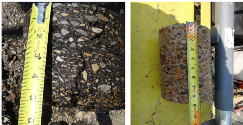
Figure 7-5. Cores from US 271 (Paris District) Prior to Overlay.
