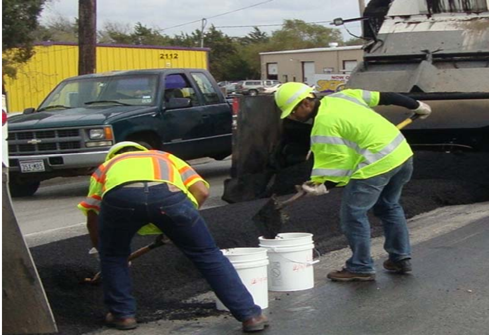
Figure 2-1. Plant-Mix Sampling from the Construction Site.
