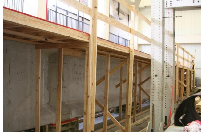
(b) North Side Formwork
