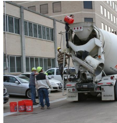
(c) Adding Admixture and Water to Truck
