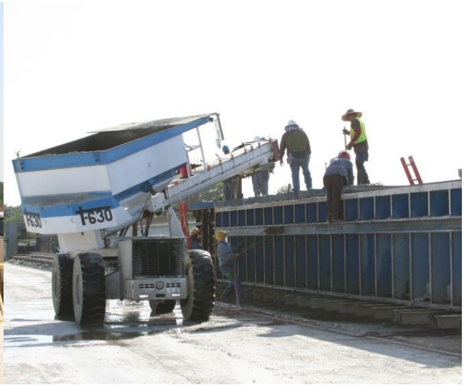
(b) Casting Concrete Transported from Batch Plant
