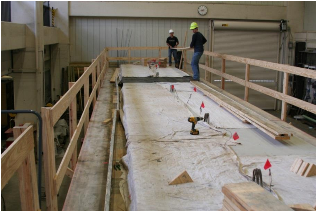
(c) Curing the Deck and Removing the Deck Formwork
