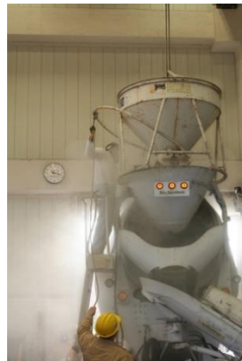
(b) Adding cement to truck
