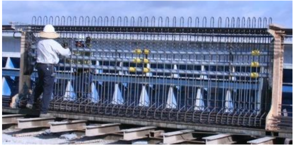
(a) Installing Reinforcement
