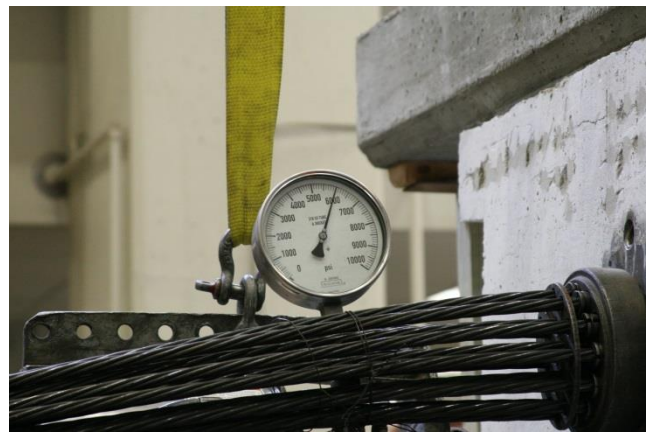
(c) Measuring Pressure during Stressing
