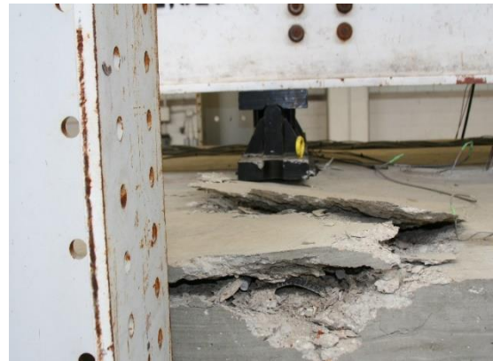
(c) Compression Failure at P = 400 kips
