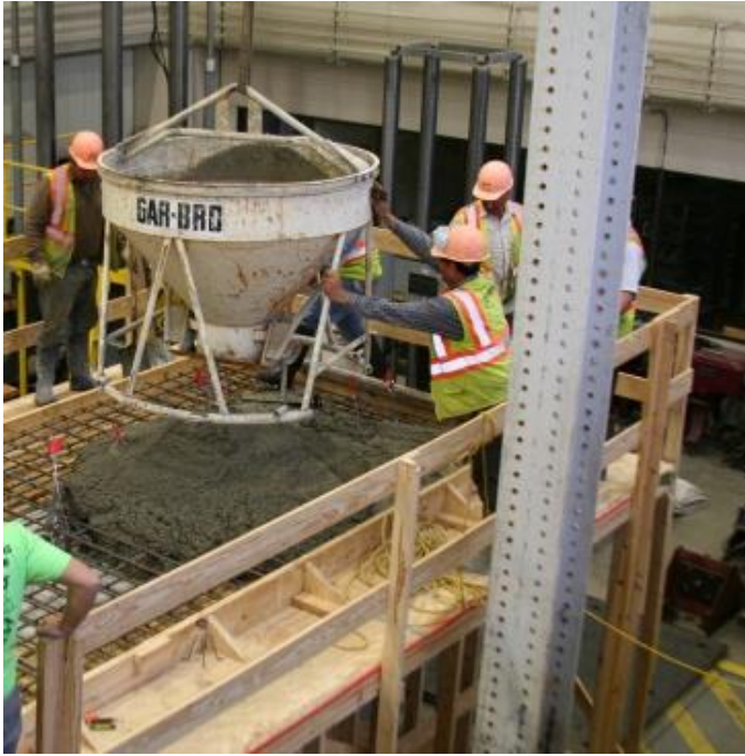
(a) Casting the Deck
