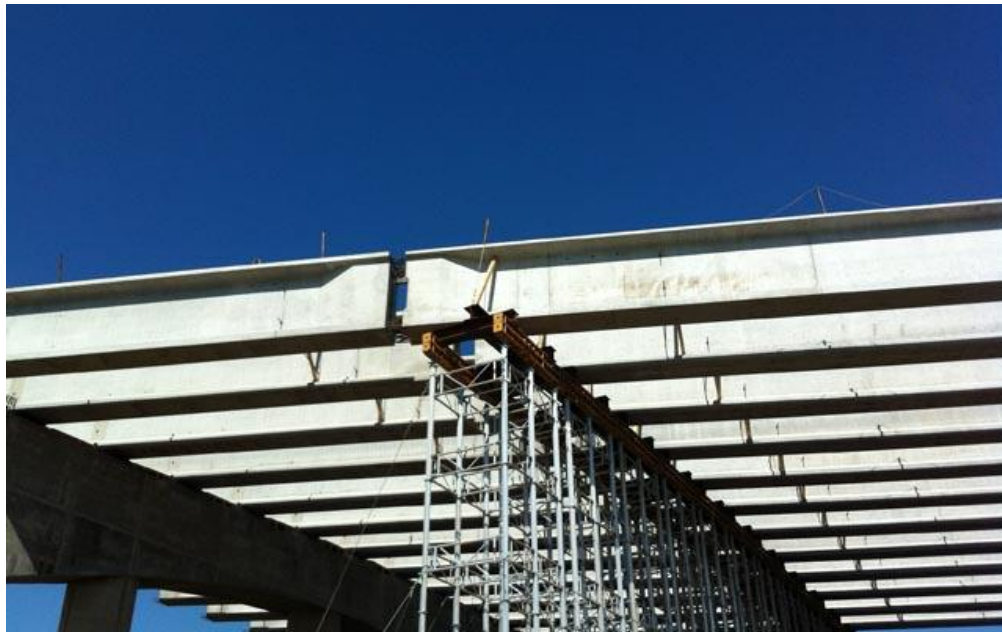
(b) Shore Towers on Both Spans
