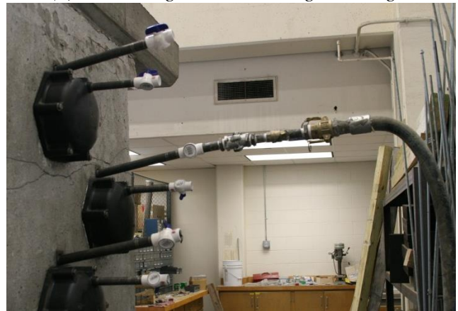
(e) Grouting Ducts Using Air Pressure
