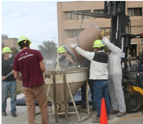
(a) Measuring Cement into Hopper
