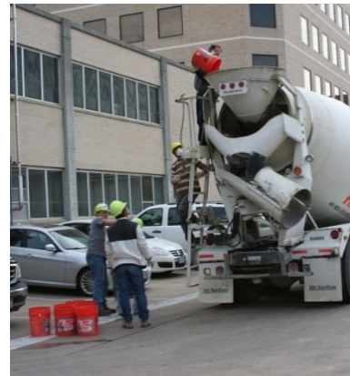
(c) Adding admixture-water mix to truck
