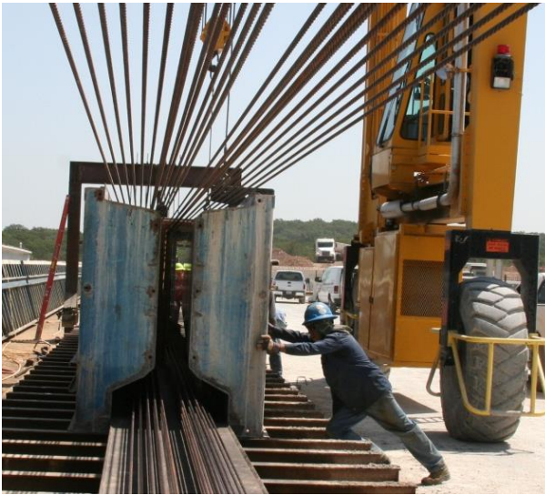
(a) Installing Formwork
