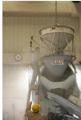
(b) Adding Cement to Truck
