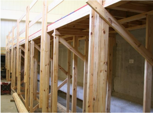
(a) South Side Formwork
