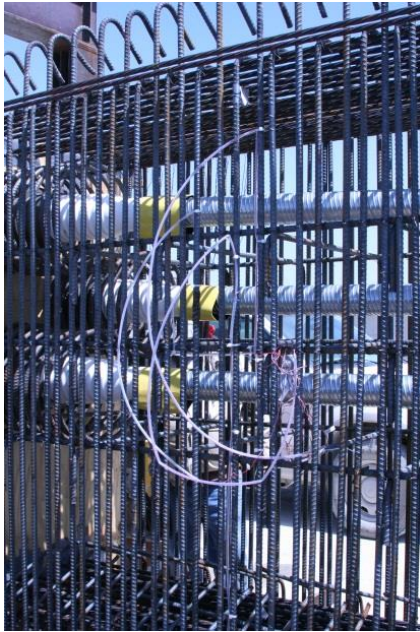
(c) Protecting Gage Wires
