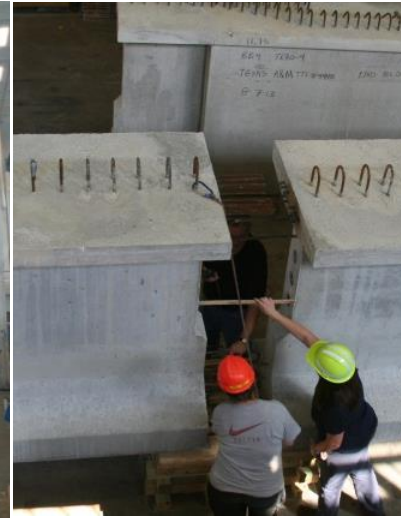
(c) Verifying Segment Spacing and Placement
