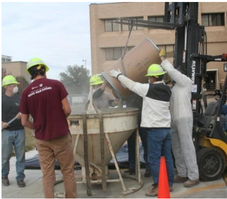
(a) Measuring cement into hopper
