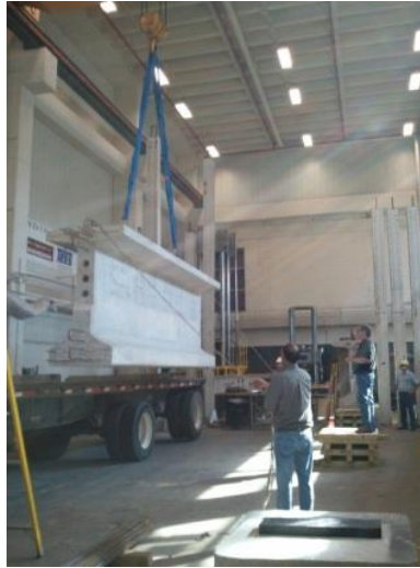
(b) Placing Girder Segments
