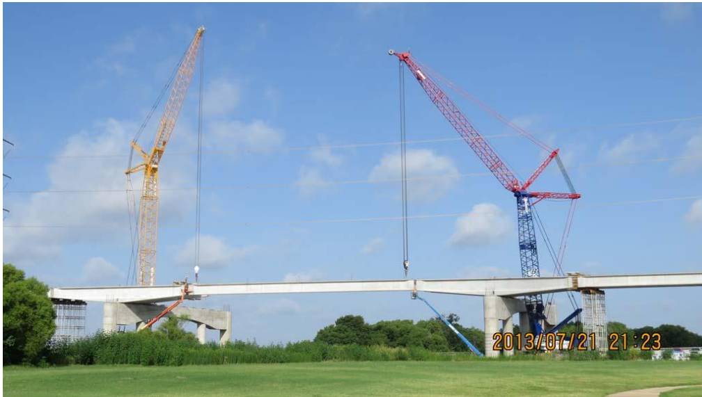
(a) Placing the Drop-in Segment within Span 11
