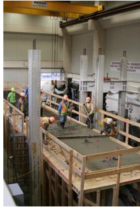
(b) Finishing the Deck
