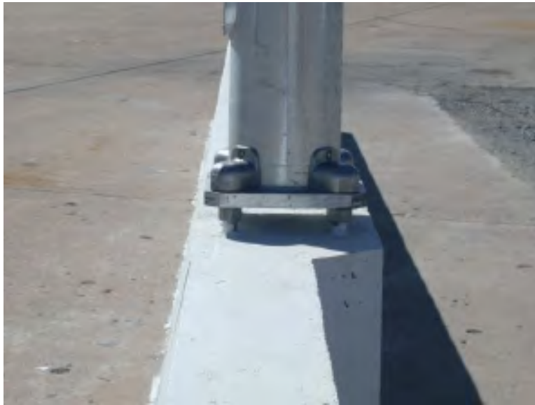
Figure 2.9. Luminaire Pole Attached to Single Slope Barrier for MwRSF Tests: ZOI-1 and ZOI-2 (12).
