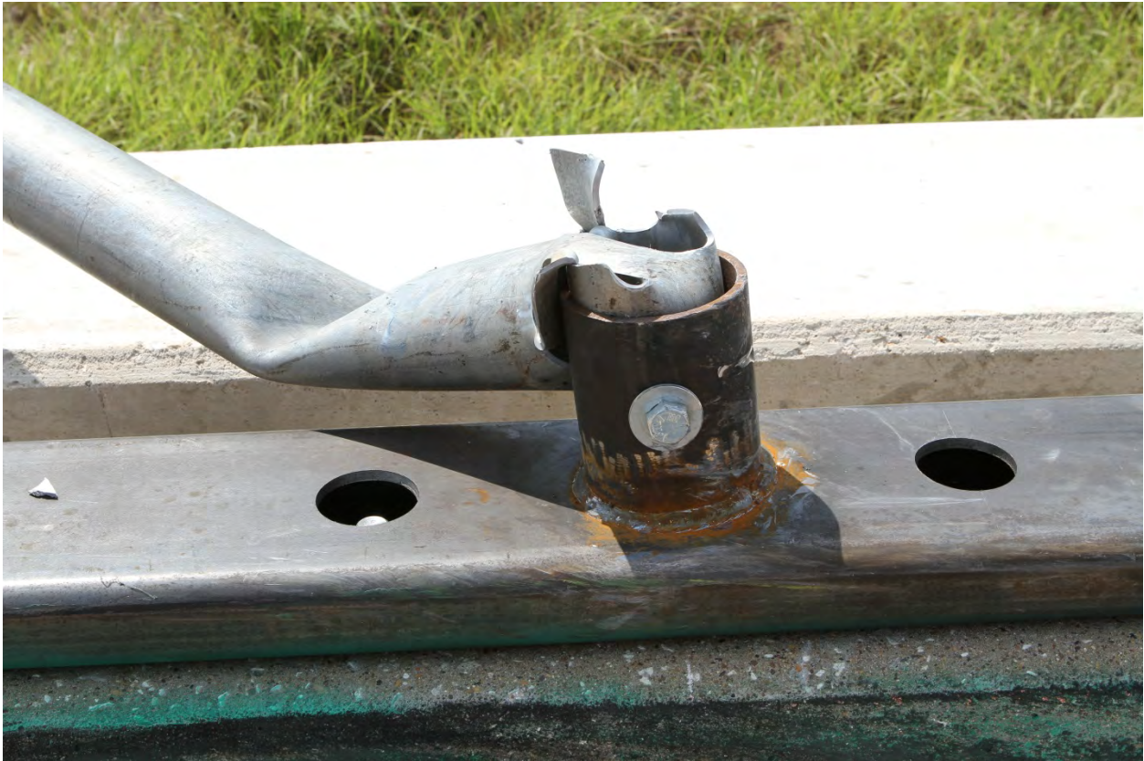
Figure 6.36. Slotted 10 BWG Sign Support on CMB after Test No. 466462-4.
