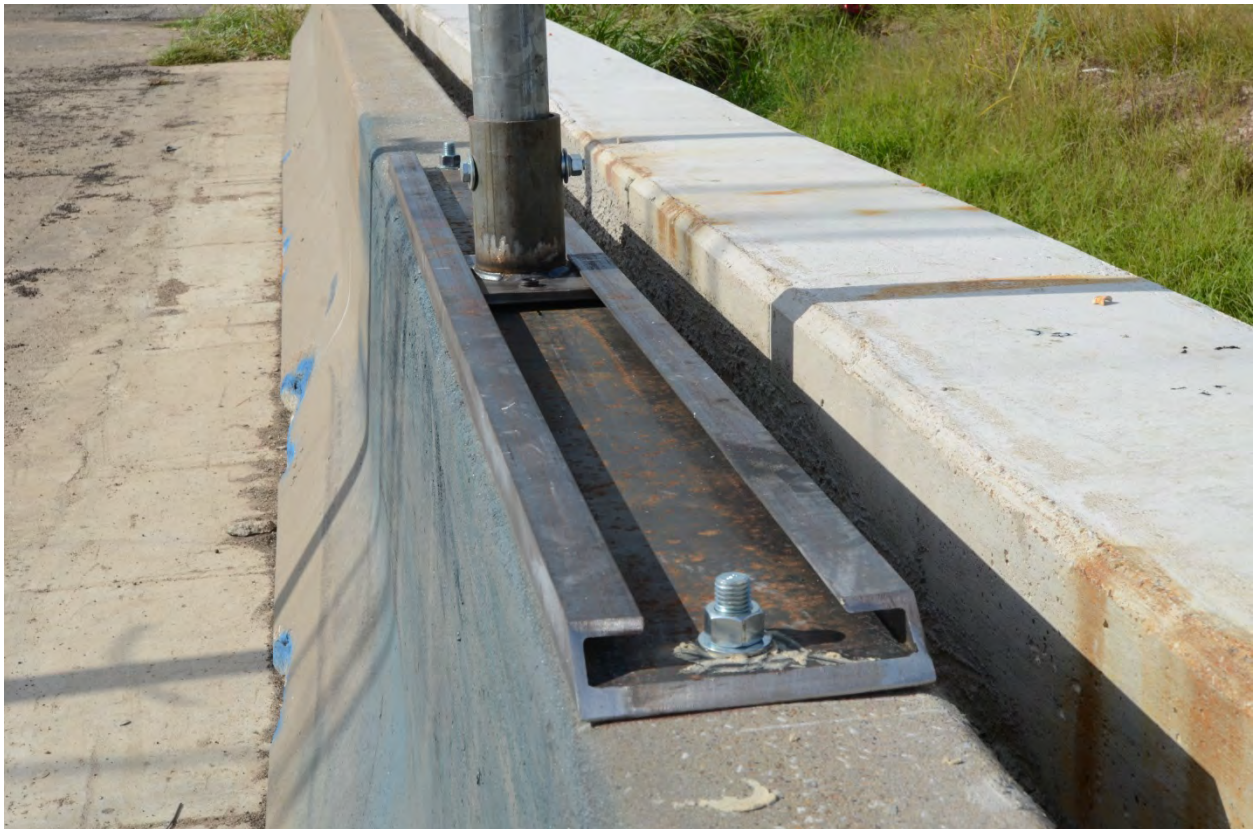
Figure 6.23. Chute Channel Sign Support on CMB before Test No. 466462-3.
