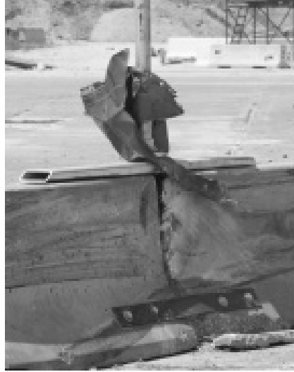
Figure 2.8. Sign Support Connection after the Crash Test (11).
