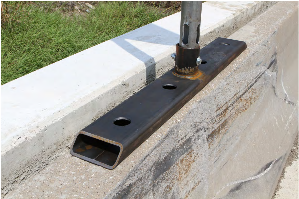
Figure 6.32. Slotted 10 BWG Sign Support on CMB before Test No. 466462-4.
