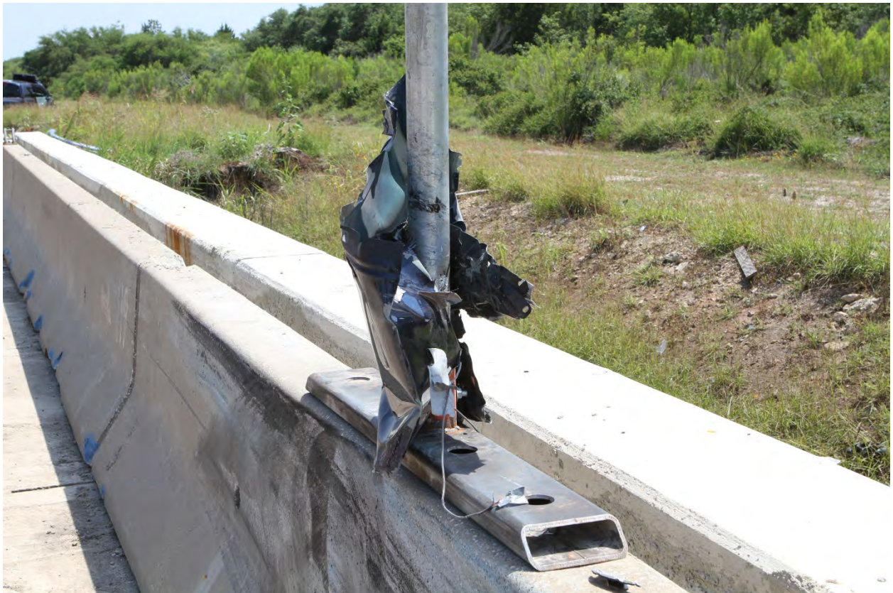
Figure 6.9. Spread Tube Sign Support System on CMB after Test No. 466462-1.
