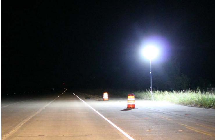
Figure 18. Northbound Approach to Balloon Light.
