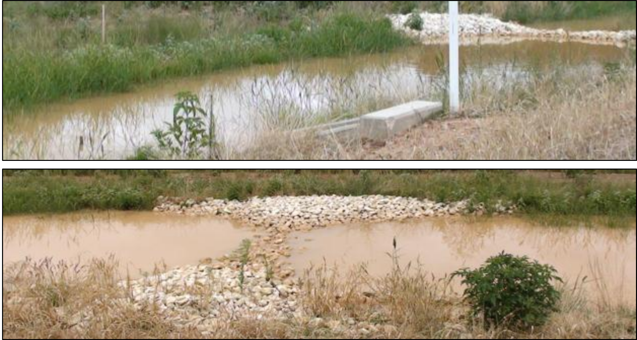
Figure 20. Hearne Project Watershed 1 Swale with Rock Check Dam.
