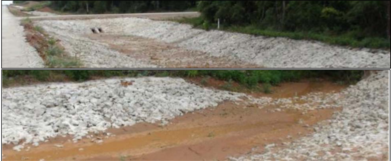
Figure 23. Hearne Project Watershed 4 Swale Covered by Rock Riprap.
