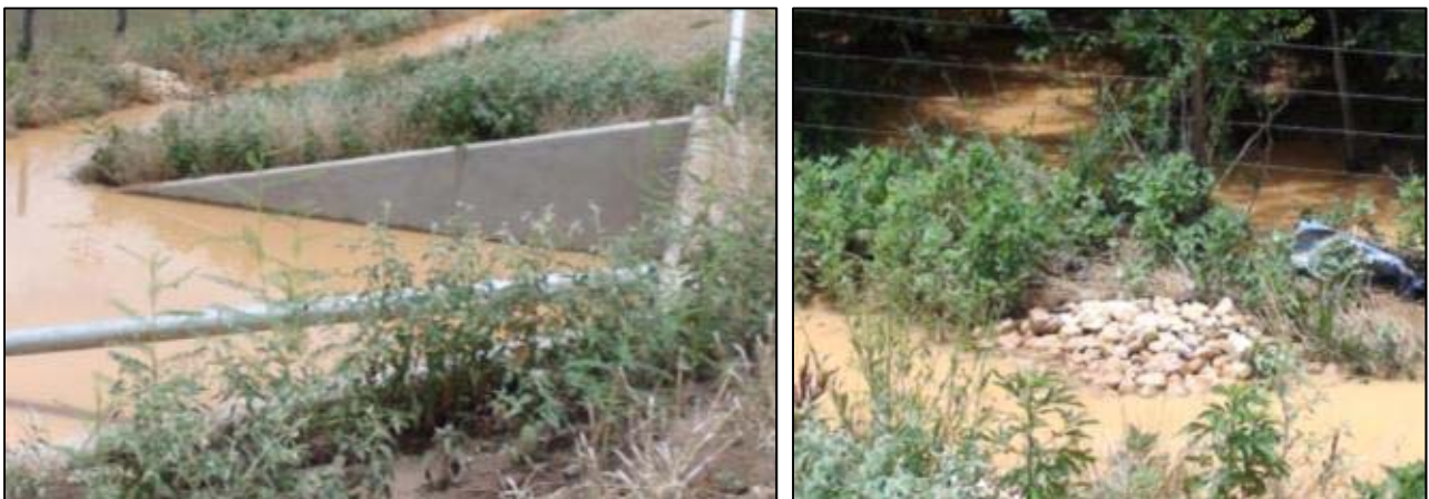
Figure 24. Hearne Project Watershed 5 Swale Used as a Retention Basin.
