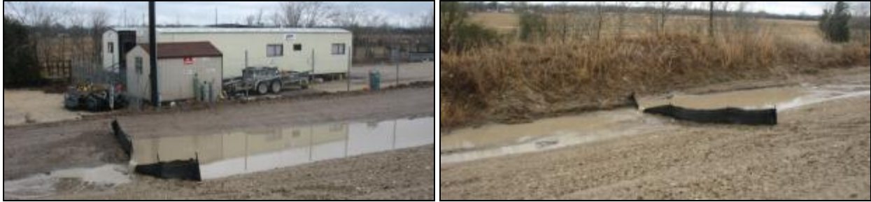
Figure 19. CS Project Watershed 3 Swale with Silt Fence on Bare Soil.
