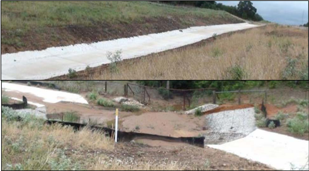
Figure 21. Hearne Project Watershed 2 Concrete-Paved Channel.
