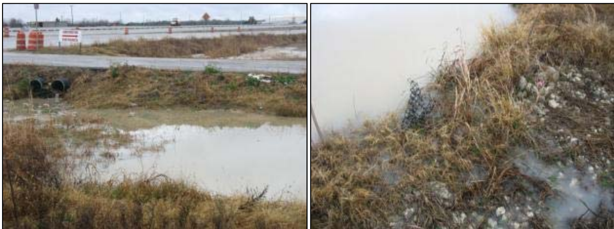
Figure 13. CS Project Watershed 1. Left – Culvert and Detention Basin, Right – Discharge from the Detention Basin.
