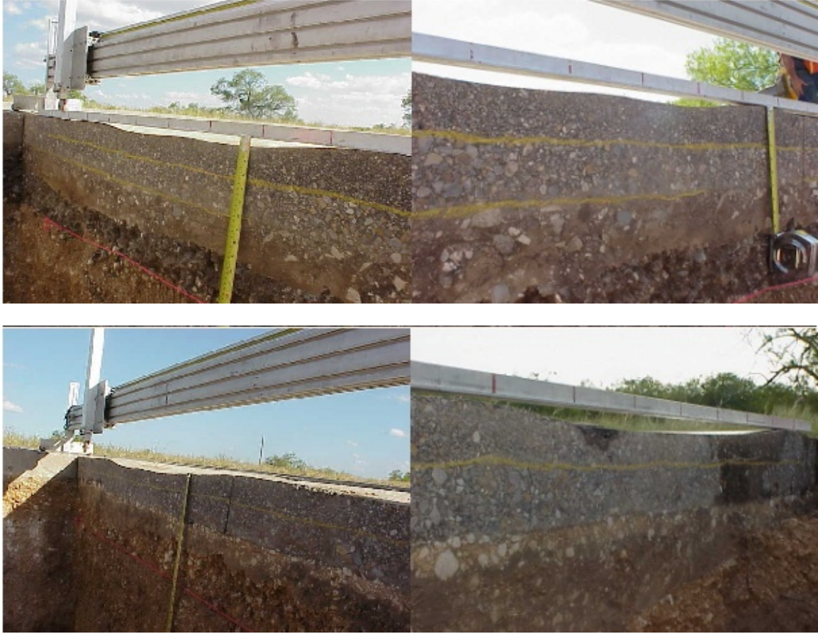
Figure C-13. Trench Profiles for 161 (Top) and 162 (Bottom).
