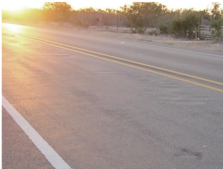
Figure B.12. Subtle Pavement Roughness (Uvalde-CAM).
