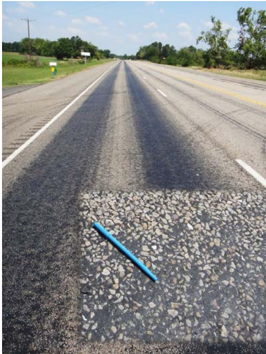
(a) Flushing through the Surface Treatment
