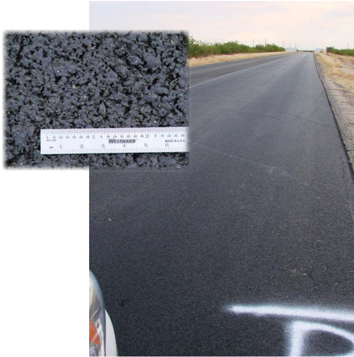
Figure D.5. Hoban-Fine DGM, Entry Road (Pecos RTC).
