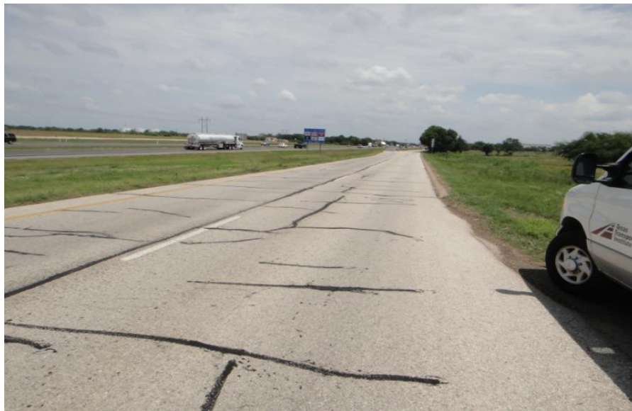
Figure D.20. Existing Pavement Surface (Bryan-Fine SMA).
