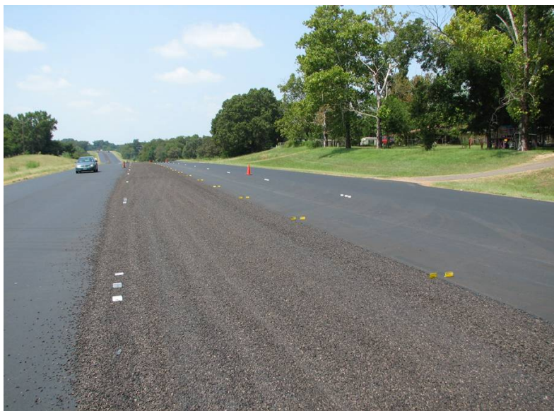
Figure B.15. Surface Treatment on Top of New CAM (Mt. Pleasant-CAM).
