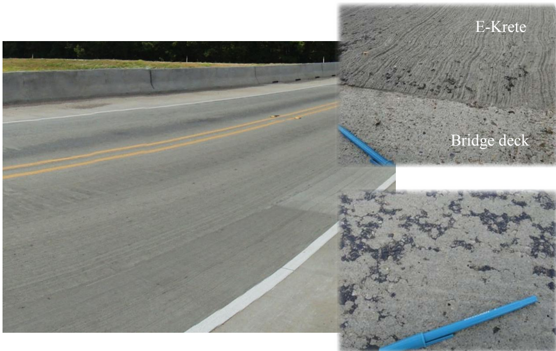
Figure B.43. Project and Surface Texture on Overpass (Atlanta-E-Krete).
