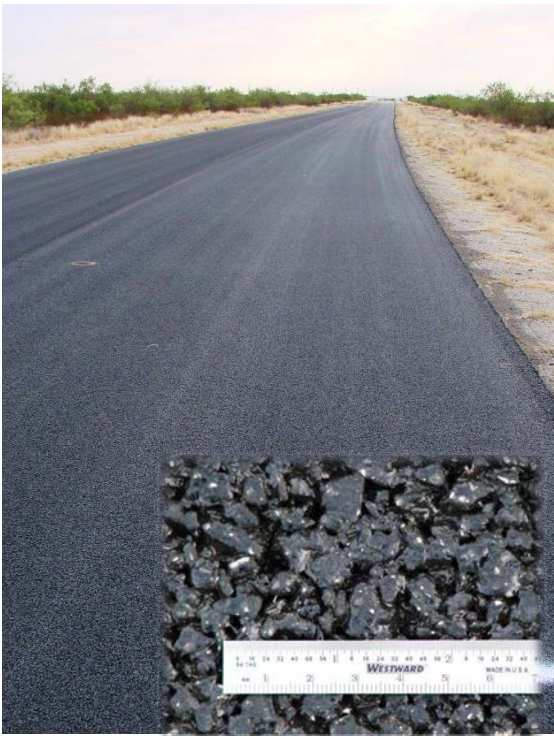
(a) Entry Road
