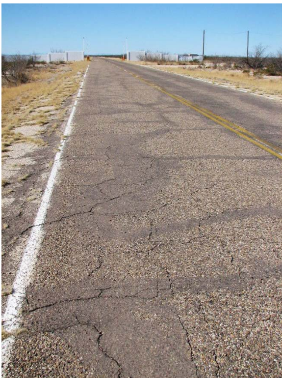
(a) Entry Road
