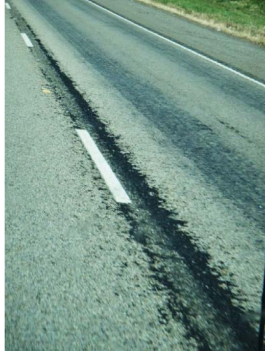
(b) Surface Treatment Construction Joint
