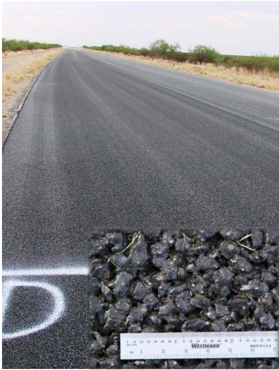
(a) Entry Road
