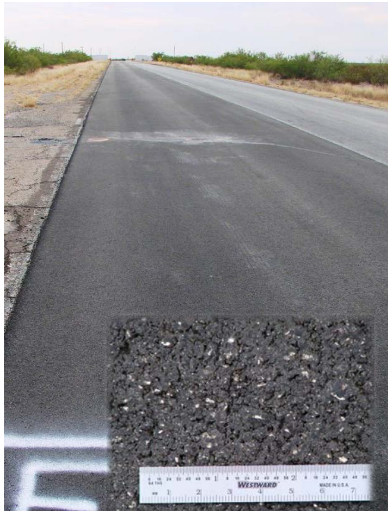
(a) Entry Road
