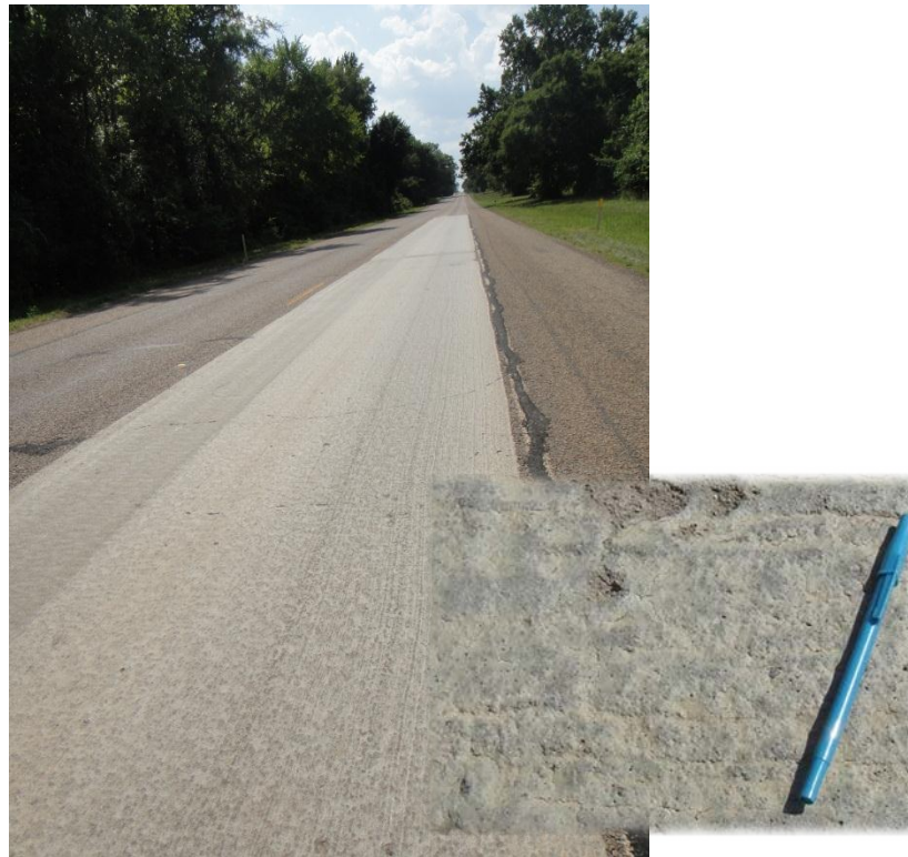
Figure B.41. Project and Surface Texture on US 80 (Atlanta-E-Krete).
