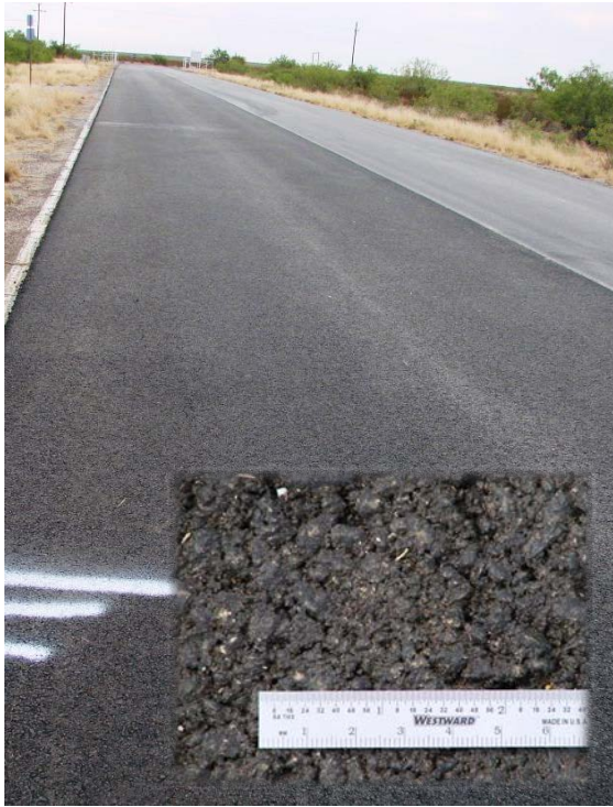
(a) Entry Road
