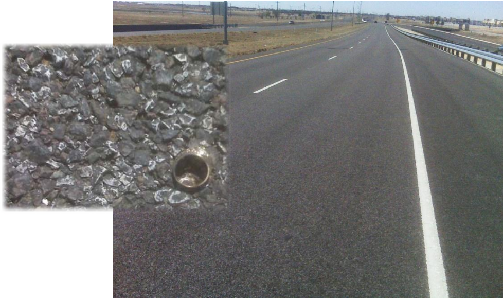
Figure B.31. Project and Surface Texture (Lubbock-NM OGFC).
