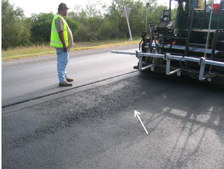
Figure B.10. Low-Density Cold Streak with Potential for Raveling (Uvalde-CAM).
