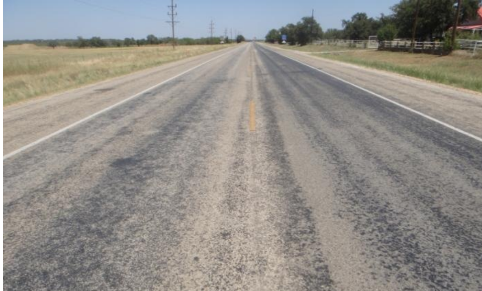
Figure D.29. Flushing Surface Treatment (Brownwood-Fine PFC).
