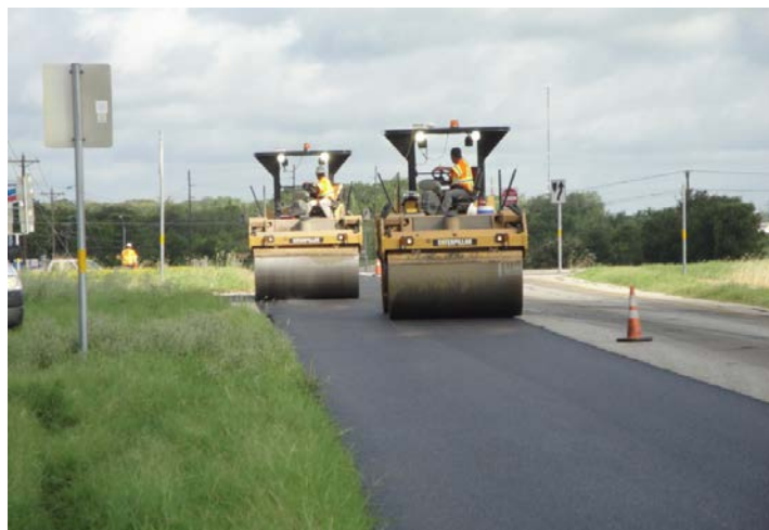
Figure D.21. Tandem Roller Compaction (Bryan-Fine SMA).
