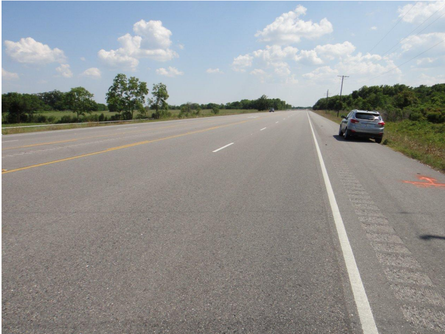
Figure 37. Perfect Condition of RAP/RAS Test Section on SH146, Houston.
