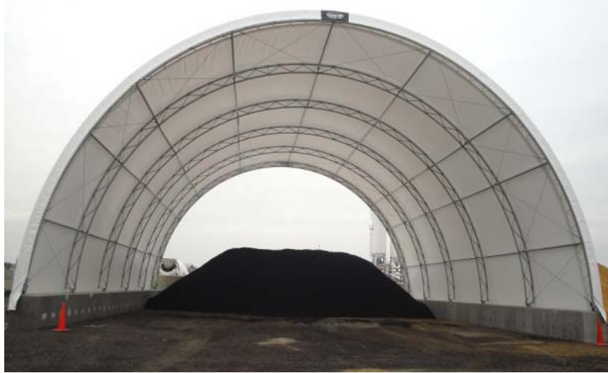
Figure 7. Covered RAS Storing Facility.
