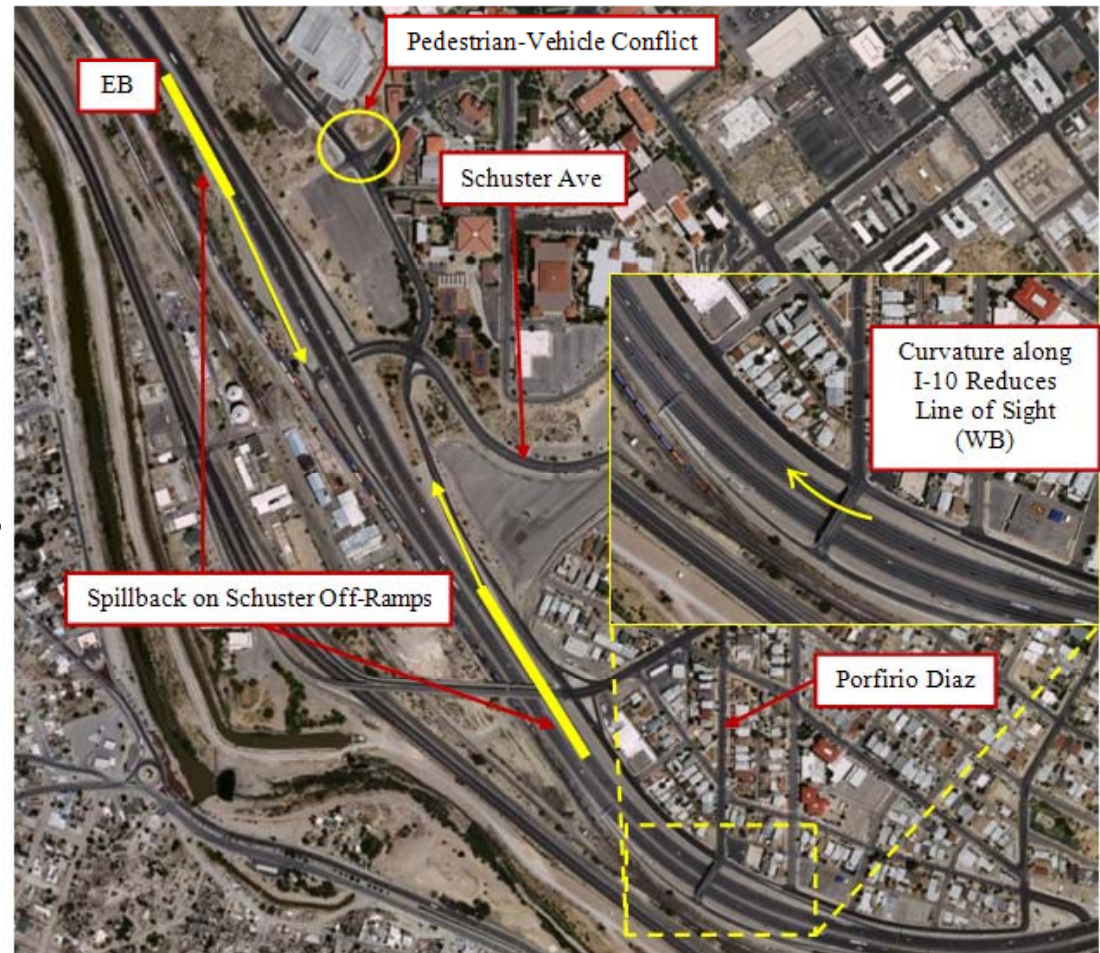
During Morning Peak Hours , there is a Spillback on both Schuster Off-Ramps
