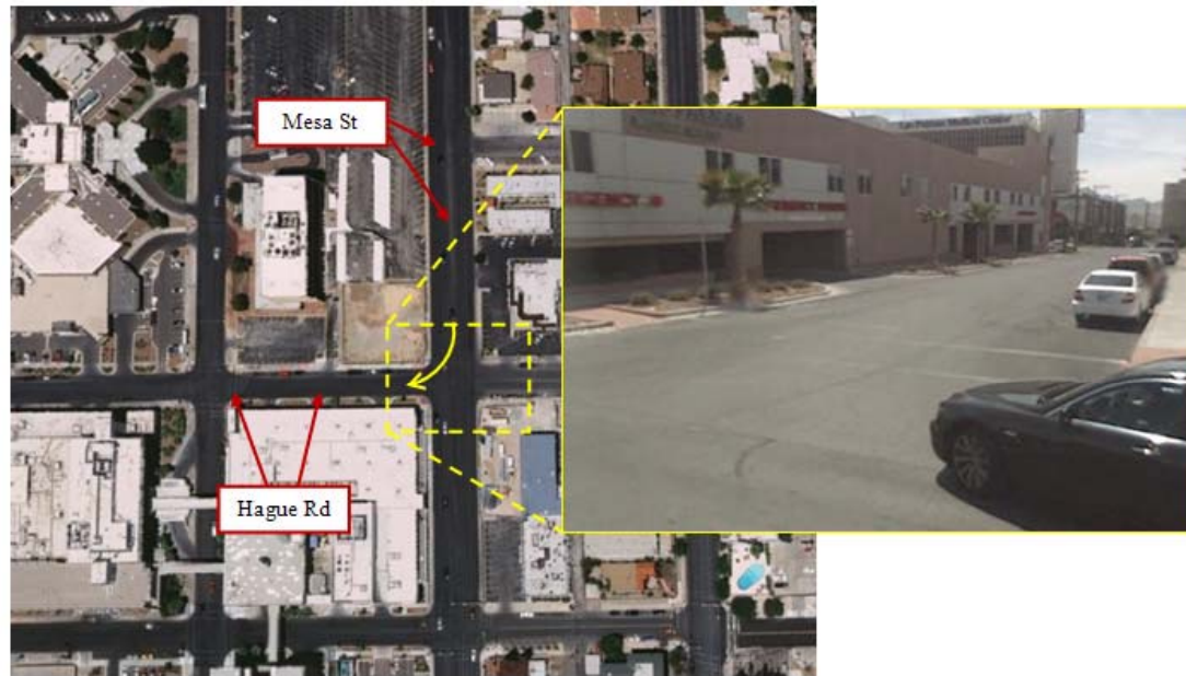
The Crossing Striping on Hague Rd. near Mesa St. is Barely Visible to Drivers
