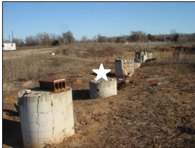
Figure 12-21. Five Straight Shaft Foundations at the NGES.
