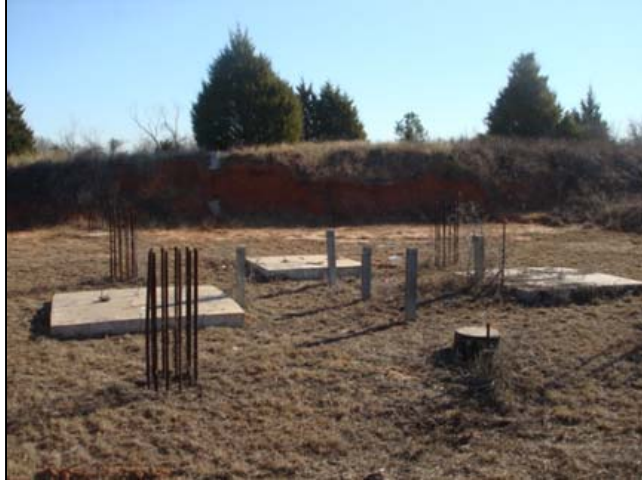
Figure 12-3. Large Footings at the Sand Site.
