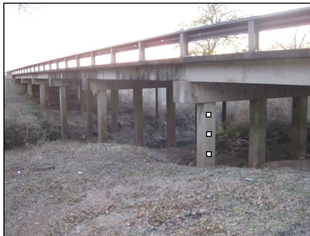
Figure 9-4. Accelerometers on Kountze Bayou Bridge.
