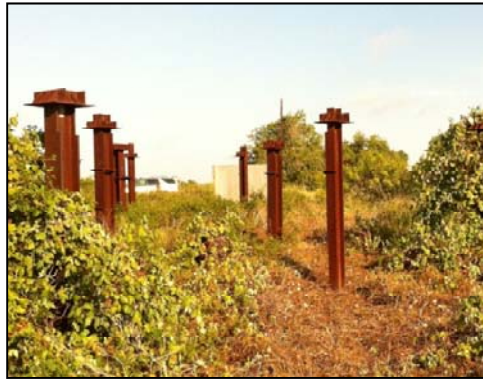
Figure 12-25. H-Piles at the NGES.
