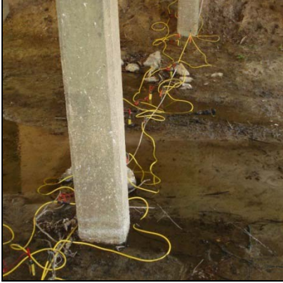
Figure 12-34. Two Piles Tested through Water.
