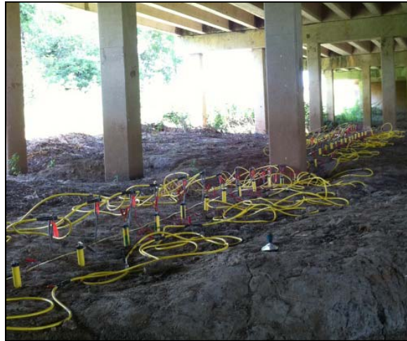
Figure 12-31. Field Setup for Bridge 17-026-0116-03-037.
