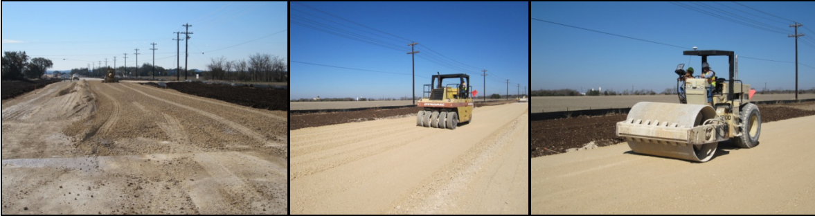
Figure 2.3. Spreading and Compacting Control Strip 1.
