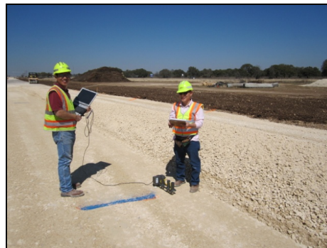
Figure 2.4. PSPA Testing on US 183 Flex Base.
