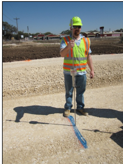
Figure 2.11. DCP Testing on US 183 Flex Base.
