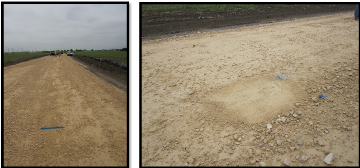
Figure 4.2. Location of Testing on Rose Lane and Site Preparation Required.
